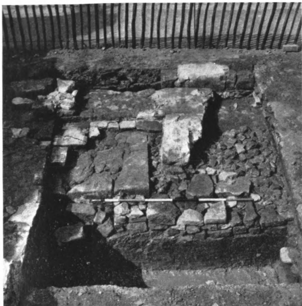
Fig. 1. Trench 1 from the south, before the removal of the footings and jamb of the 17th-c. fireplace
