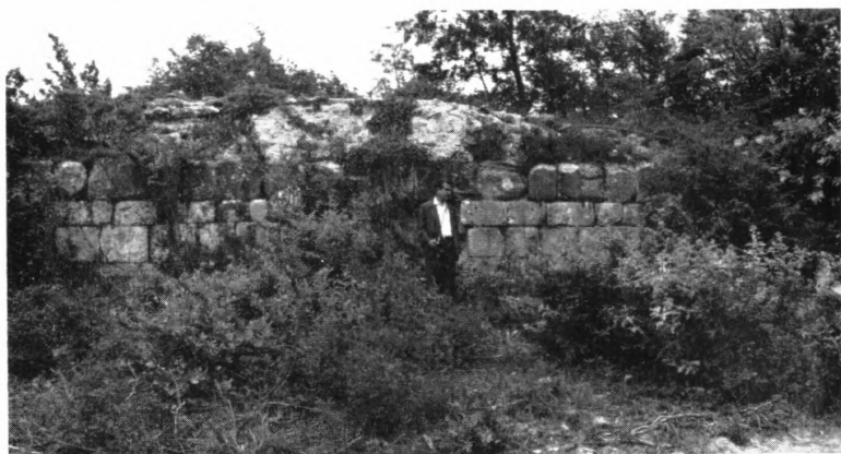
1. Inner face of Wall, about 250 m. south of Derviş Kapı
