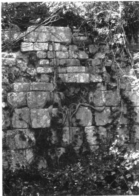
2. Inner face of Wall, about 2 km. north of Derviş Kapı
