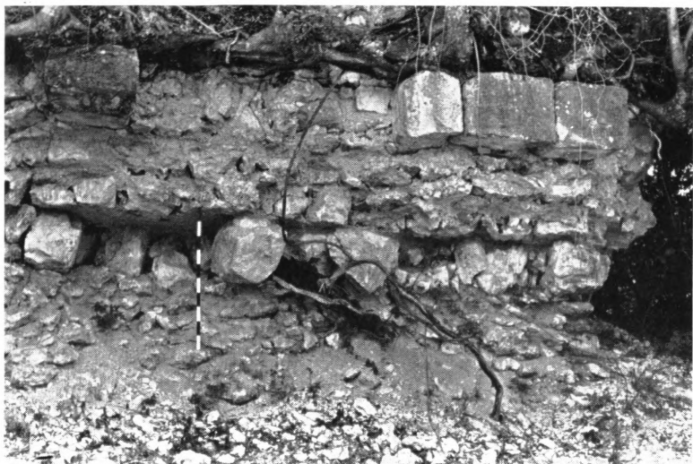
1. Inner face of Wall, about 150 m. south of Derviş Kapı
