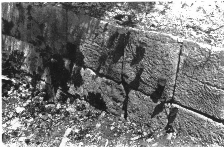
1. Outer face of Wall, about 1 km. north of Derviş Kapı
