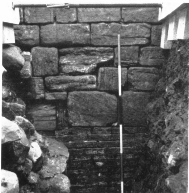
2. The outer face of the town wall above Close Gate
