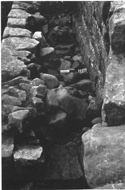
Fig. 2. Narrow curtain wall inset into broad west wing wall, looking westwards.
