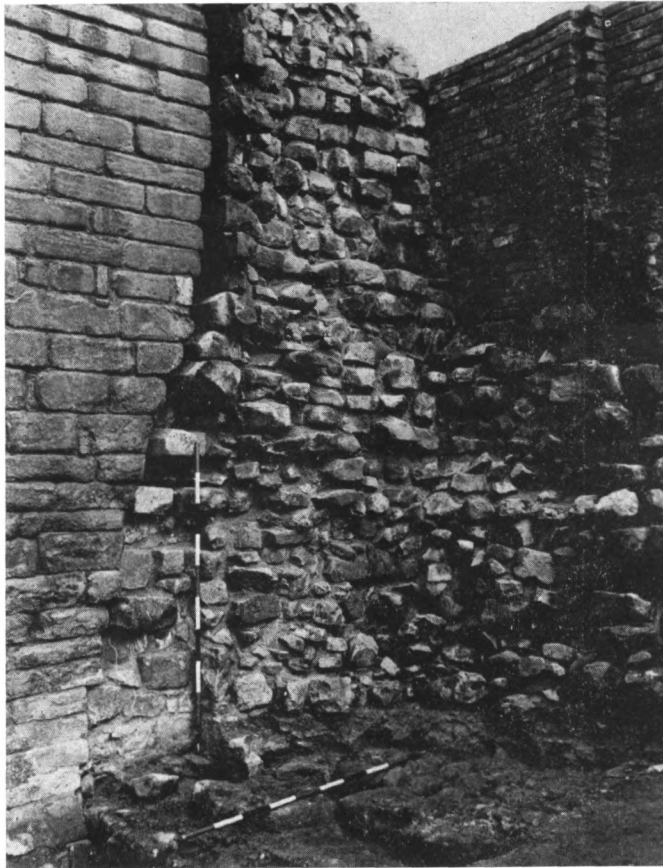
1. The junction of the twelfth- and thirteenth-century curtain walls
