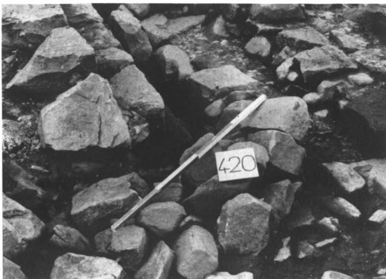
a. Rubble drain (Context 420) through the east face of the Milecastle west wall. Scale: 1 m.
