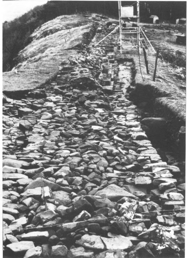
b. The curtain to the east of Milecastle 35; looking East.
