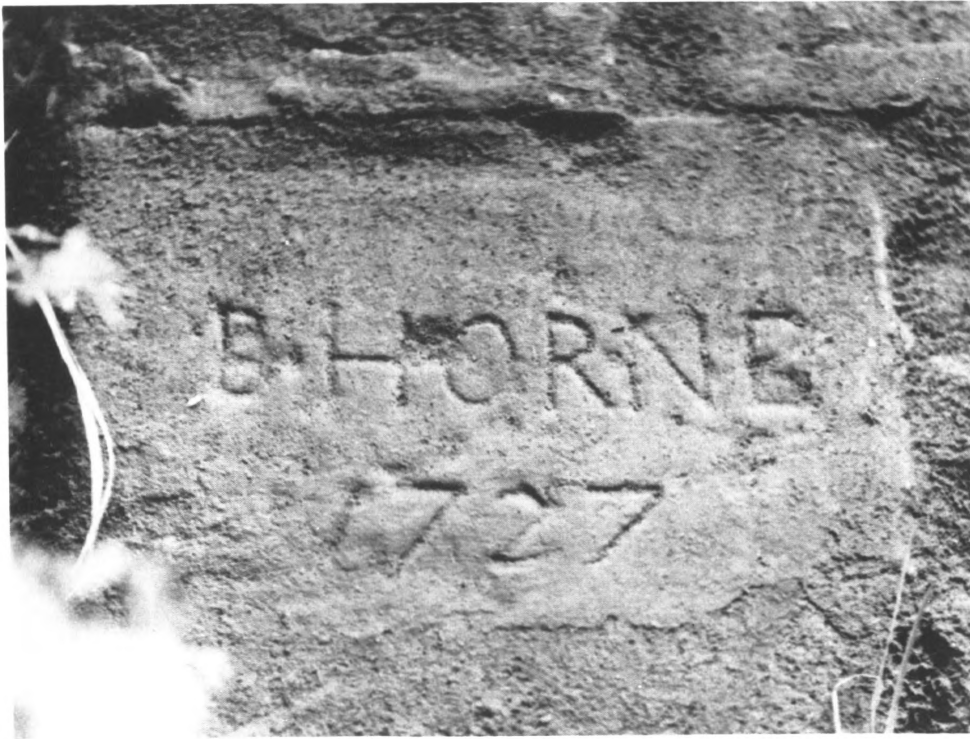
Causey Arch, West abutment: stone at foot of face of abutment.
