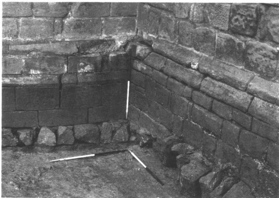
Junction between Morden Tower (left) and Curtain Wall to south (right).
