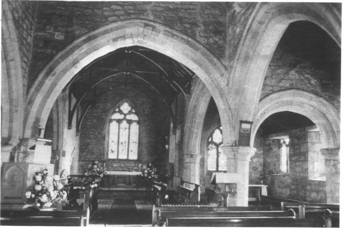
Interior looking east.
