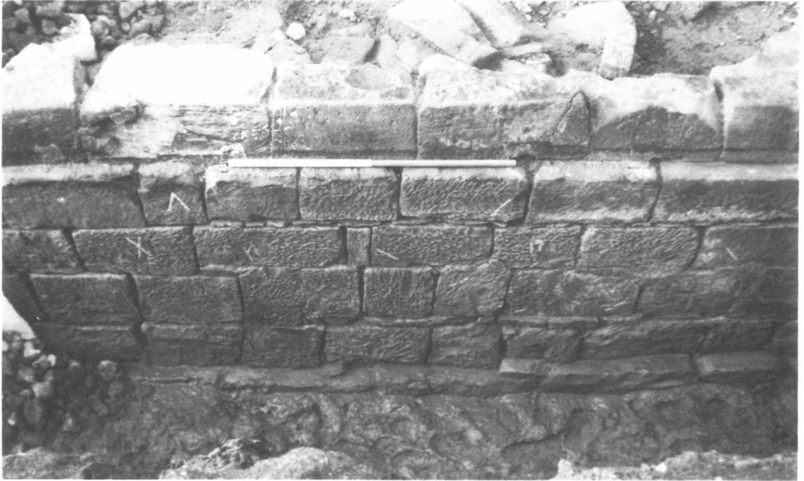
Fig. 10 Wall 42, showing masons' marks.
