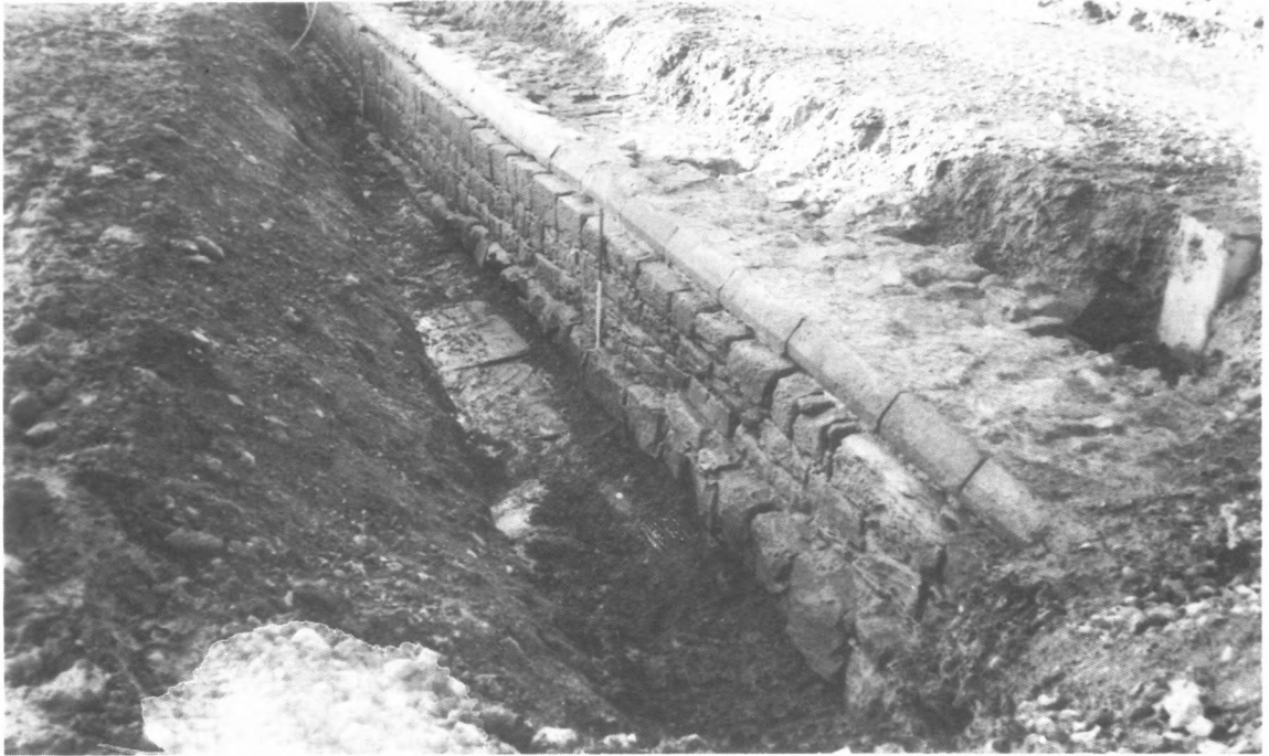
Fig. 8 The Quayside wall, central section.
