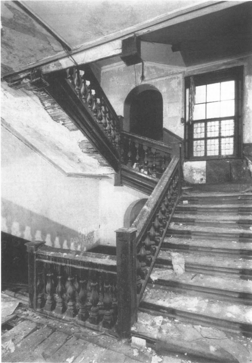
Fig. 7 No. 98. Stair between first and second floors in 1976. (Courtesy of the Royal Commission for Historic Monuments England: NMR B/529, 11.1.1976).
