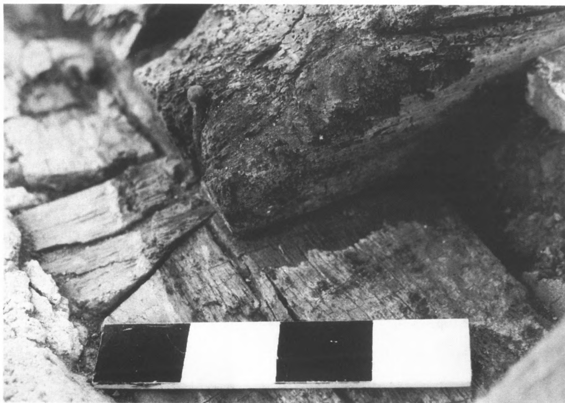
Fig. 14 Truss B, east end of tie beam cut off when boards were laid to raise ends of rafters, now showing remains of dovetail joint onto wall plate.
