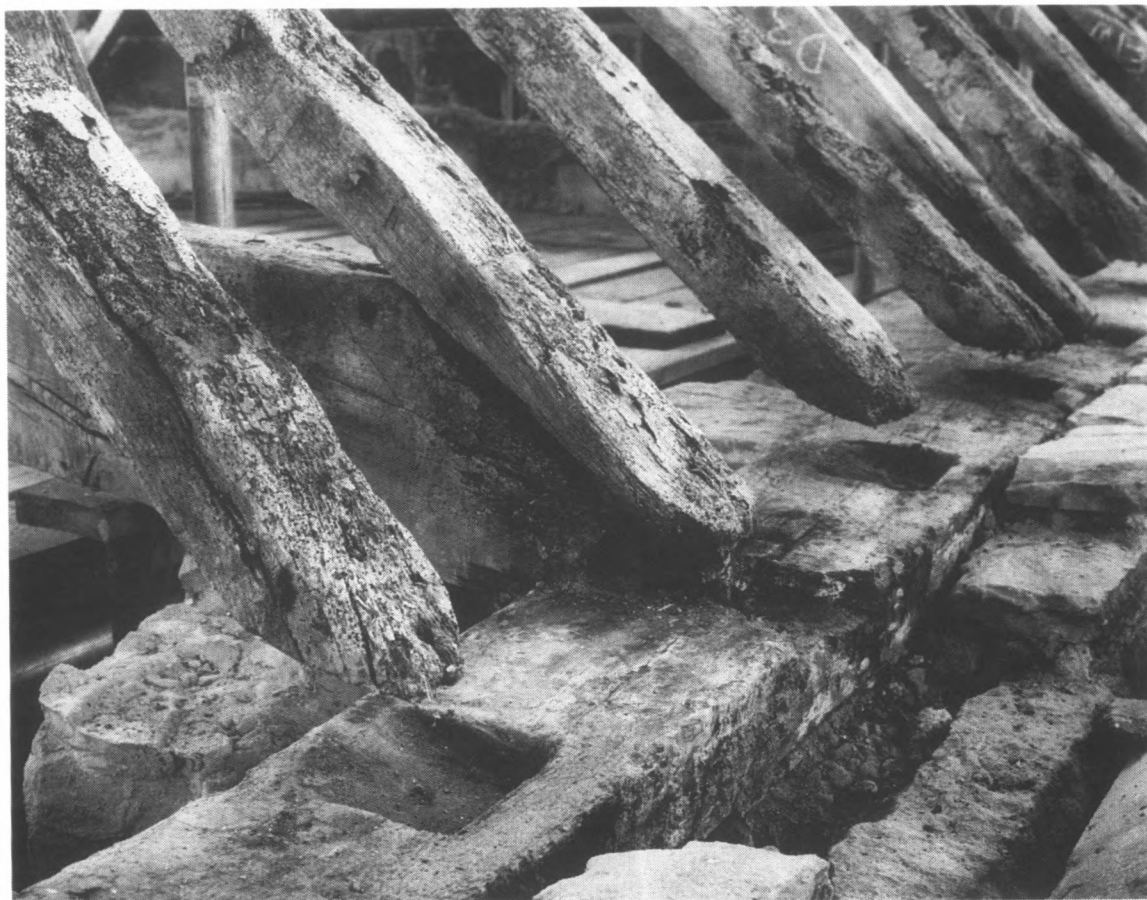
Fig. 10 Example of slots in wall plate for ends of original rafters near south end of west side. The ends were raised when deal boards were laid on the wall tops.
