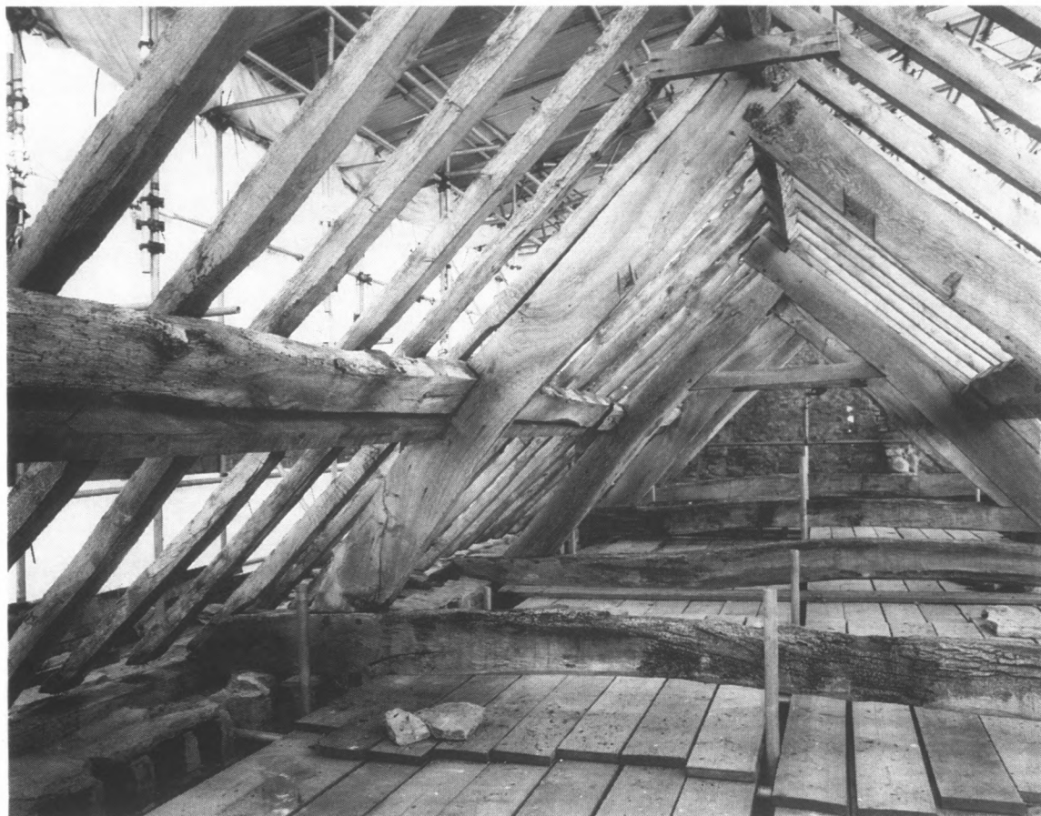
Fig. 9 West end of south face of truss D. Note curved end of principal, bark on the tie beam and thinner later purlin. Note also top row of nest holes in wall.
