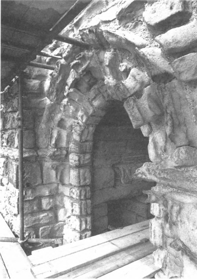
Fig. 13 Head of a clerestory window on the south side, showing severe weathering, 1996. © English Heritage/Jonathan Bailey.
