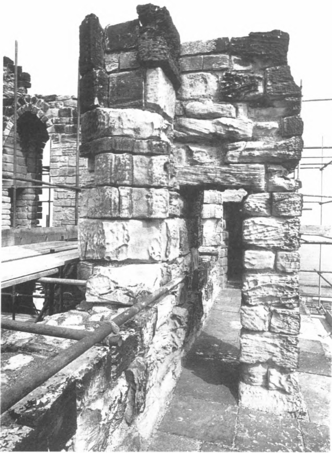
Fig. 14 Top of south wall, 1996, showing severe weathering and the sloping pavings laid c. 1914 to shed water. The window reveal is for the great chamber which was added above the vaulting. © English Heritage/Jonathan Bailey.
