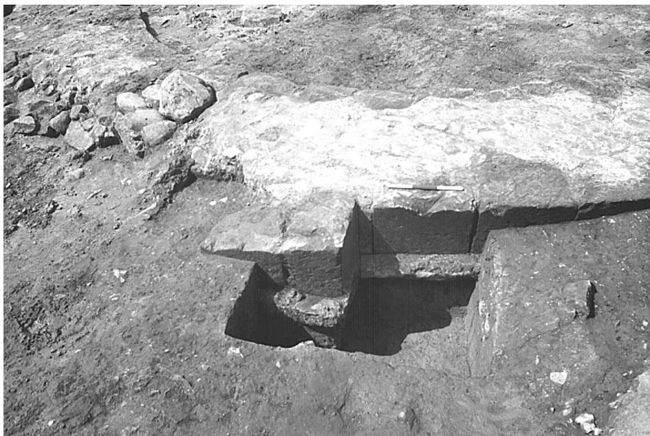
*Fig. 7 21 Castle Terrace. Section cut against the external face of apse wall showing one of the pilasters and the mortar foundation bed. Scale is 0.3m long.*
