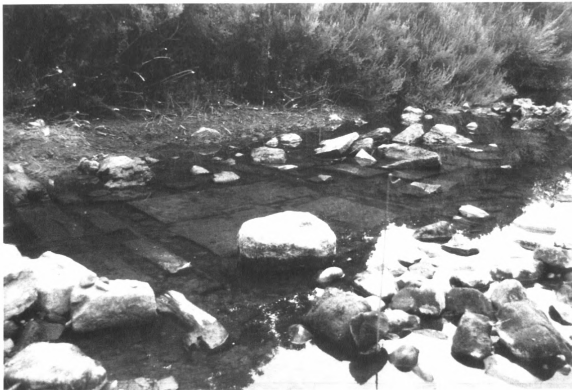
Fig. 9 The watermill during survey by Tyne and Wear Museums in 1995. Viewed from the west. At centre left, both ends of Timber 1 protrude from the water. In the centre the wheelhouse floor is overlain by a large boulder. The displaced blocks from the outfall are at centre right.
