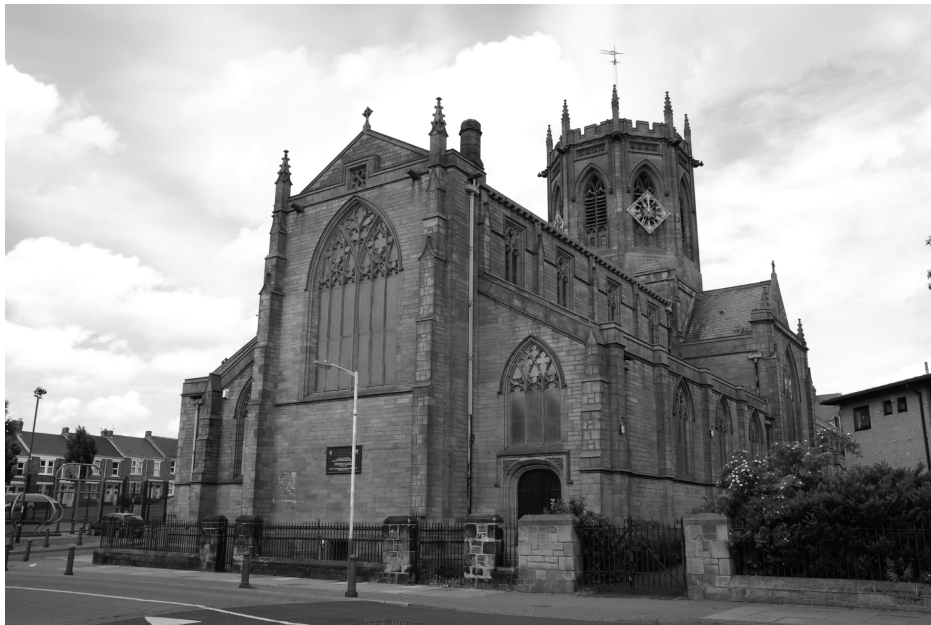
Fig. 6 Bensham (Gateshead), St Chad.
