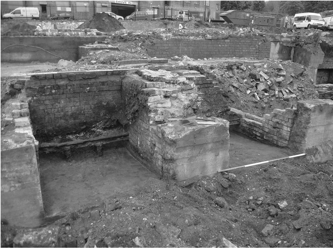
Fig. 8 The two central furnaces, in the north-west extension of Building 1, which would have significantly increased the capacity of the works. The refractory-brick superstructure and bull-nose rail can be seen in each furnace, as can the cast concrete facing that retained the imprint of the wood shuttering from its construction.
