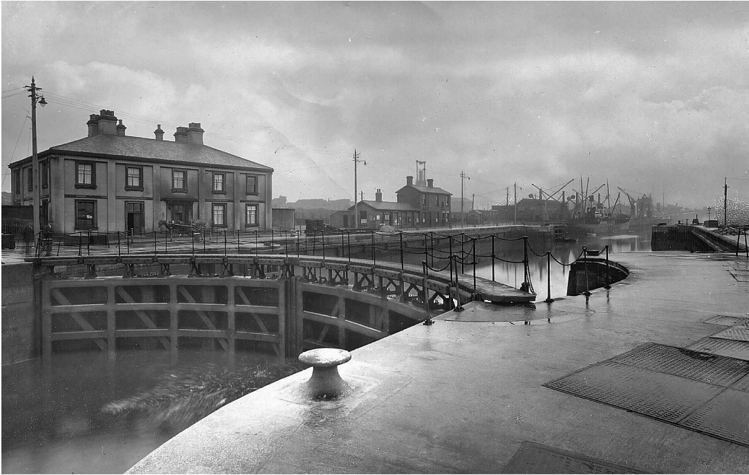
Fig. 9 A photograph of the north gates of the Sixty-Foot Lock looking south-east with the Custom House and Dock Manager's Office beyond the entrance. Probably taken in the mid 1920s. With thanks to the Port of Tyne Authority.
