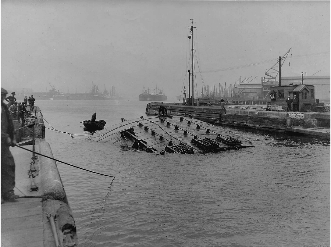
Fig. 12 Photograph from 1935 showing the north-east gate of the WMP being floated along the Seventy Foot Entrance for refurbishment. With thanks to the Port of Tyne Authority.
