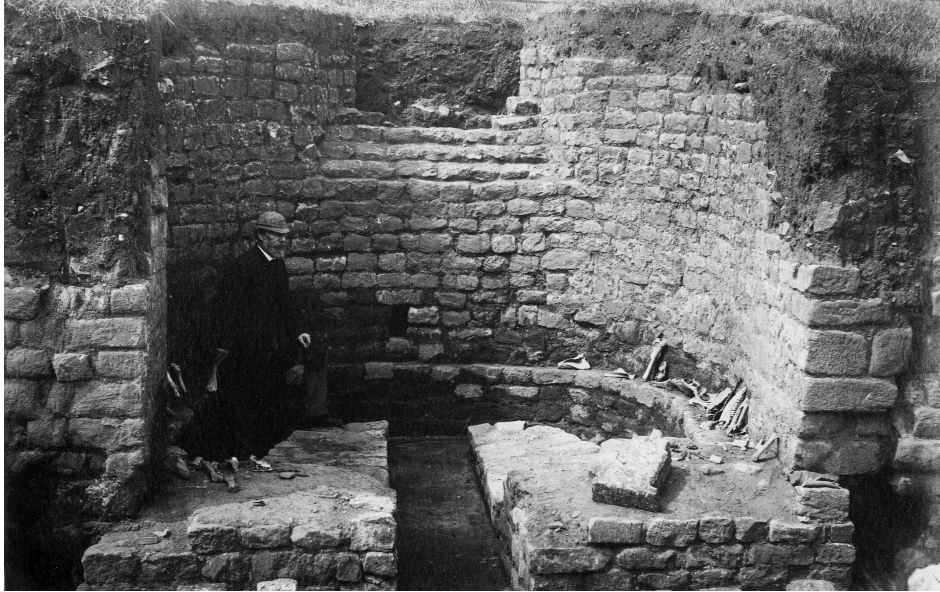
Fig. 6.i William Tailford Jnr standing in the excavated apse of the caldarium with finds including a tufa voussoir, hypocaust pila and animal bones on display; viewed from the east. (The Victorian caption reads 'River-side buildings', rather than 'Baths'.) Photograph by J. P. Gibson, 1884 (Copyright Tyne & Wear Archives and Museums).
