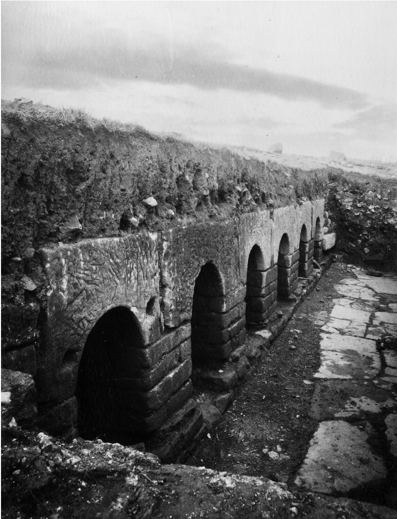
Fig. 4 Start of clearance of the interior of the changing room, viewed from the south; the arch of the northernmost niche collapsed. (The Victorian caption reads 'River-side buildings', rather than 'Baths'.) Photograph by J. P. Gibson, 1884 (Copyright Tyne & Wear Archives and Museums).
