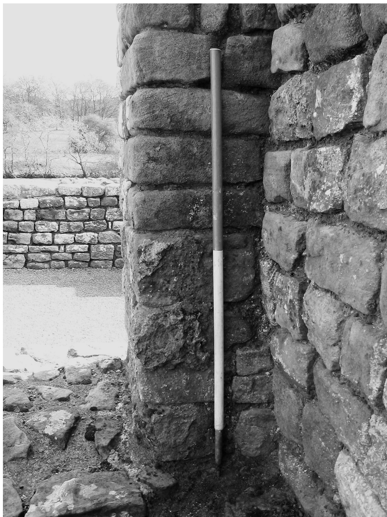
Fig. 23 Inner face of the southern arch respond of the apse. At centre left remnants of red plaster. Photograph, the authors.
