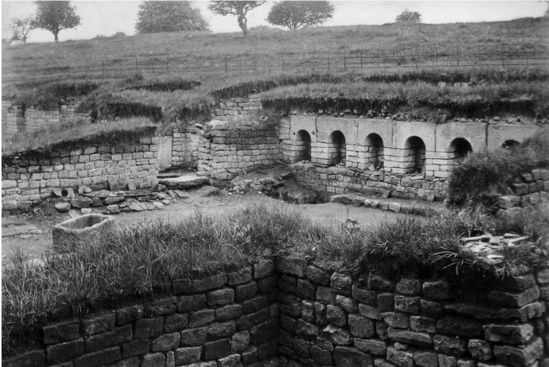
Fig. 8 Photograph by J. P. Gibson of the northern part of the building, sometime after July 1886, viewed from the north-east. Part of the porch in the right foreground, a sondage dug in the south-west corner of the changing room, finds on display against the south wall (Copyright Trustees of the Clayton Collection and English Heritage).
