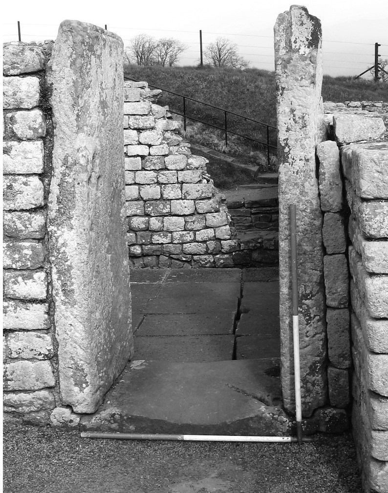
Fig. 20 Monolithic stone jambs in doorway between ante-room D and laconicum B, viewed from the south. Photograph, the authors.
