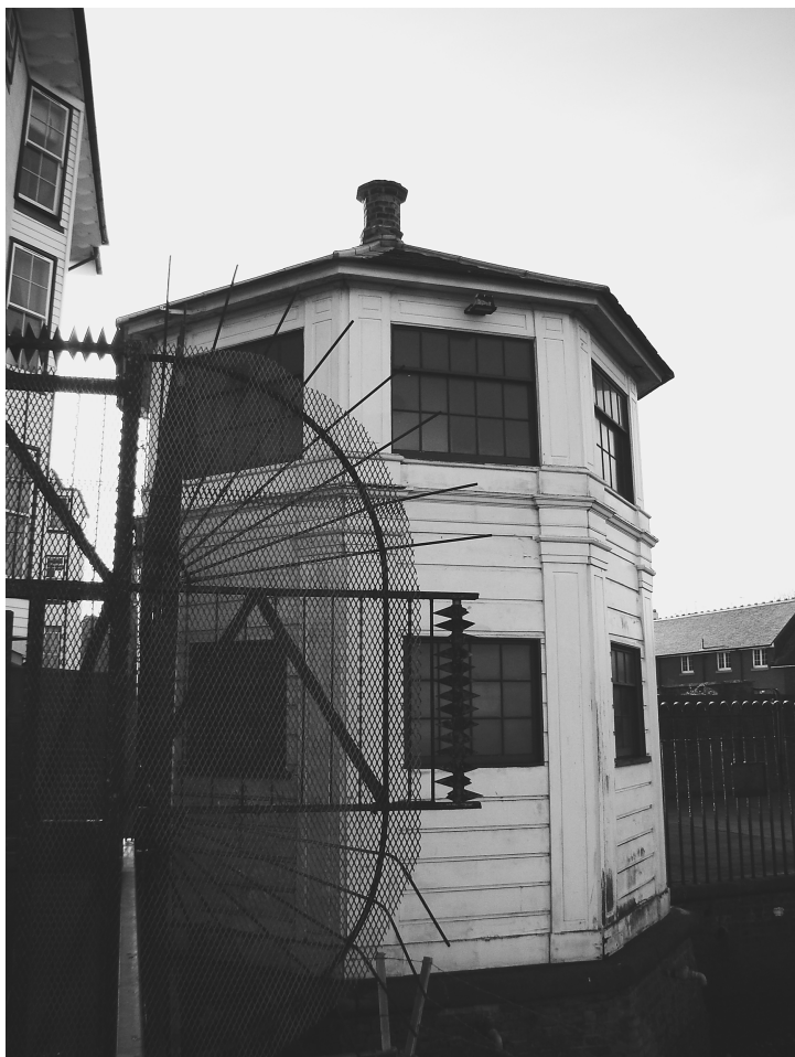
Fig. 4 Tidewaiters' tower, Gravesend, Kent. Photograph and permission to publish from Conrad Broadley.
