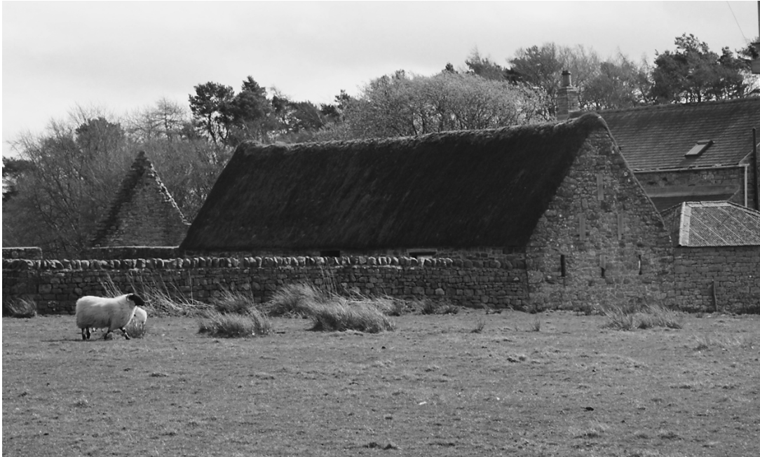
Fig. 14 High Meadow Barn — later 18th- or early 19th-century heather-thatched structure.
