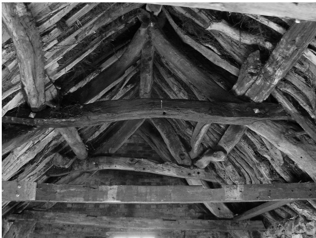
Fig. 5 Interior of barn roof looking north, December 2013. The sawn timbers have been added, perhaps in the late 19th century, to control spread of crucks.
