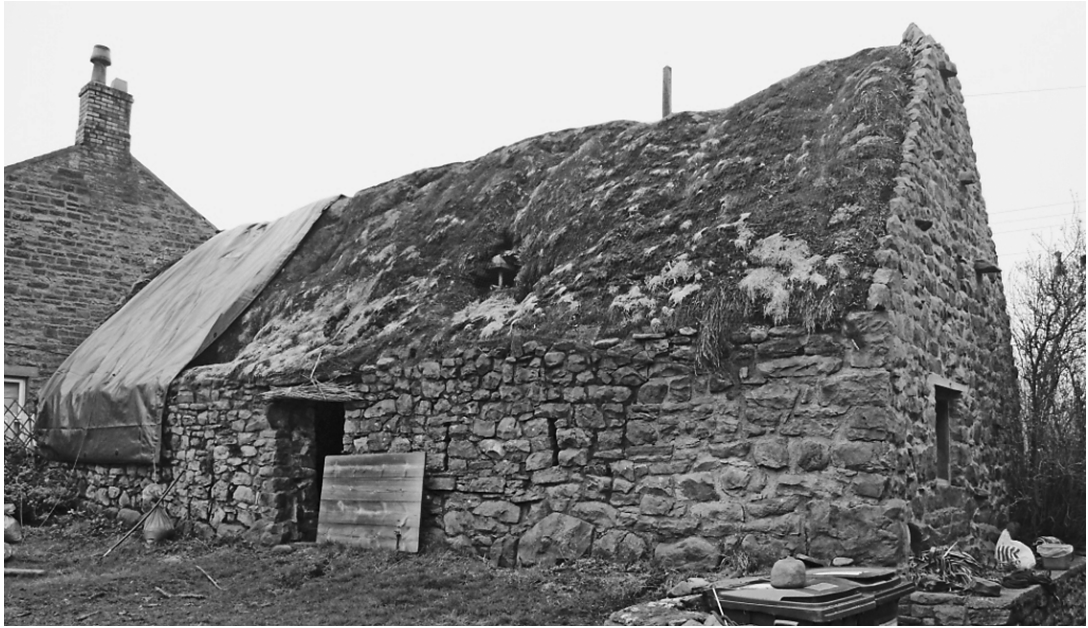
Fig. 3 South-west side of Black Barn 2010. The failure of the thatch is evident.
