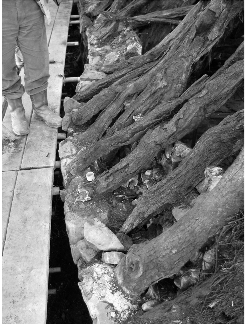
Fig. 7 The south-west eaves wall showing effect of spreading trusses and rafters.
