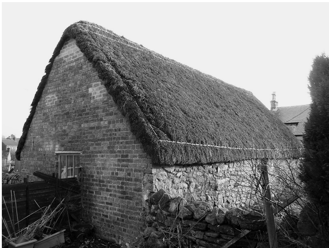
Fig. 10 The exposed ridge eaves and gables are reinforced against wind with liggers.
