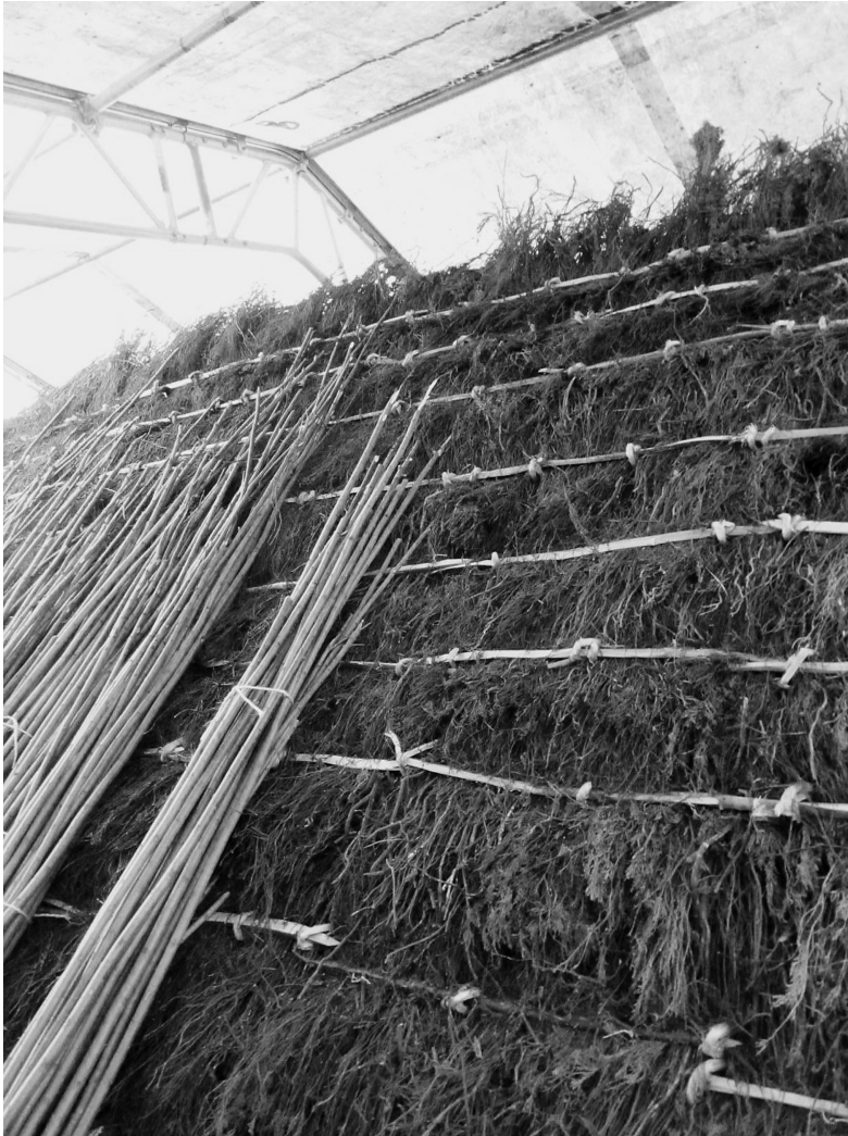
Fig. 9 The waist coat is fixed with hazel sways and spars (or staples).
