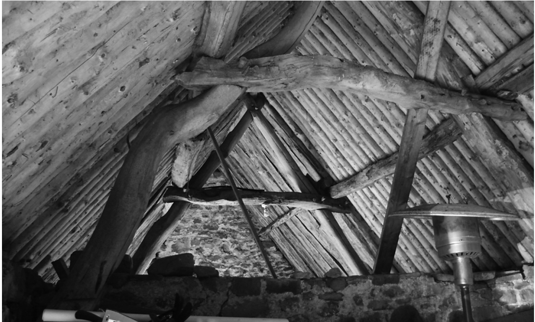
Fig. 15 High Meadow Barn — interior. The rafters renewed in round-pole in the 1990s and re-thatched.
