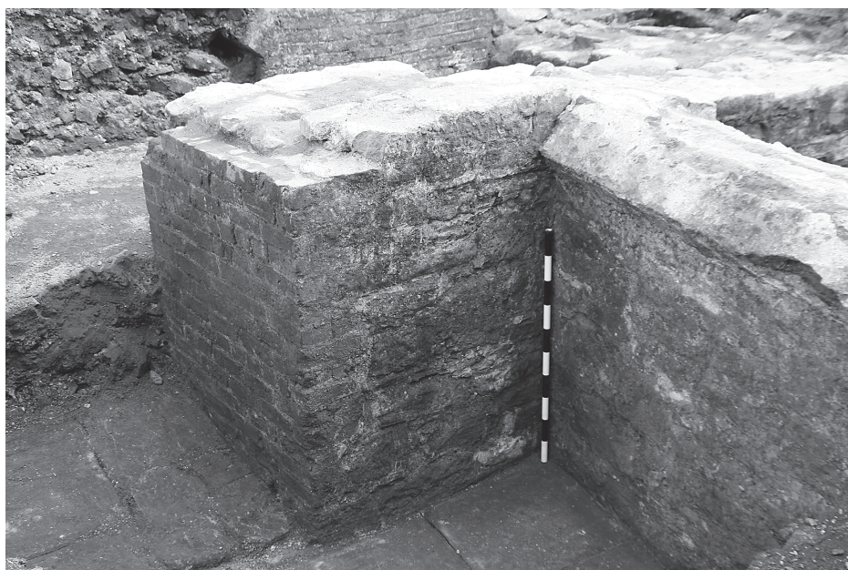
Fig. 25 Trench 2; Period 3 cellars, junction of wall [33] (with brick addition [38], centre, left) and wall [34] (brick addition [29], right); flagstone floor [36]; looking south-east (1 m scale).
