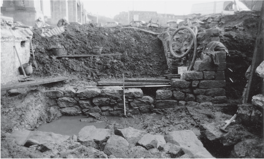
Fig. 11 Walls [122] and [122.1] from the north.
