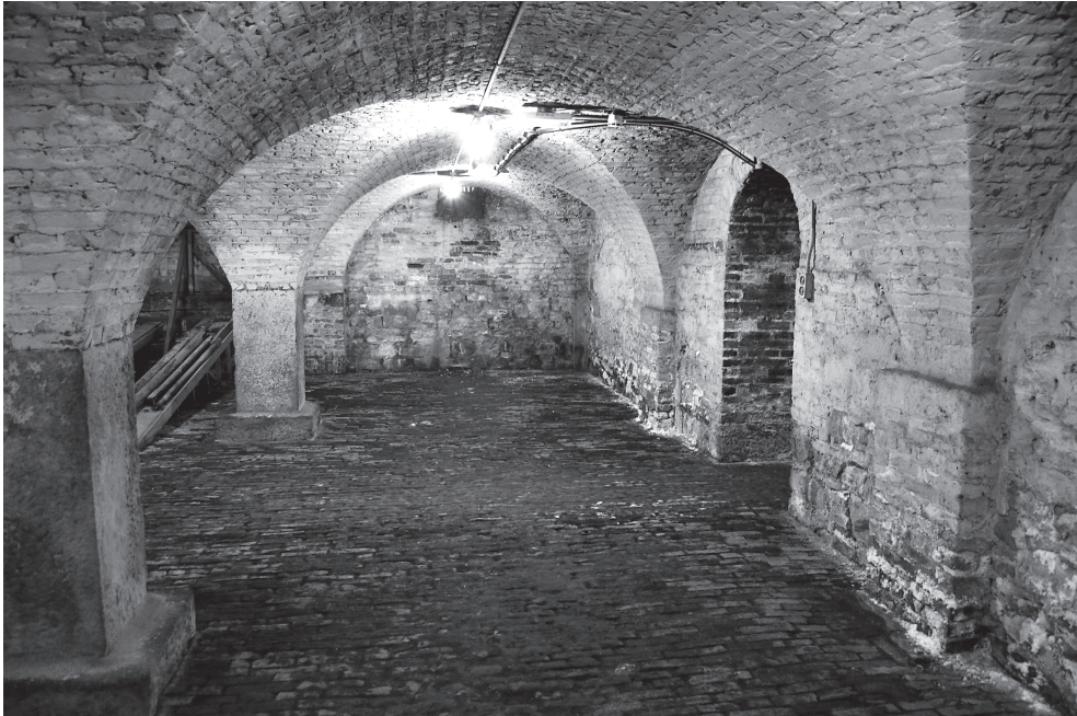
Fig. 4 The vaulted cellars beneath Custom House.
