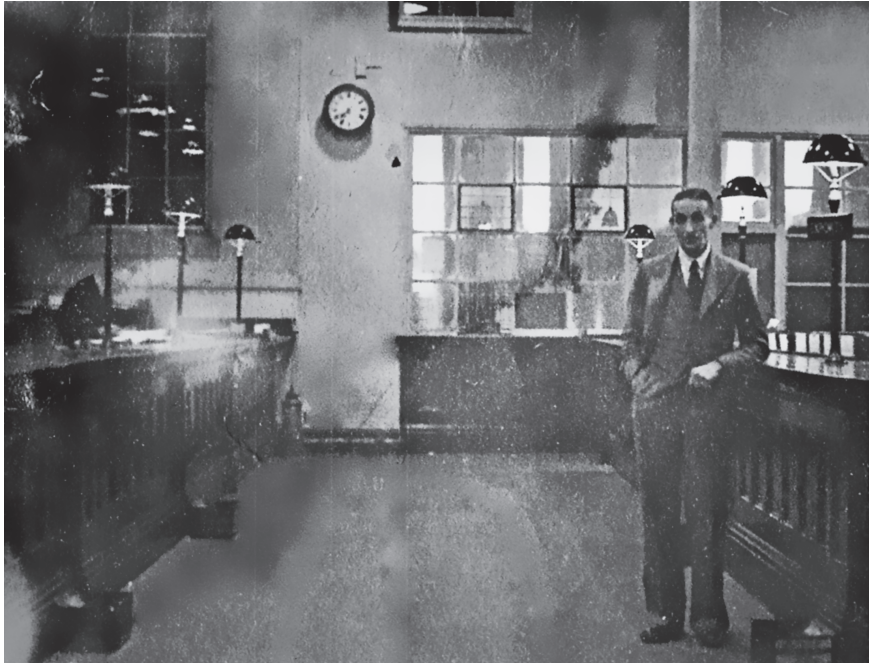
Fig. 10 Interior of the Long Room c. 1955, with counters for imports on left and exports on right. (Photo: Mrs Enid James). The column behind William Burn (Deputy Collector) indicates the line of the east wall of Smirke's Long Room, before its extension in the early twentieth century.
