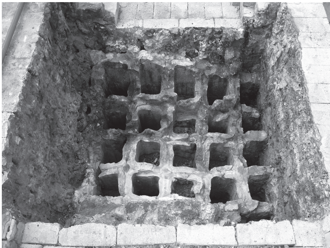
Fig. 12 Detail of recuperator tubes.
