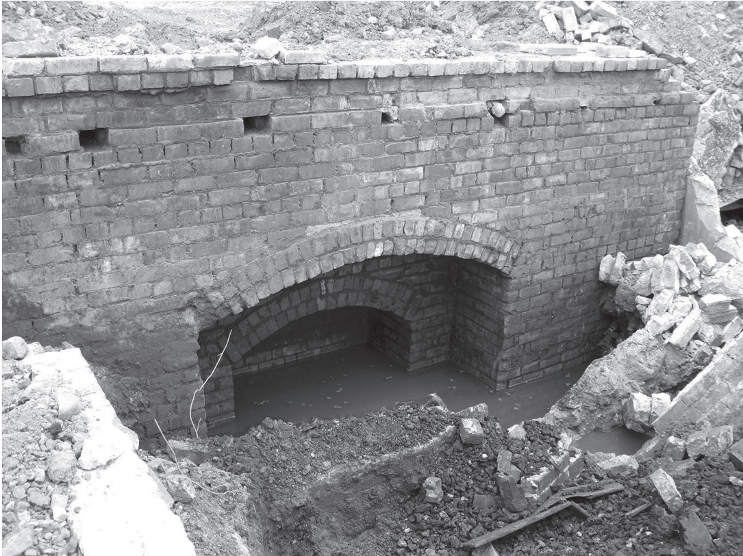
Fig. 9 Furnace 5 and its cave opening.
