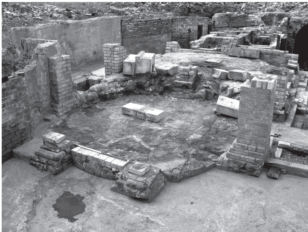
Fig. 11 Columns supporting the tank of the PYREX furnace.
