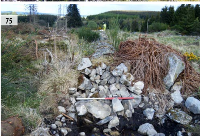
PLATE 73 View of the road corridor and the upstanding stoen dykes PLATE 74 General view of Dyke AMA19 PLATE 75 East facing section through Dyke AMA17 showing the random rubble construction PLATE 76 View of Dyke AMA18
