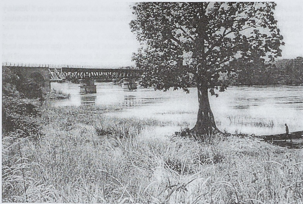
Fig. 5 The old rail/road bridge across the Niger at Jebba. Photo. by F.N.Hepper, 7-10-57
