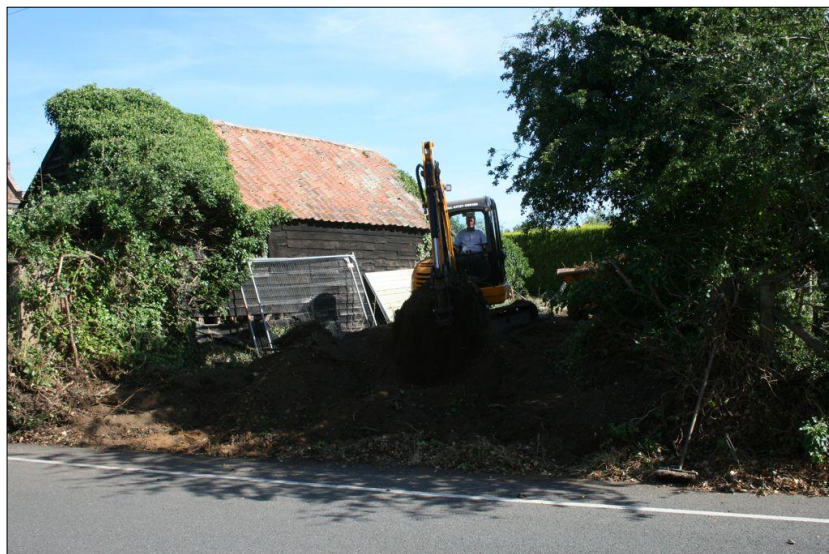
Plate 5: Drive east of barn, topsoil stripping
