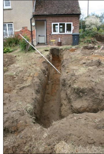
Plate 2: Extension footing, south trench
