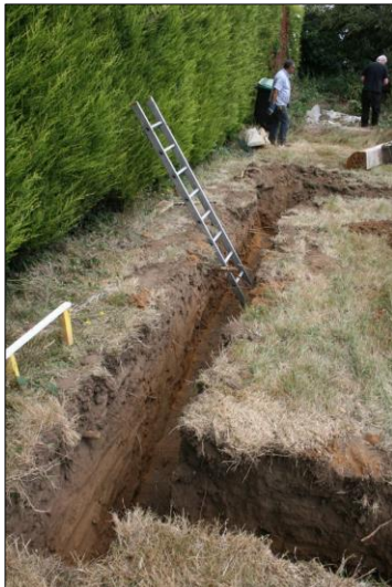
Plate 3: Garage footing, north trench
