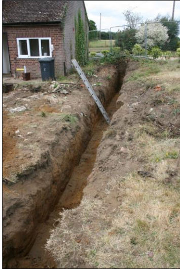
Plate 1: Extension footing, north trench
