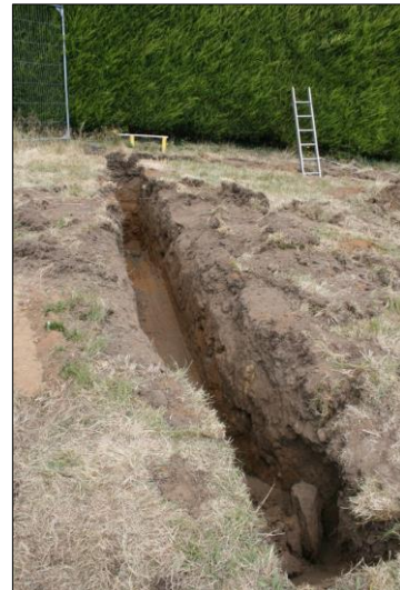
Plate 4: Garage footing, west trench
