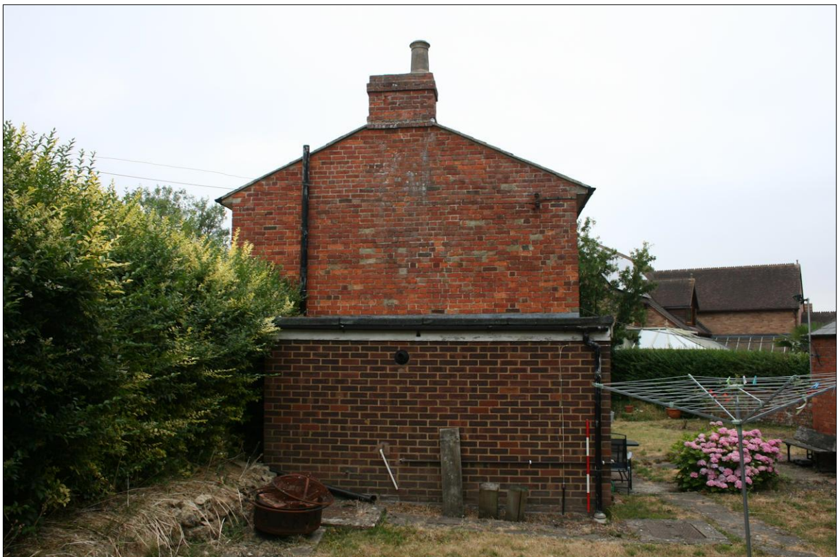
Figure 16: Outbuilding, west elevation from west
