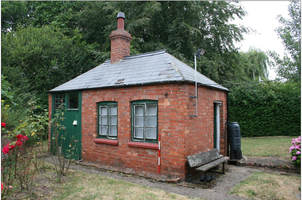
Figure 31: Outbuilding, east elevation from north-east
