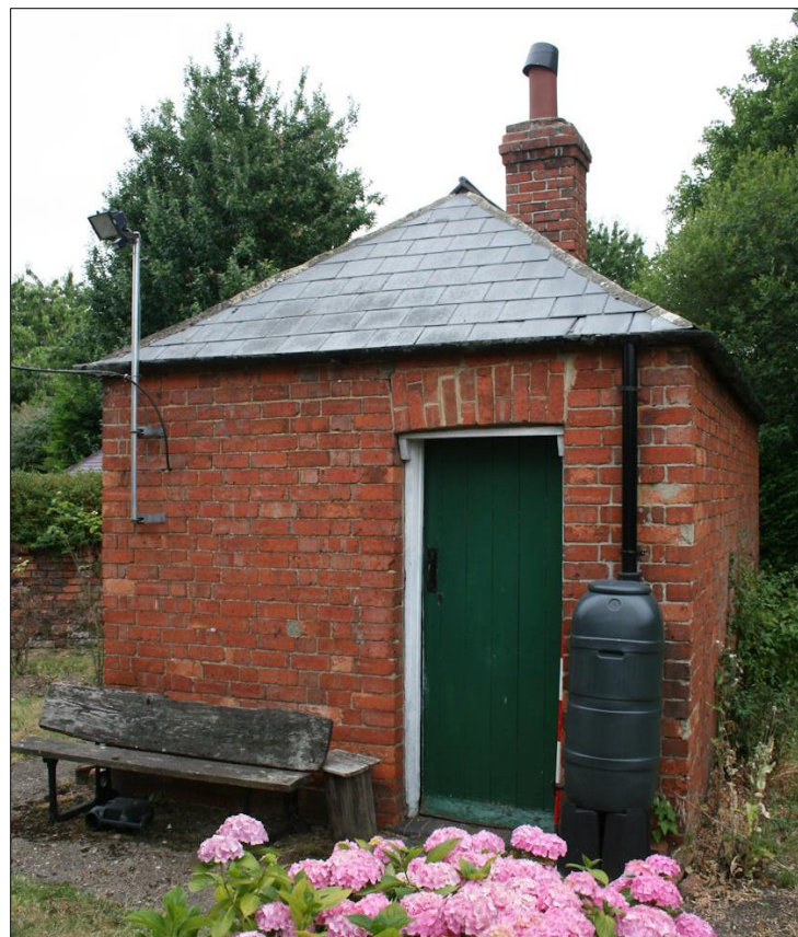
Figure 30: Outbuilding, north elevation from north
