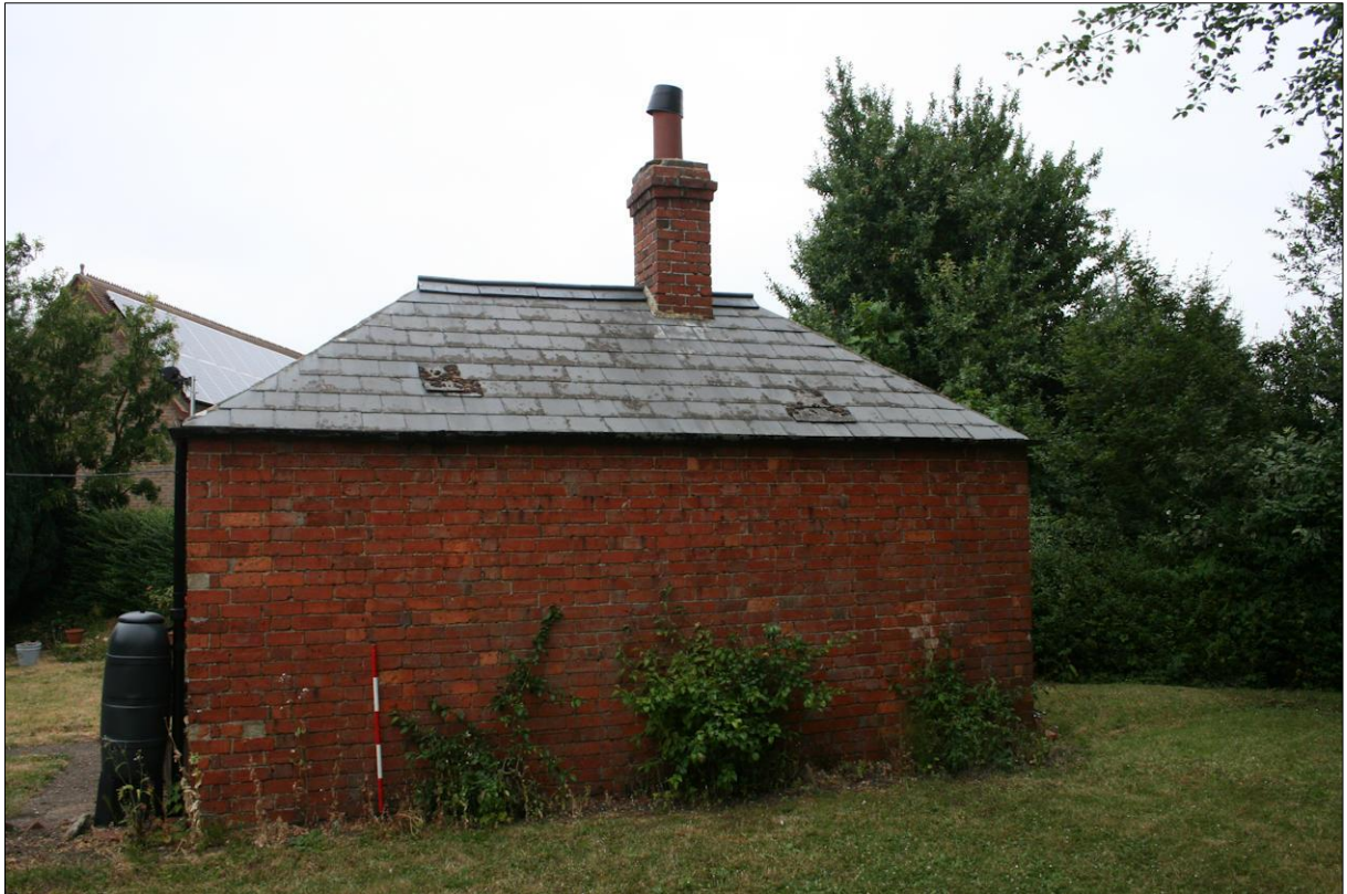
Figure 33: Outbuilding, west elevation from west
