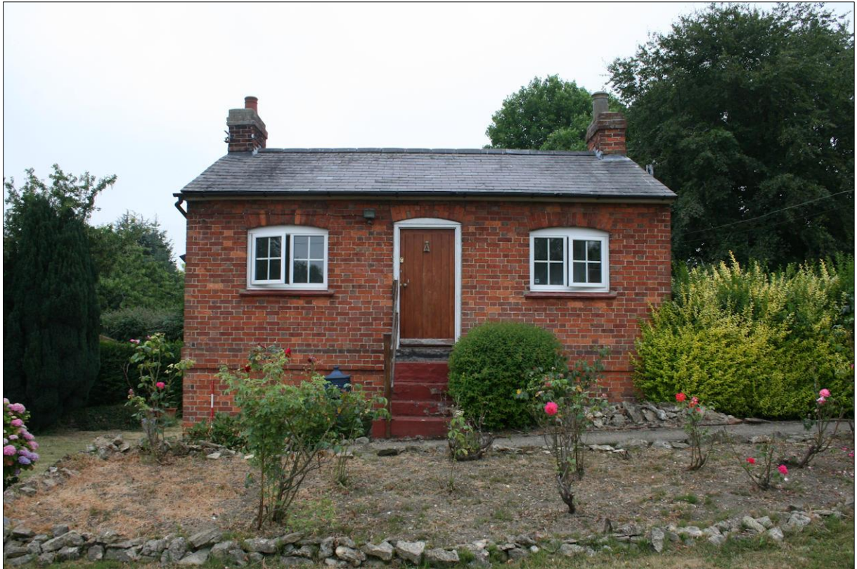
Figure 13: Cottage, north elevation from north
