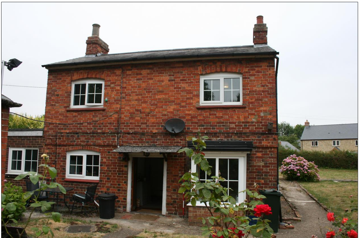
Figure 14: Outbuilding, south elevation from south
