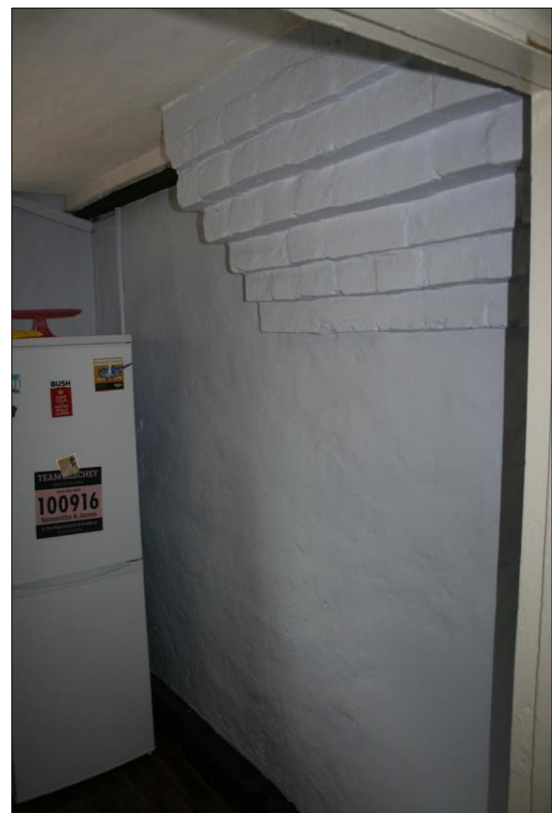
Figure 22: Cottage, G3 kitchen looking south-west
