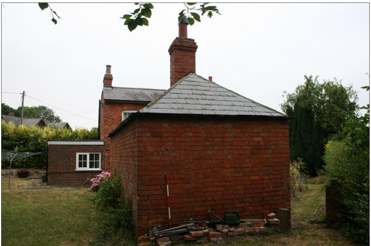
Figure 32: Outbuilding, south elevation from south
