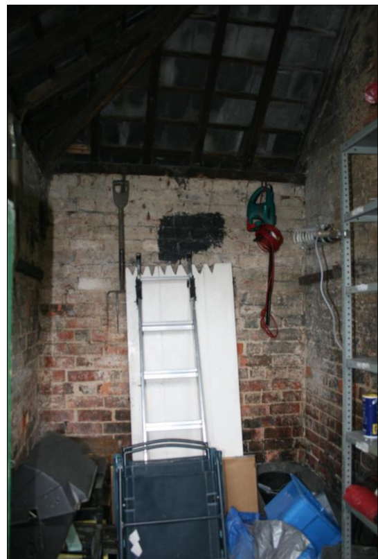
Figure 35: Outbuilding, OB2 'garage' looking west
