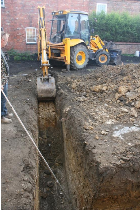
Figure 7: Excavating the deep rear (NE) trench, looking SE
