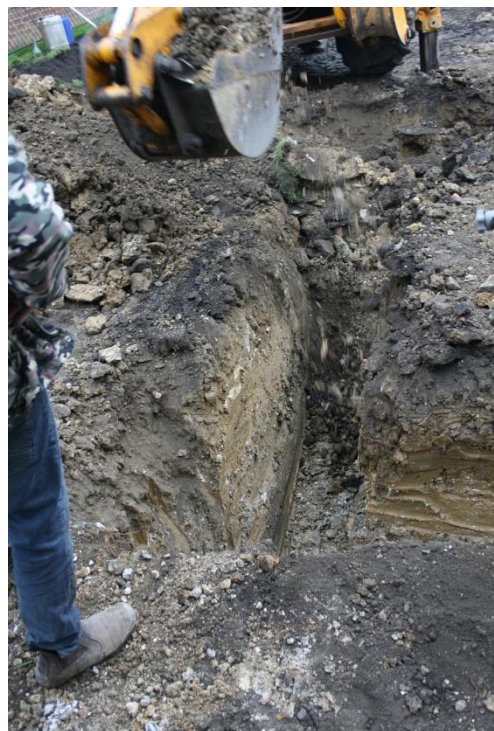
Figure 10: Excavating the SE trench, looking SW
