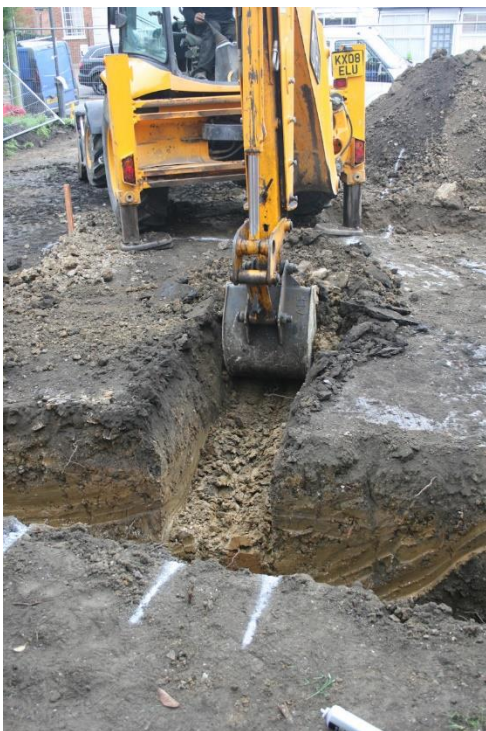
Figure 9: Excavating the shallow central trench, looking SW
