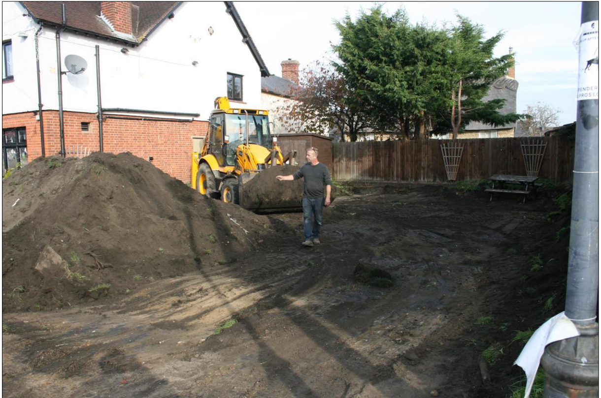
Figure 5: The site during topsoil removal, looking north
