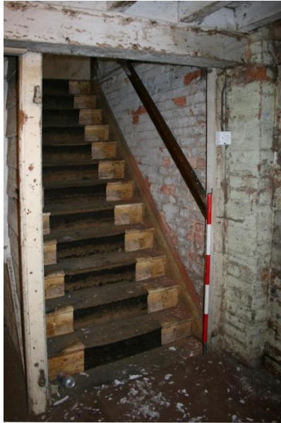
Plate 31: F1 landing, stairs to second floor
