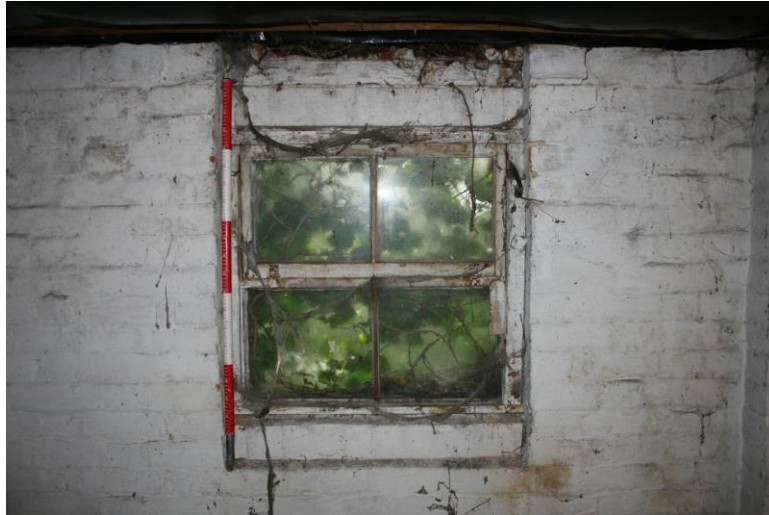
Plate 34: S1, detail of hopper window on south side
