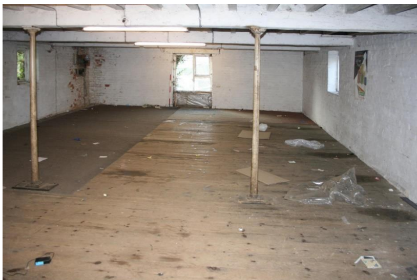
Plate 24: F1, looking west
