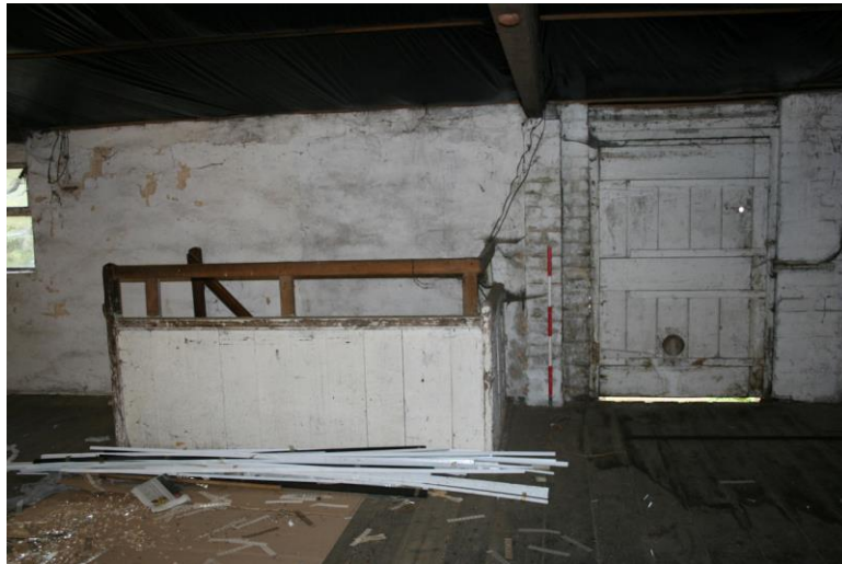
Plate 35: S1, top of stairs and taking-in door on north side
