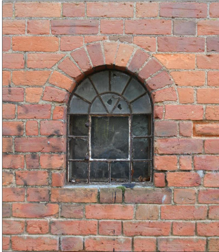
Plate 4: Building 2, close-up of small arched window in north elevation
