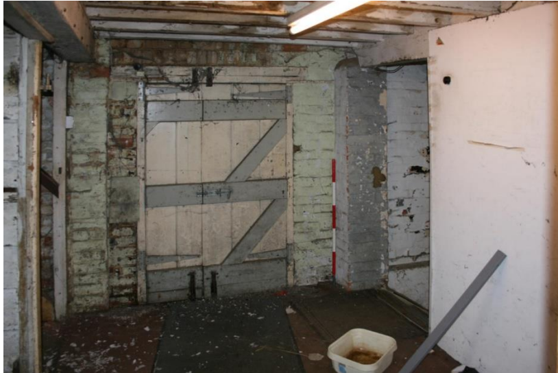
Plate 22: F1 landing, looking north
