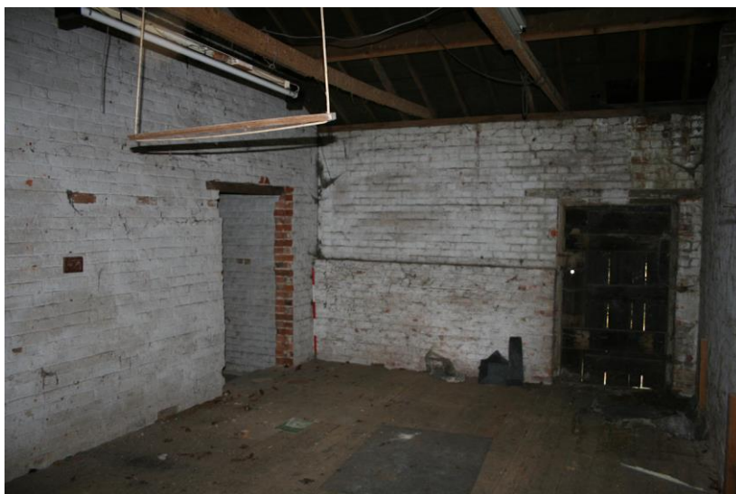
Plate 30: F4, looking north
