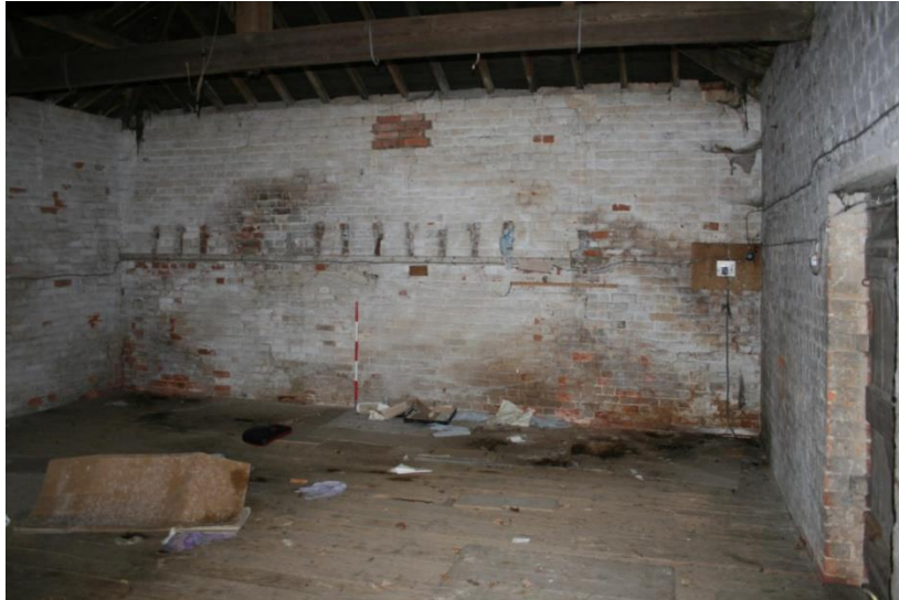
Plate 28: F3, looking west
