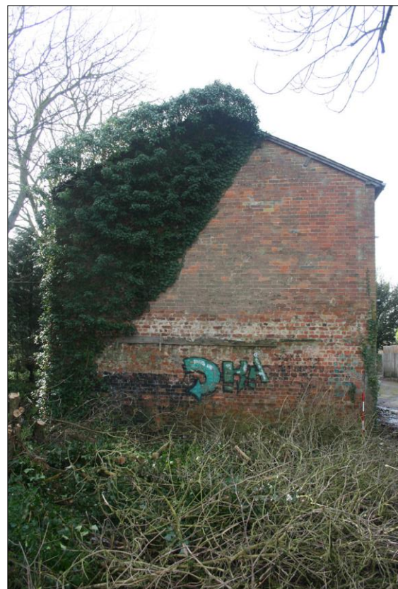
Plate 3: Building 2, east elevation from east
