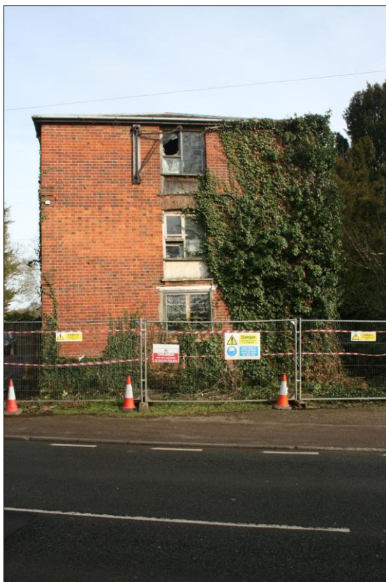
Plate 2: Building 1, west elevation from west
