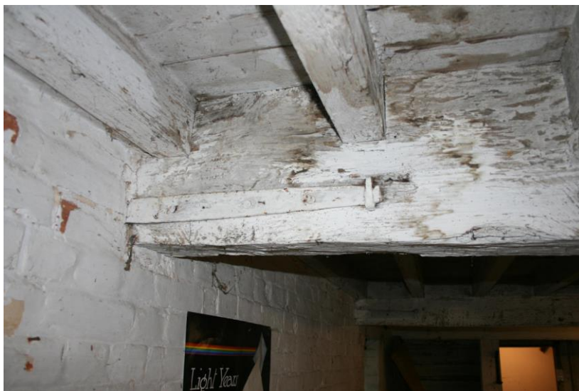
Plate 26: F1, detail of strapping on principal joist
