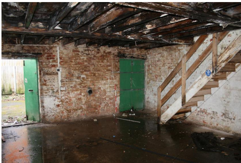
Plate 17: G5, looking north-east
