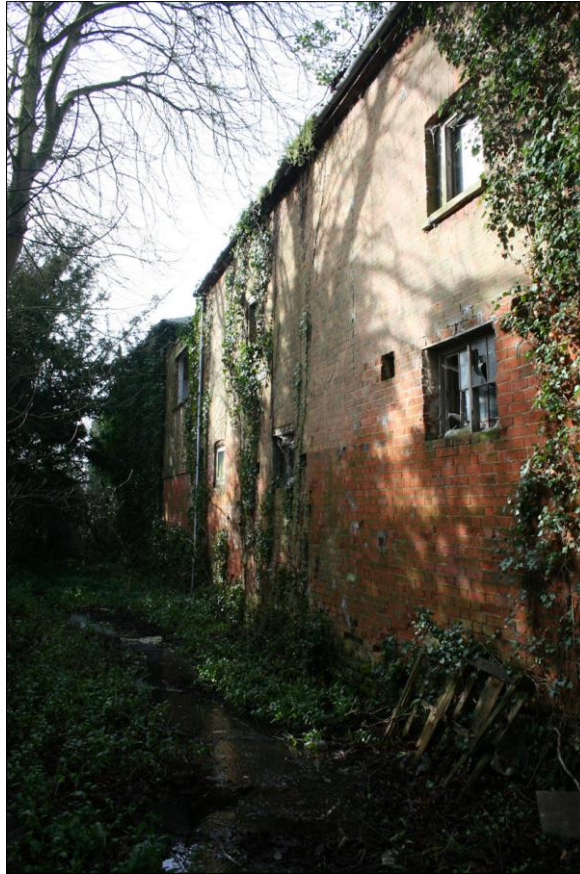
Plate 1: Buildings 1 & 2, south elevations from south-east
