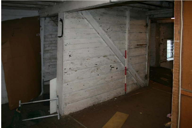
Plate 25: F1, detail of timber partition enclosing stairs
