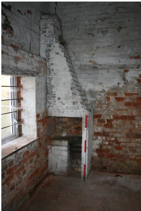
Plate 14: G4, detail of hearth in north-east corner
