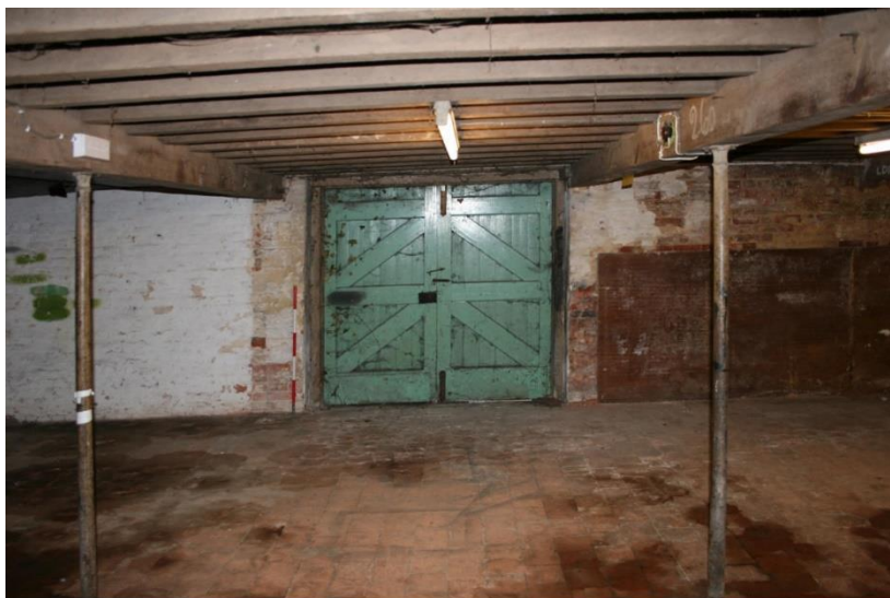
Plate 7: G2, detail of double doors to north
