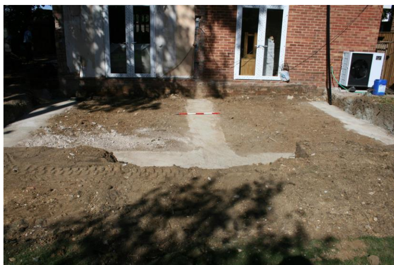
Figure 8: South extension footings with oversite reduced, from south
