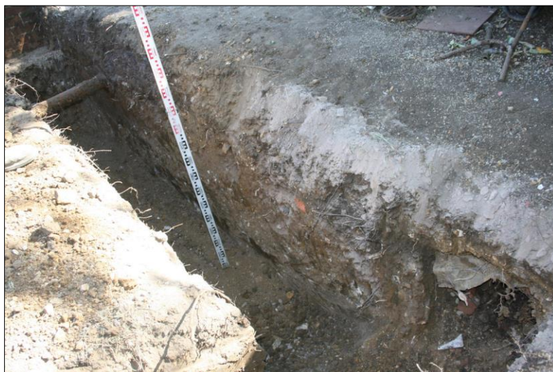
Figure 11: West extension footings: south trench, from north-west
