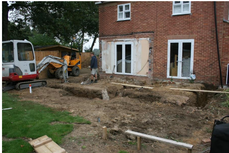
Figure 6: Excavating south extension footings: general view from south-east
