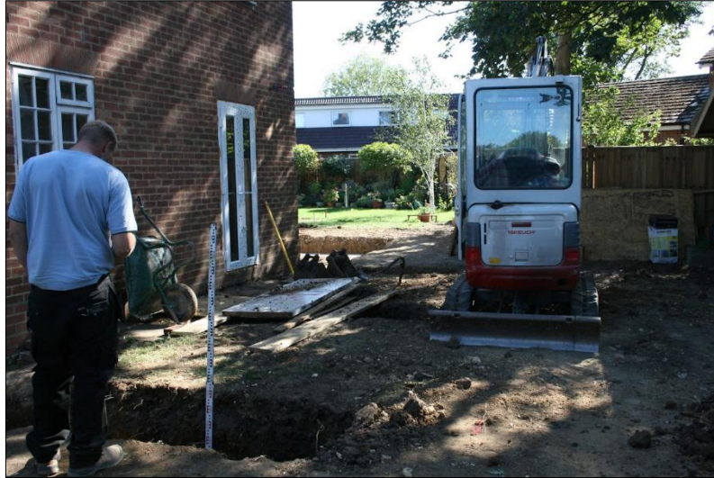
Figure 9: General view during excavation of west extension footings, from north
