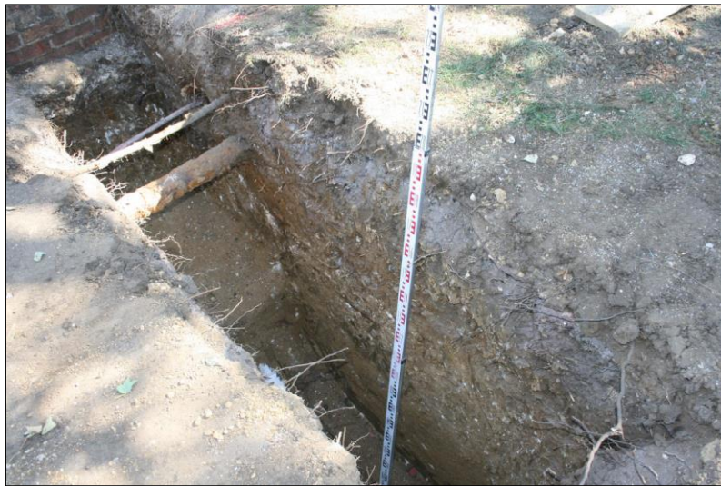
Figure 10: West extension footings: north trench, from north-west
