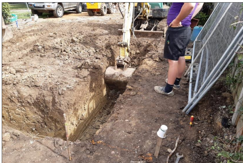
Figure 8: Excavating the east side footing trench
