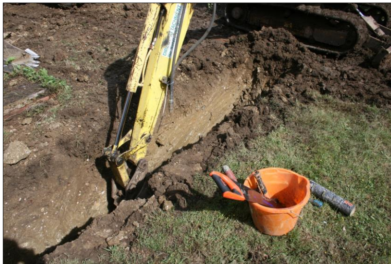
Figure 7: Excavating the south side footing trench
