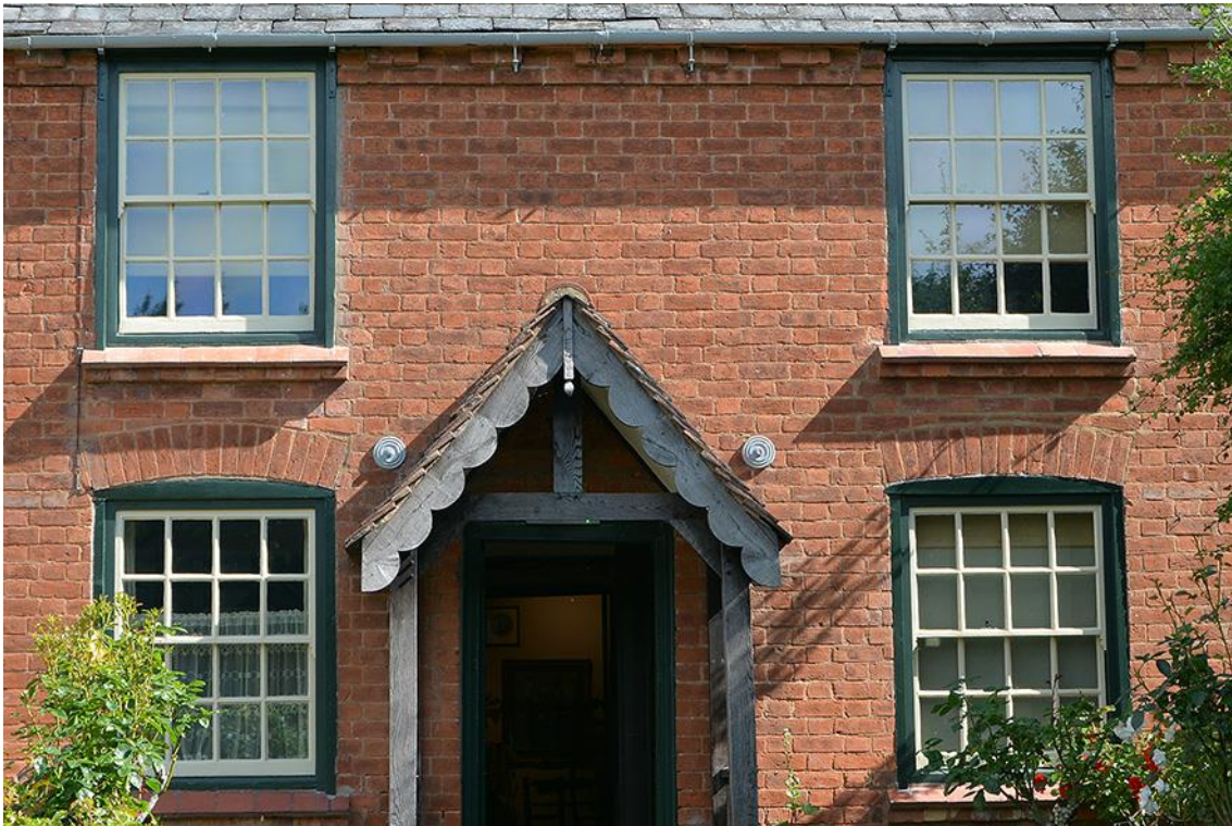
Plate 22: South, front, wall the cottage showing all four windows with sash horns
