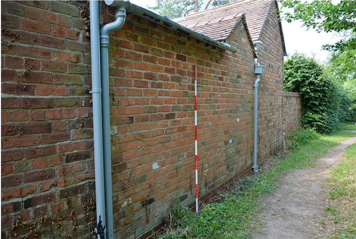
Plate 21: Northern wall of outbuildings from the north east
