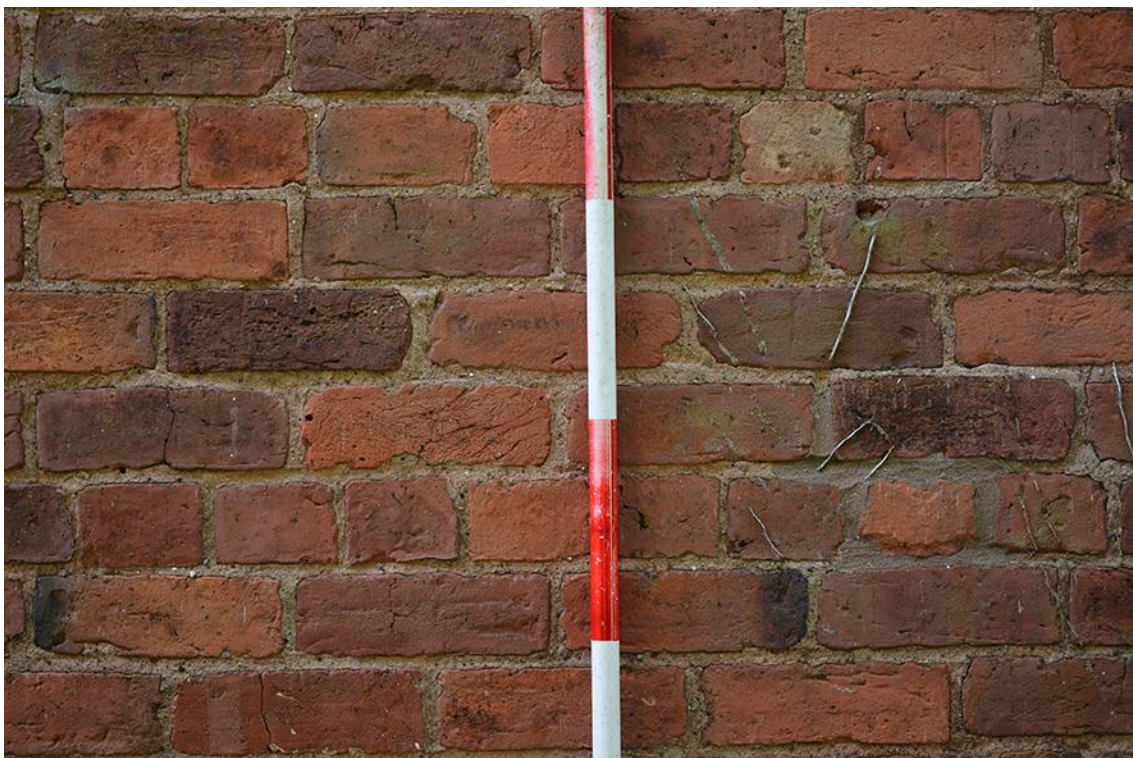
Plate 5: Detail of brickwork on original part of building
