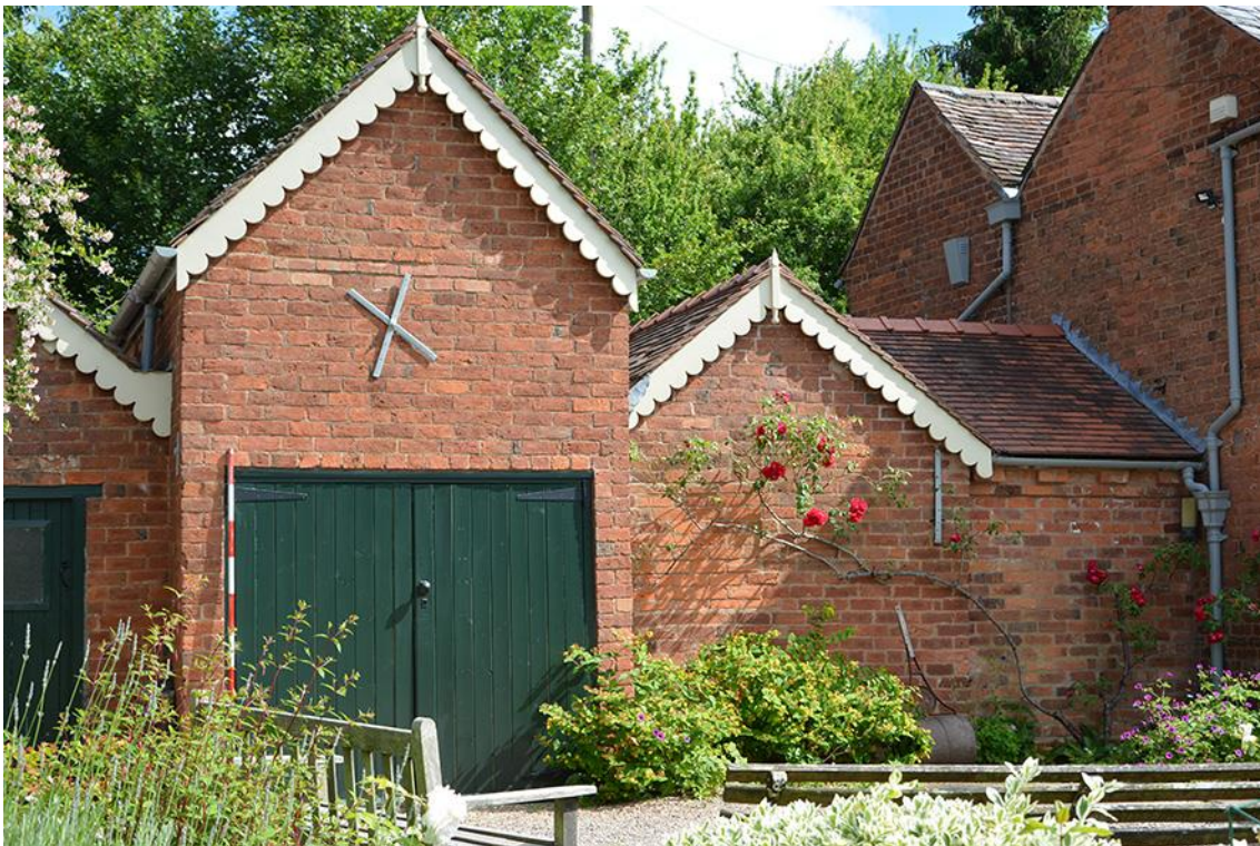
Plate 3: South elevation of adjoining outbuildings
