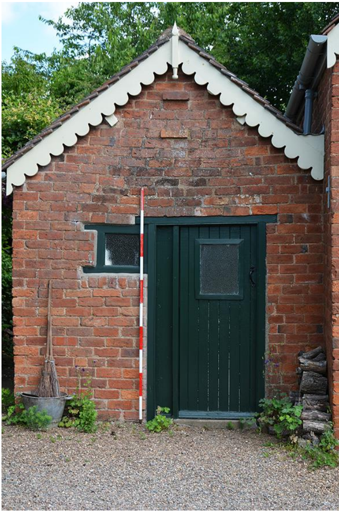
Plate 13: Stable of 1856 construction
