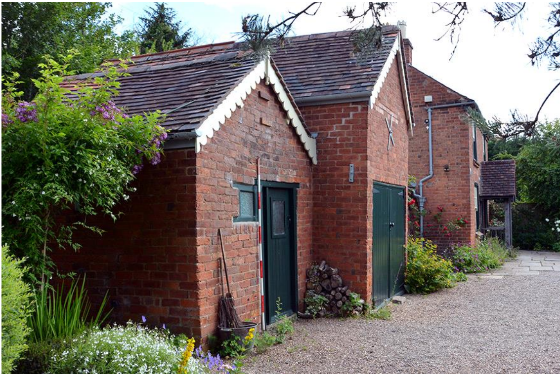
Plate 4: South elevation of adjoining outbuildings
