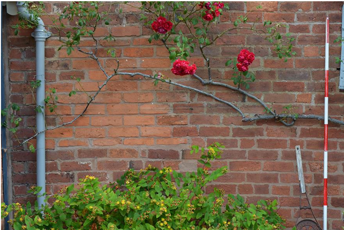
Plate 16: Blocked window in south elevation of former washhouse
