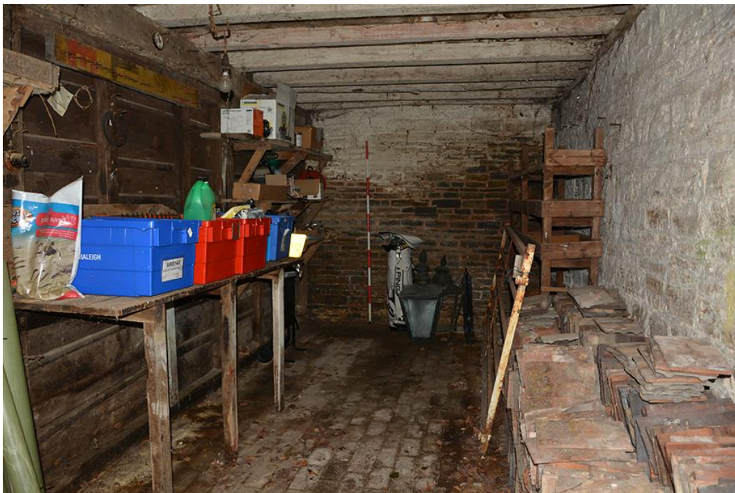
Plate 22 Cart shed, east end garage space
