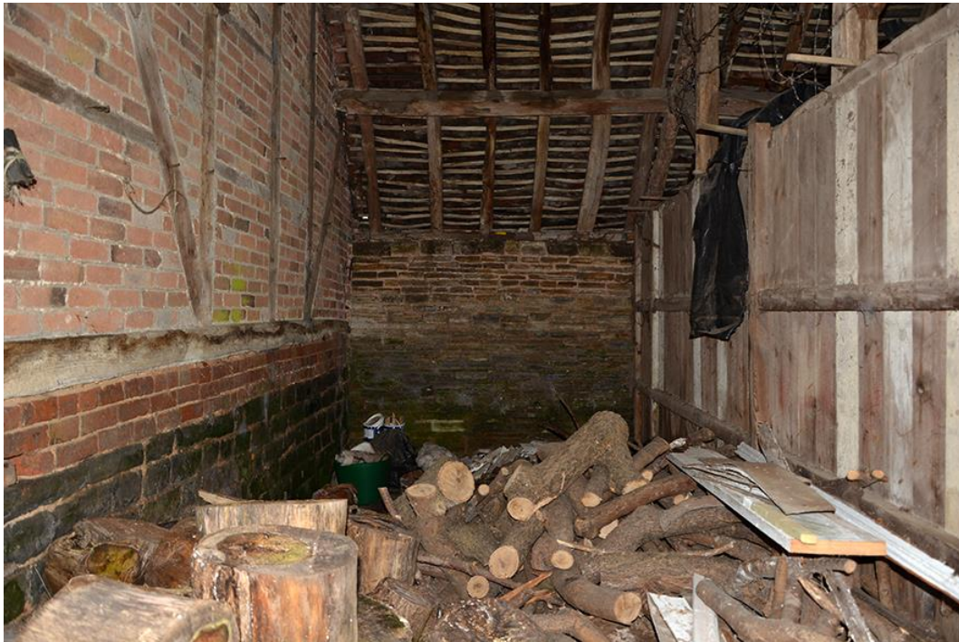
Plate 21 Cart shed, west end
