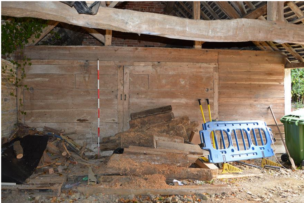
Plate 28 Cart shed interior division of reused timber panels
