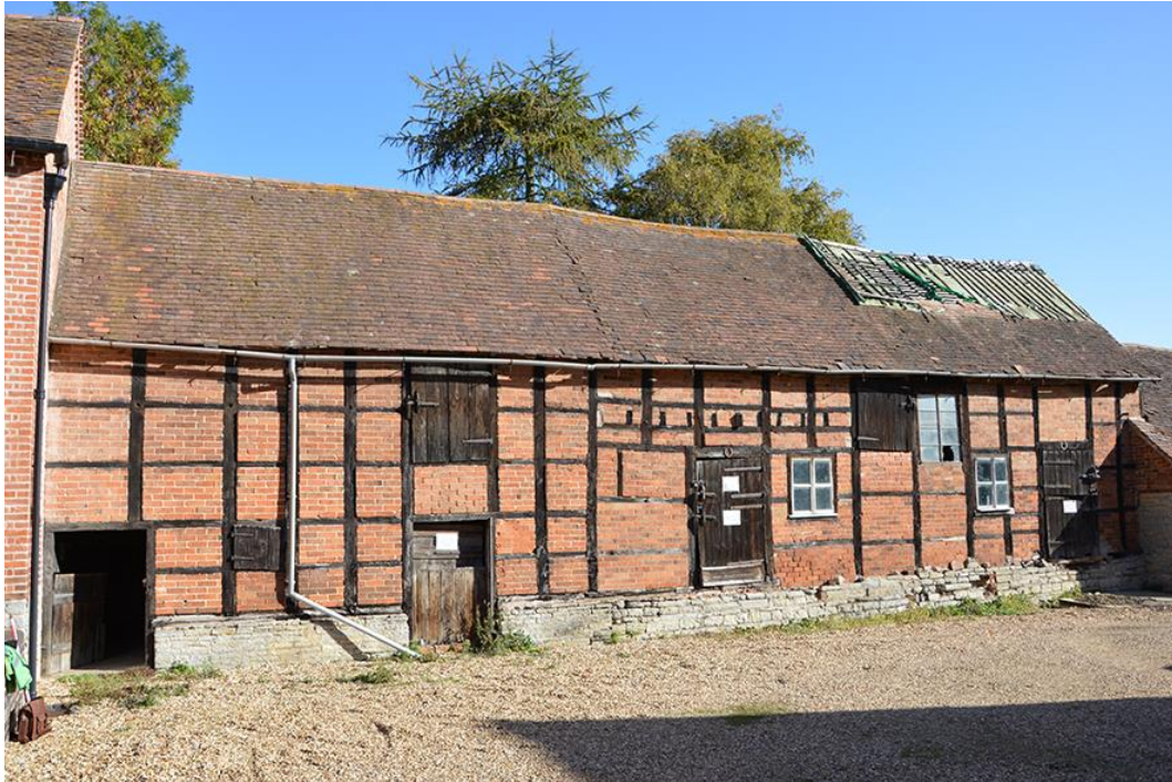
Plate 1 Timber-frame building from the south west
