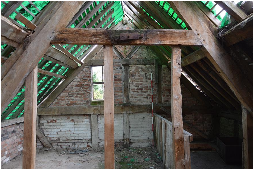
Plate 17 Eastern section, first floor interior
