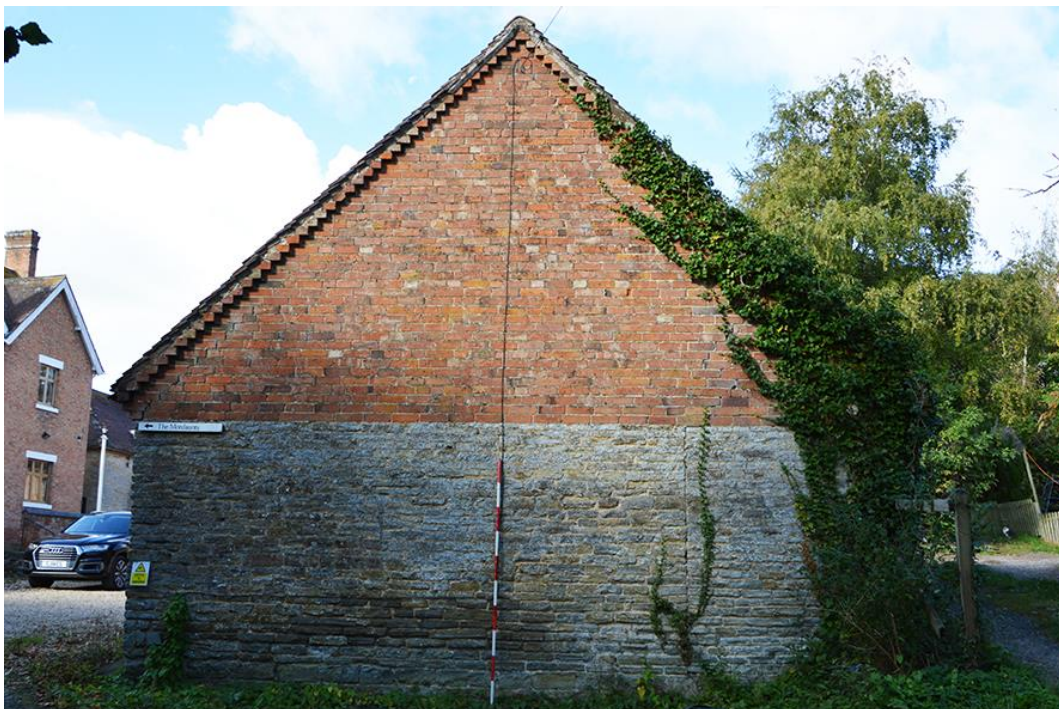
Plate 26 Cart shed gable with building break to right of ranging rod
