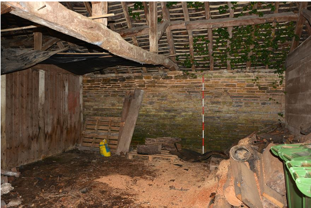
Plate 24 Cart shed, central area
