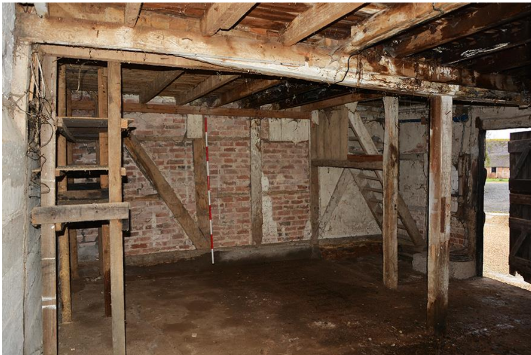
Plate 16 Eastern section, ground floor interior, note stairs
