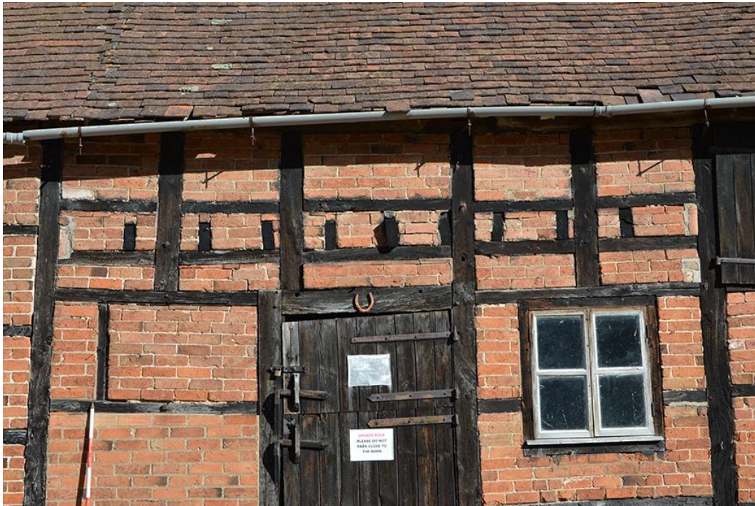
Plate 25 Timber joists of inserted floor in timber-frame building
