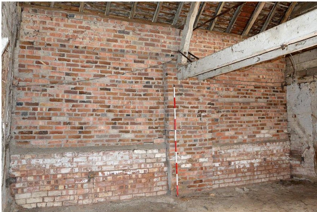
Plate 11 Central section interior, north wall
