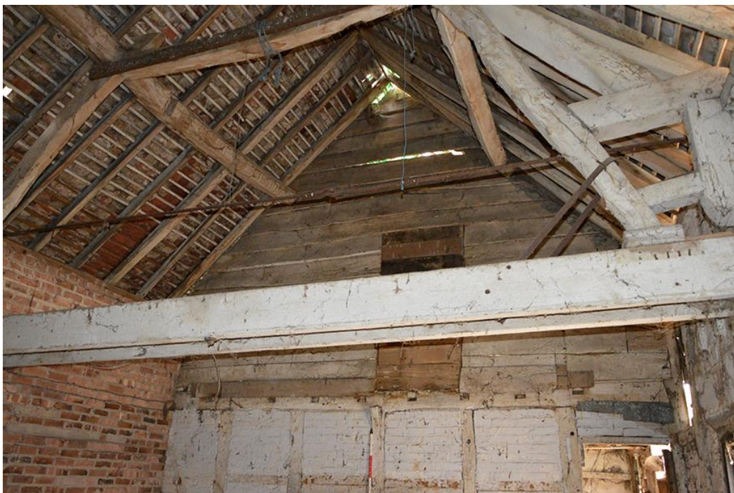
Plate 13 Central section interior, truss and east wall
