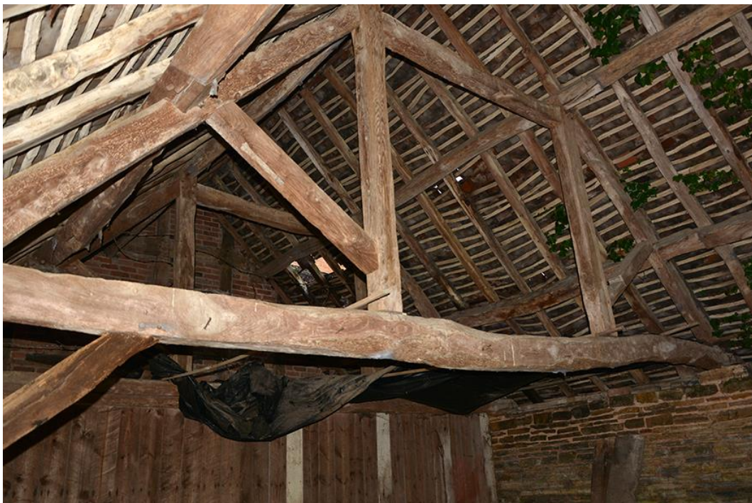
Plate 20 Cart shed, one of the trusses
