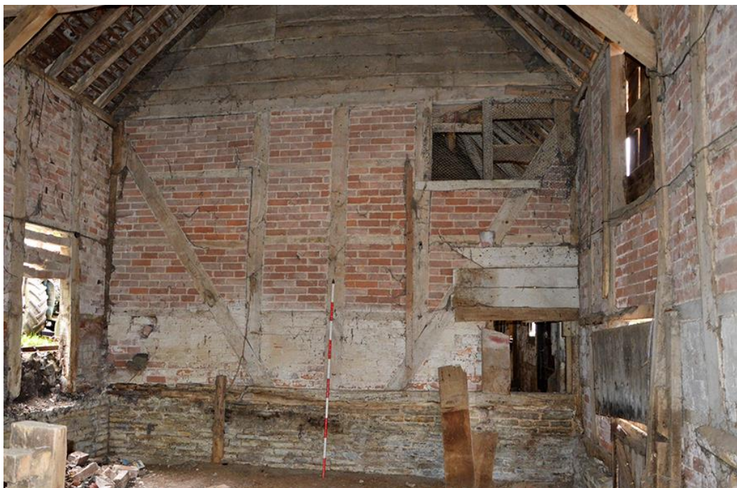
Plate 7 Western section interior, east frame
