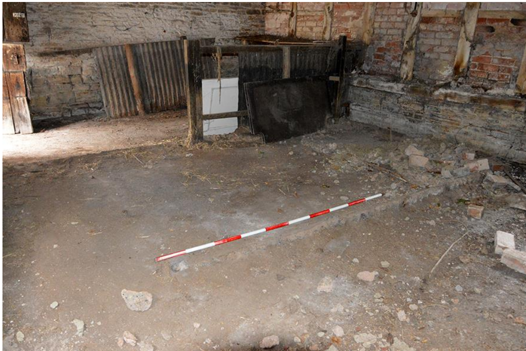
Plate 8 Western section interior, evidence of former divisions
