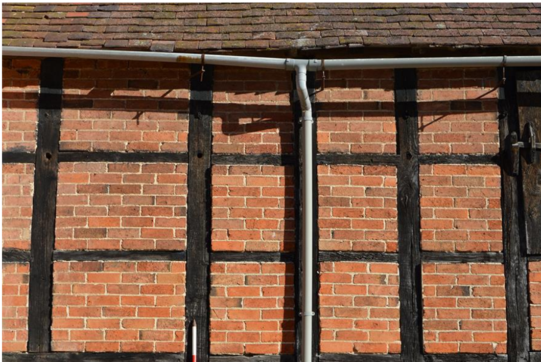
Plate 5 Peg holes from former lean-to extension
