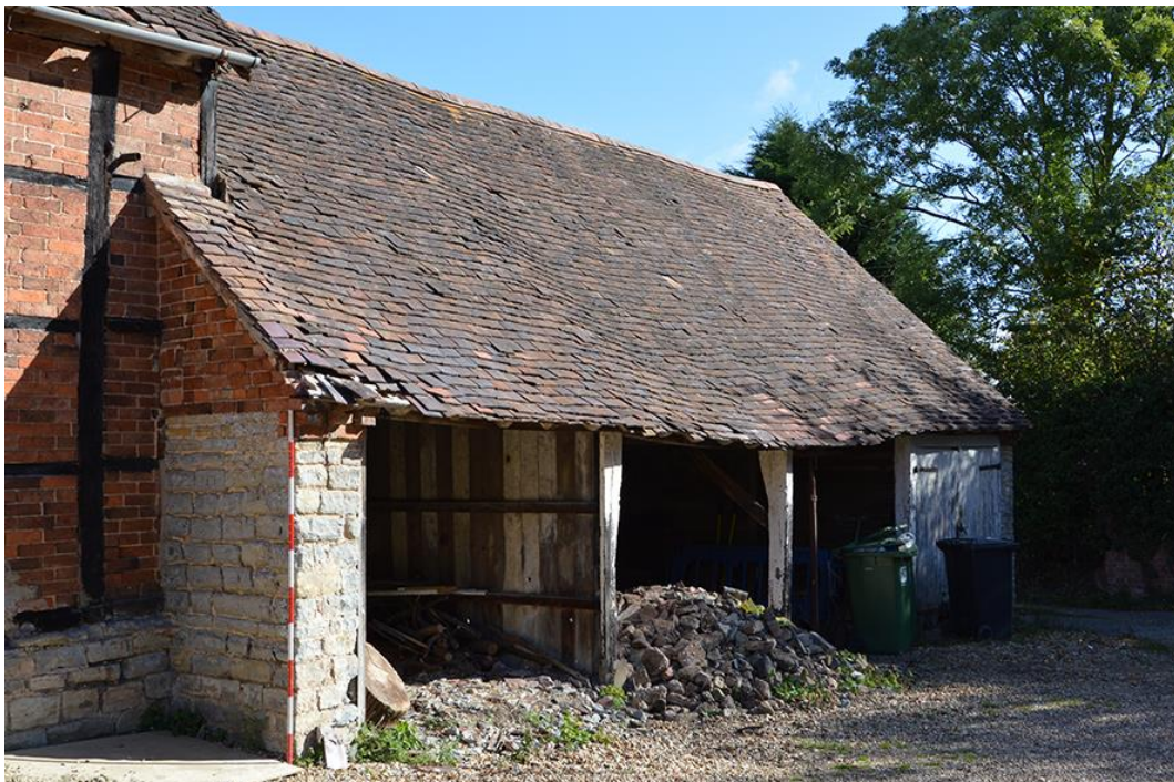
Plate 2 Cart shed from the south west
