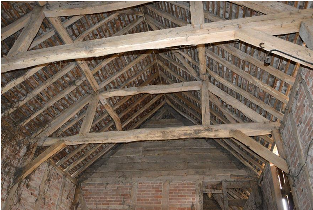
Plate 6 Western section interior, collar and post trusses
