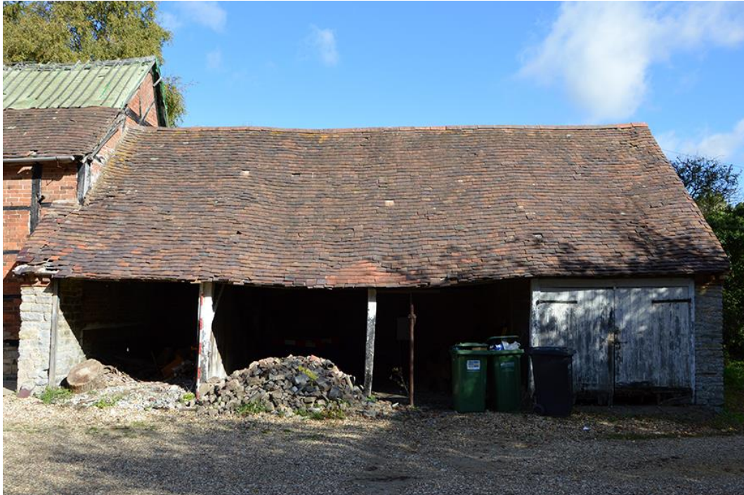
Plate 19 Cart shed, from the south
