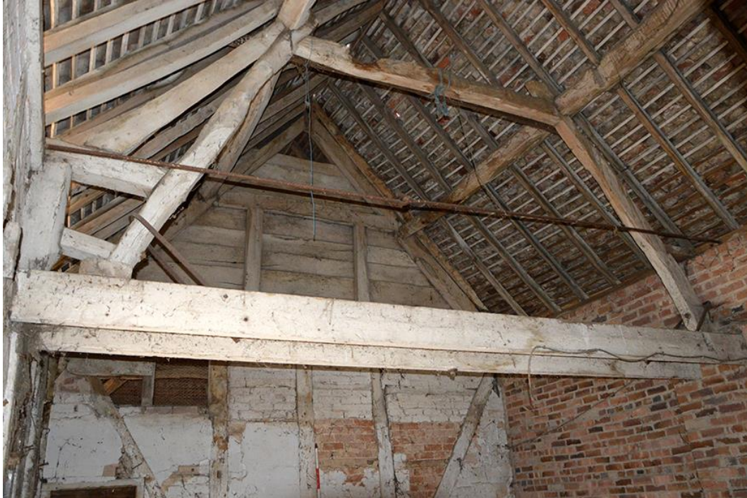
Plate 12 Central section interior, much altered cruck truss
