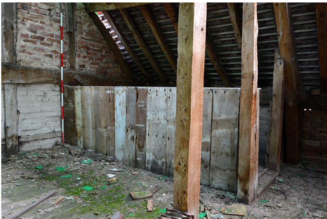
Plate 29 Timber-frame building first floor granary or apple store partition
