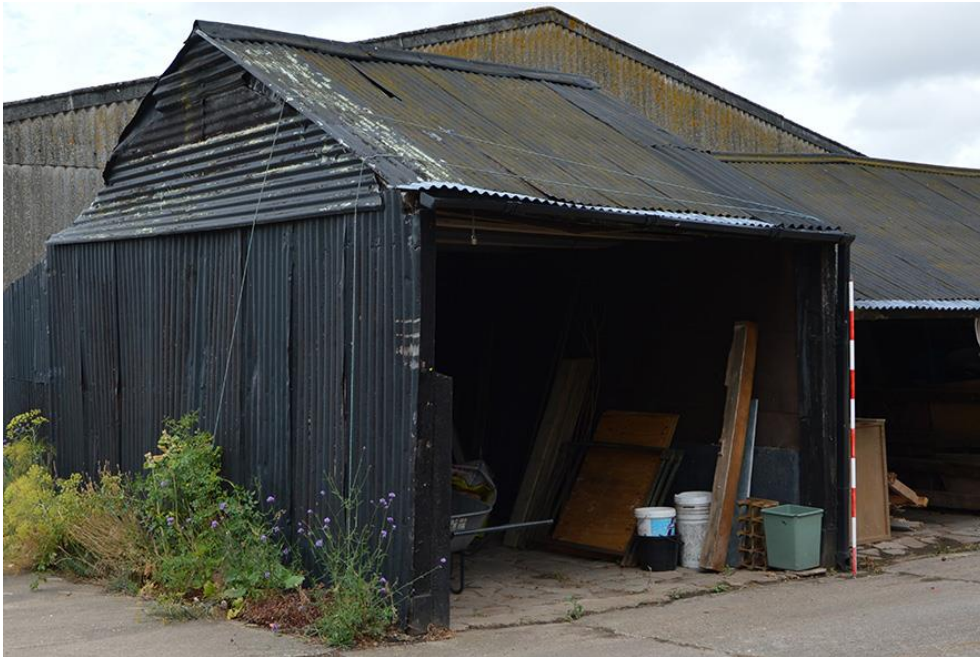
Plate 32 Area 4 of southern section of barns, showing difference of roof heights
