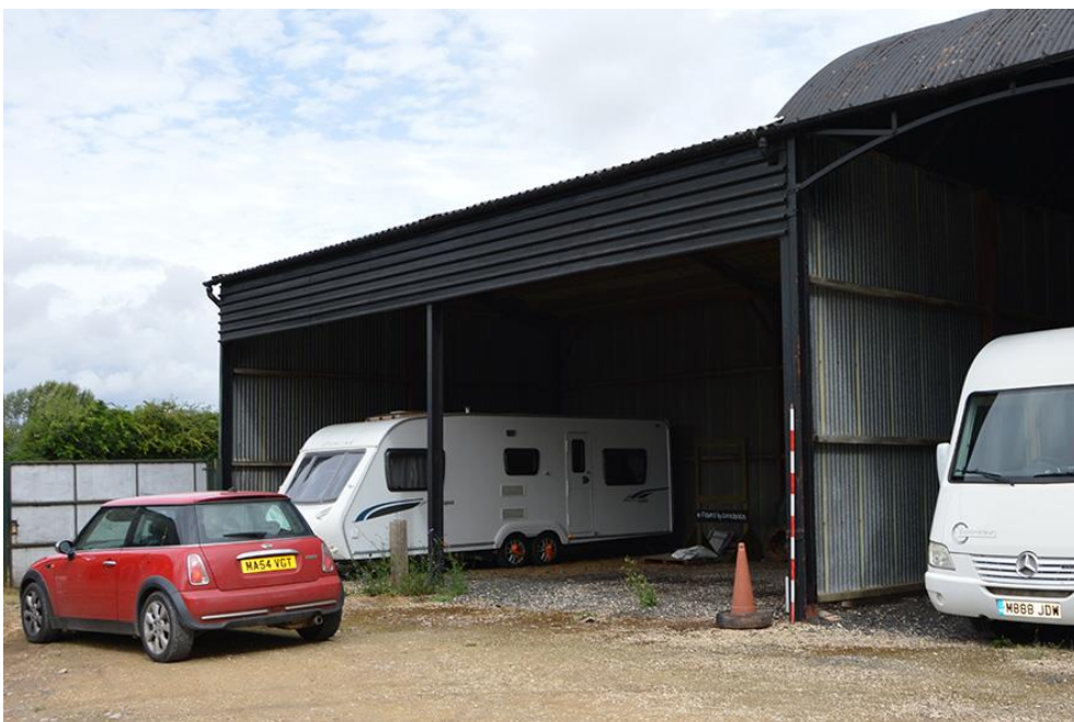
Plate 14 Late 20 th century Dutch barn from the south east
