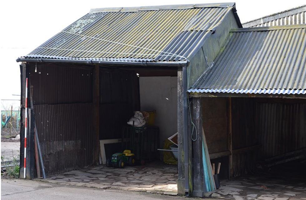
Plate 8 Southern section of barns from the west
