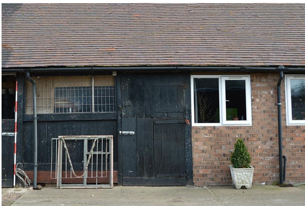
Plate 51 West elevation of workshops showing brickwork and panelling of blocking
