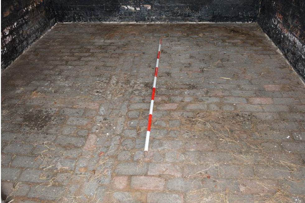
Plate 38 Brick floor with drain
