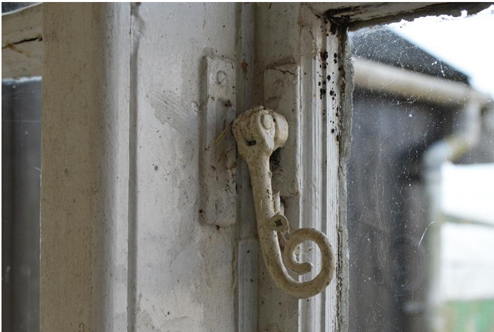
Plate 20 Spiral-ended turnbuckle catch on window of Room 1
