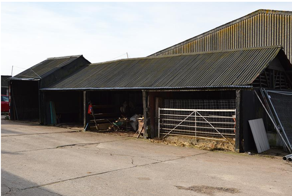
Plate 6 Barns from the north east
