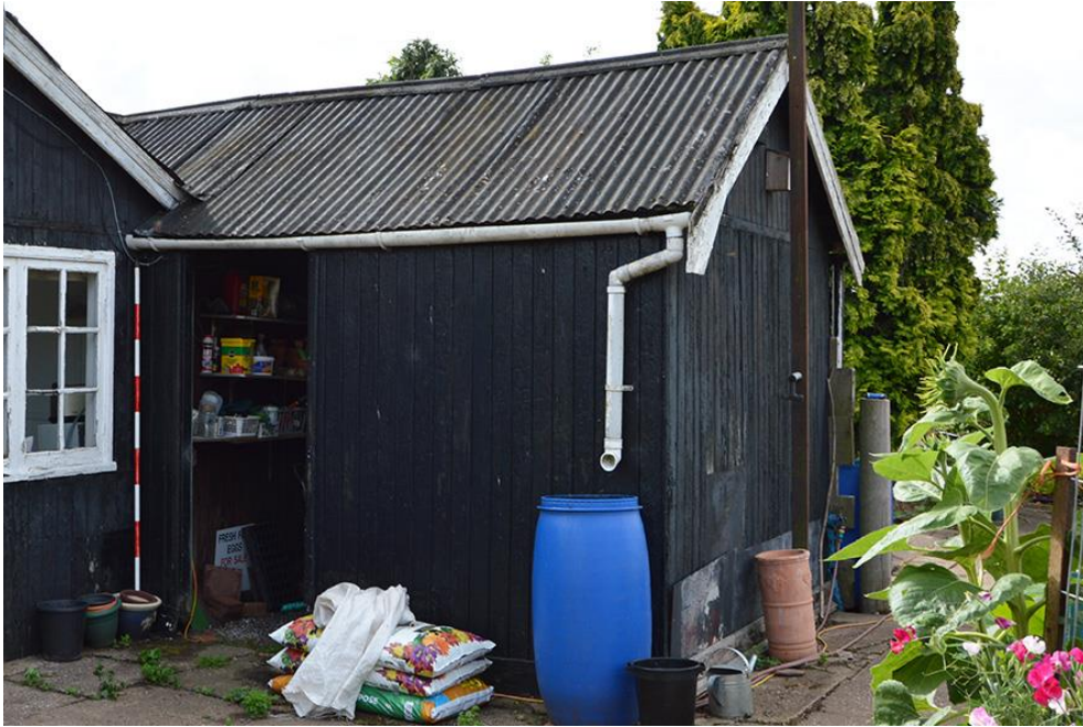
Plate 15 Exterior of external store from the north west
