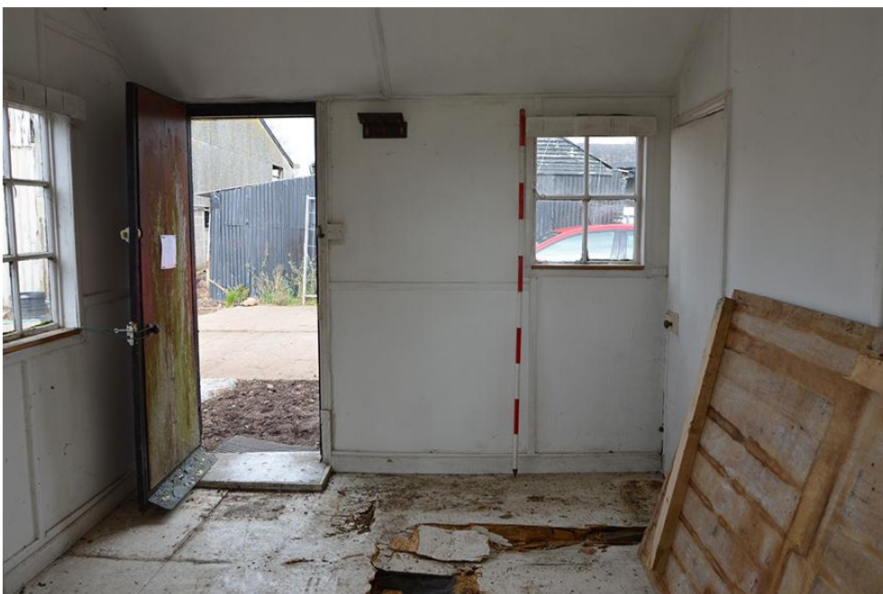
Plate 18 Interior of Room 1 from the north
