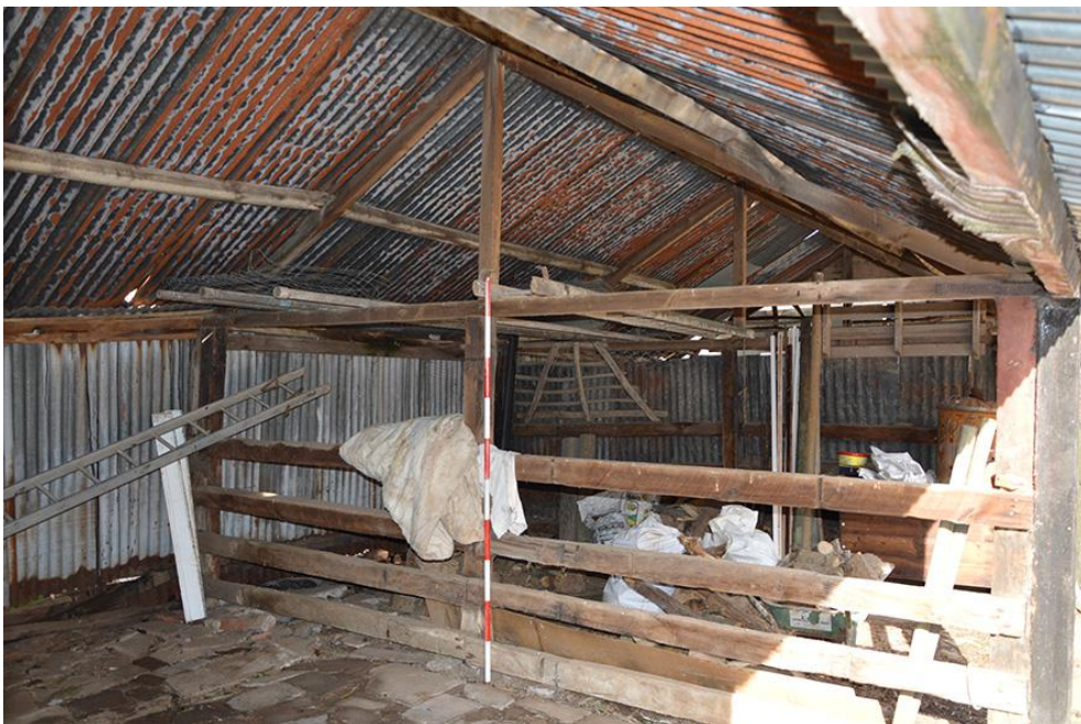
Plate 29 King-post truss within northern section of barns (Area 3)
