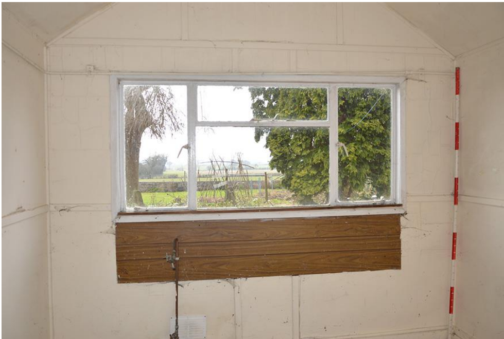
Plate 21 Interior of Room 2 from the north
