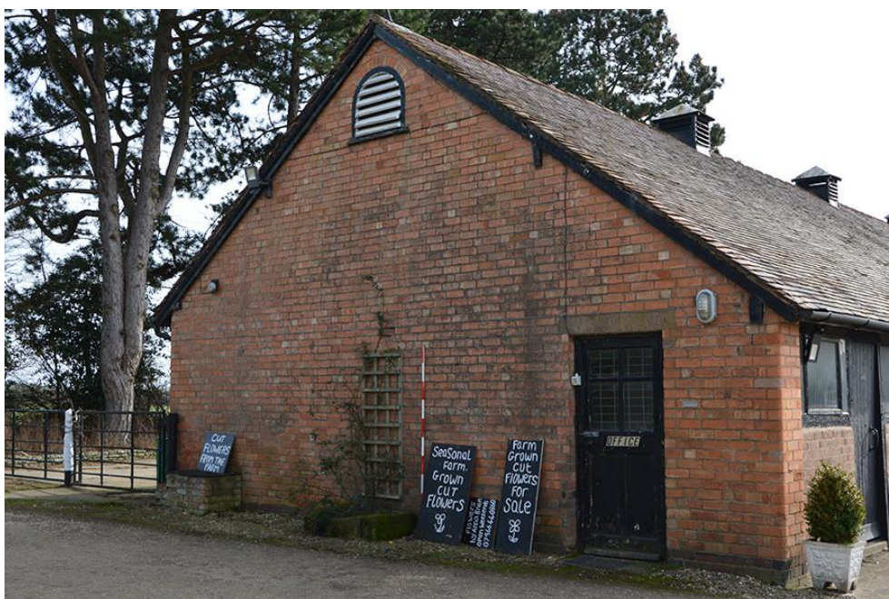
Plate 10 Northern elevation of the stables and workshops building
