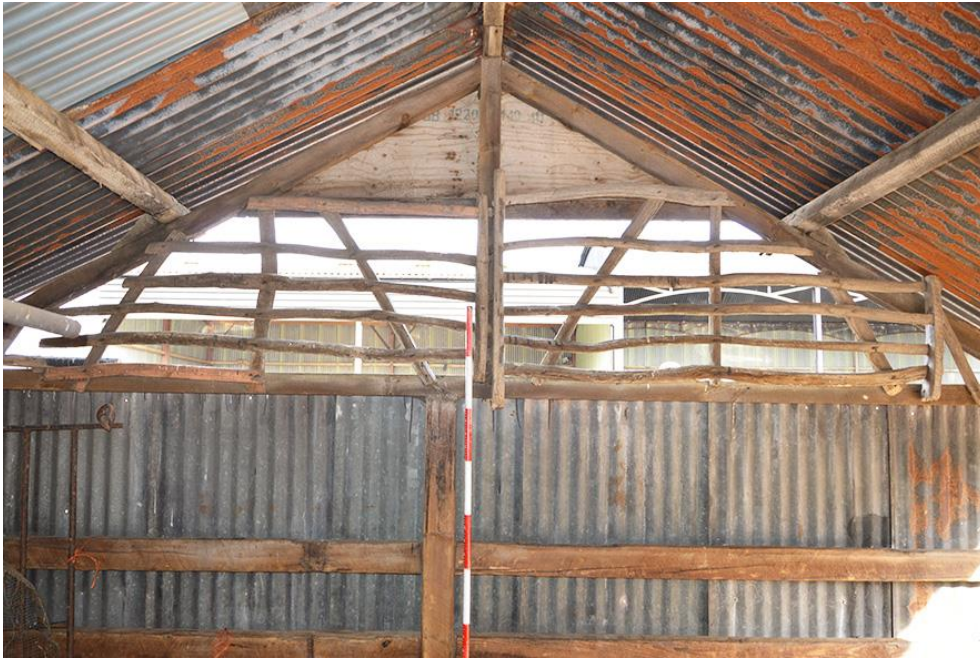
Plate 30 Staves within truss of north elevation of barns (Area 1)
