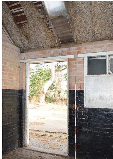
Plate 41 Interior of stables showing roof height and roof insulation
