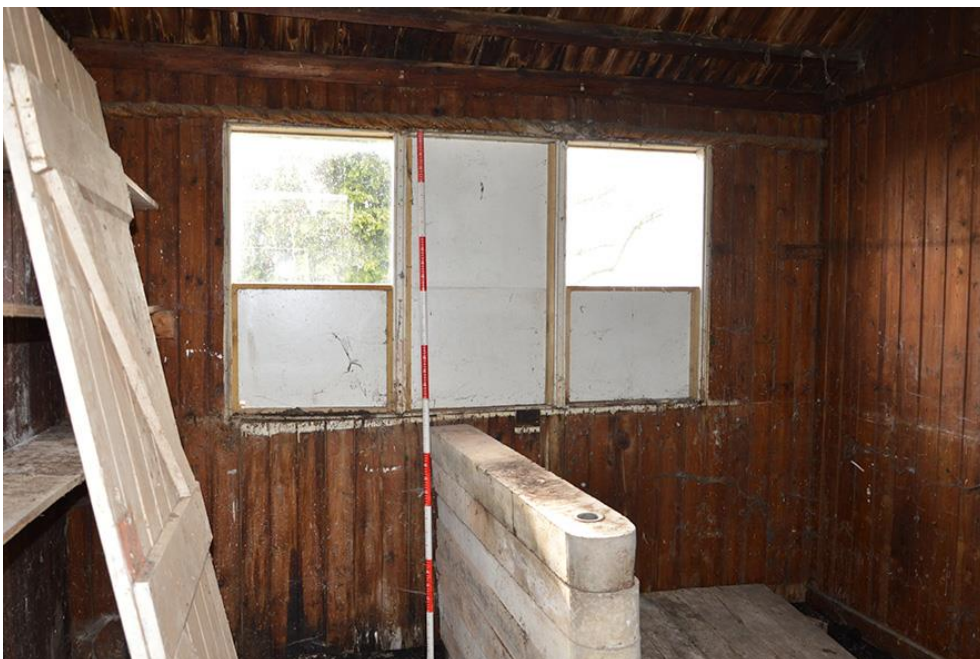
Plate 16 Interior of external store showing wooden panelling and division for stalls
