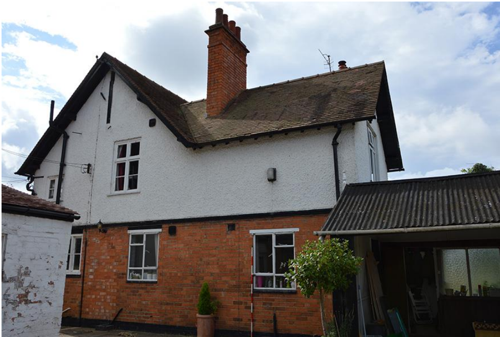
Plate 2 North elevation of Sandal Lodge house
