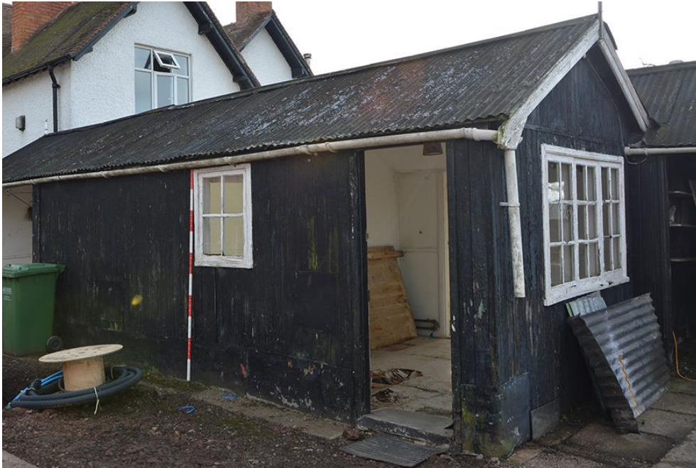
Plate 17 Exterior of Room 1 of house extension from the north west
