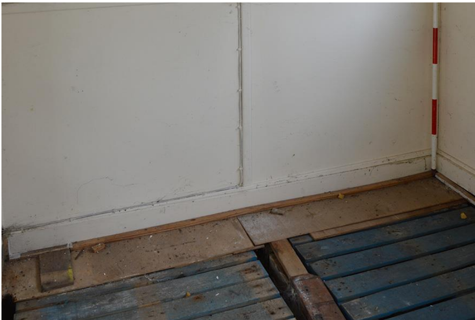
Plate 22 Part of pallet floor of Room 2
