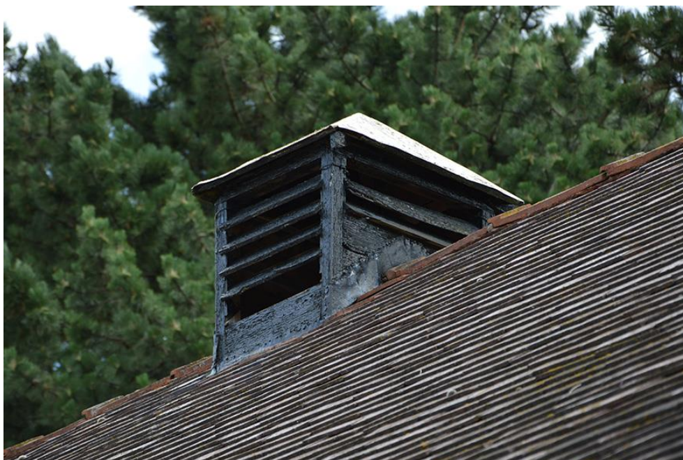
Plate 12 Cupola style ridge vent on stables and workshops building
