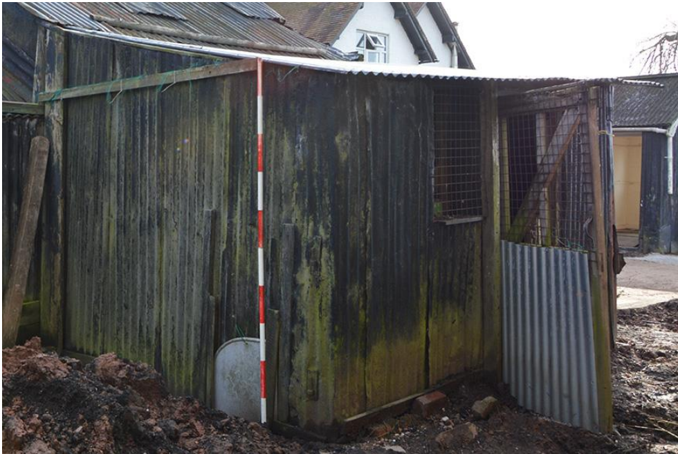
Plate 34 Exterior of Area 5 of southern section of barns
