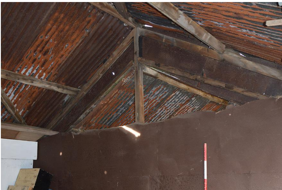
Plate 33 Trusses of Areas 3 (below) and 4 (above), note replaced king-post
