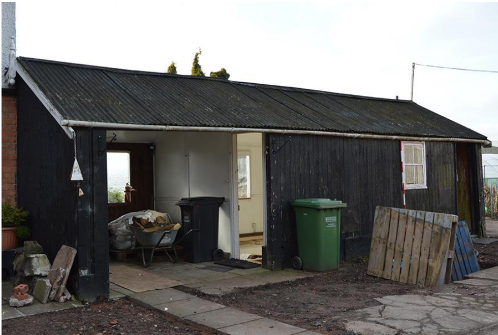
Plate 5 North elevation of house extension with porch-type entry
