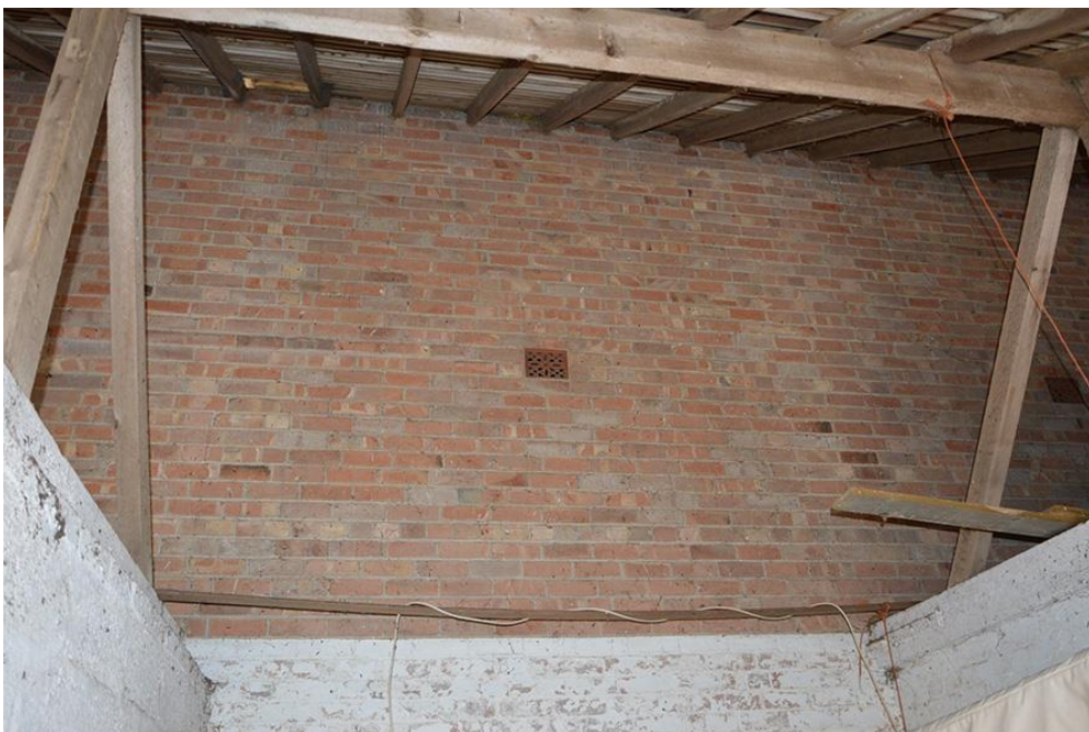
Plate 45 Ventilation brick on workshops side of the building
