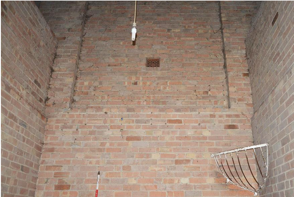
Plate 42 Stable interior showing ventilation brick
