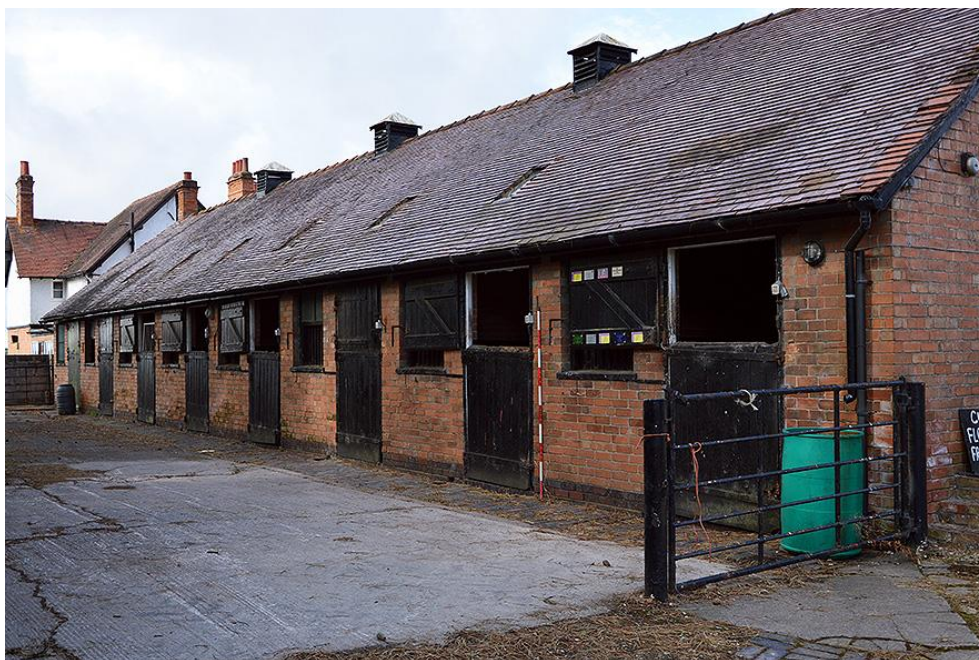
Plate 9 East elevation of stables and workshops
