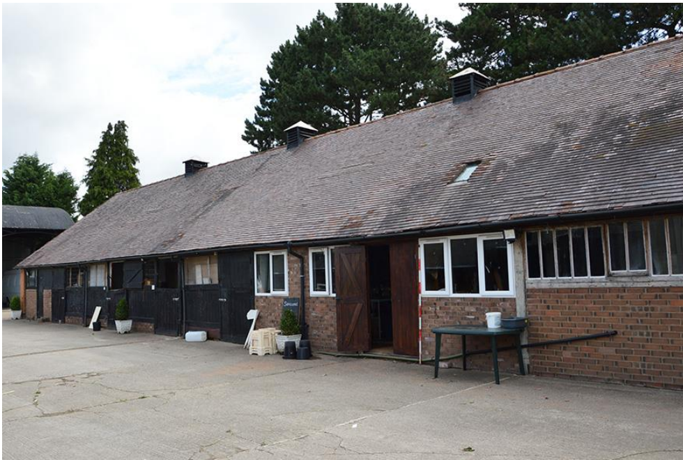
Plate 36 Exterior of workshops from south west
