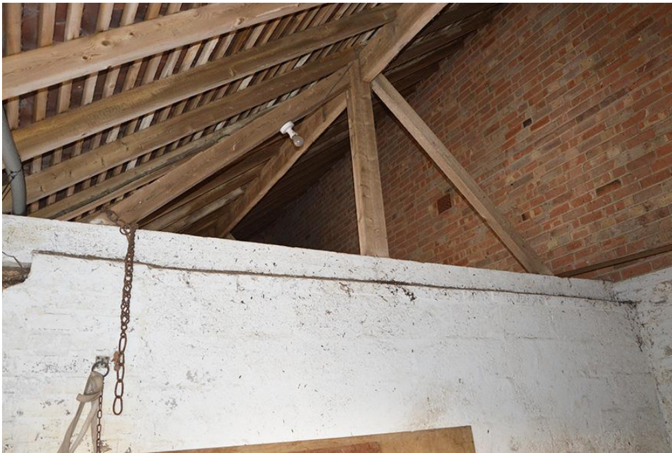
Plate 46 Interior of workshops showing roof timbers
