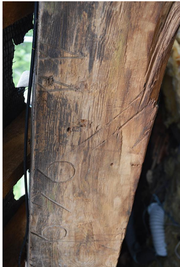
Plate 42 Timber marks on old purlins
