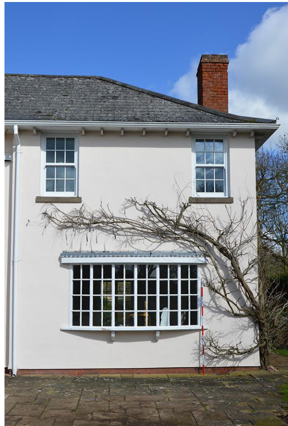
Plate 10 Bay 4 of south elevation
