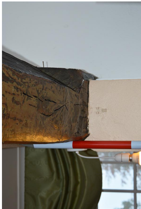
Plate 44 Inglenook bressummer with chamfer on interior
