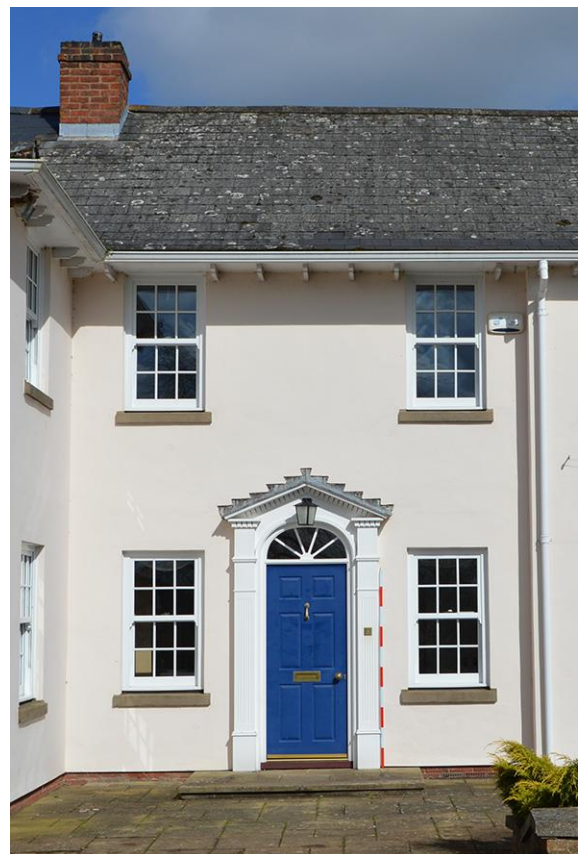
Plate 8 Bay 3 south of elevation
