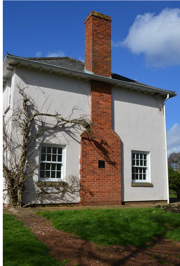
Plate 2 East elevation of Clattercut House
