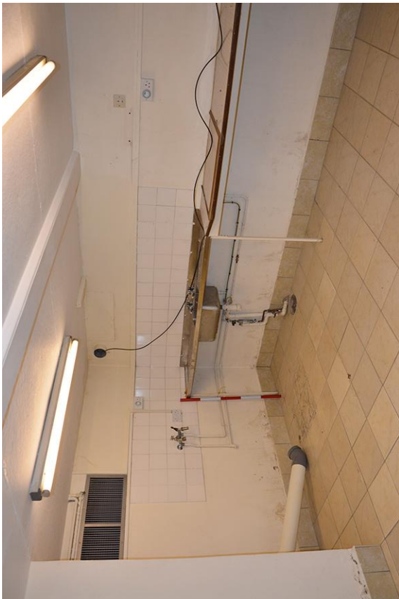
Plate 25 Southern room of basement
