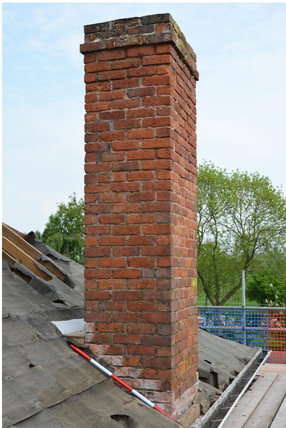
Plate 11 East elevation chimney stack
