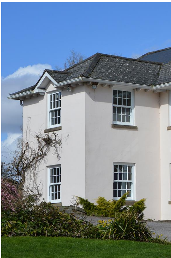
Plate 7 Bay 2 of south elevation
