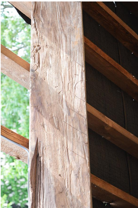
Plate 43 Timber marks on old purlins
