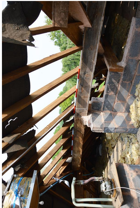
Plate 34 Old purlins in roofspace
