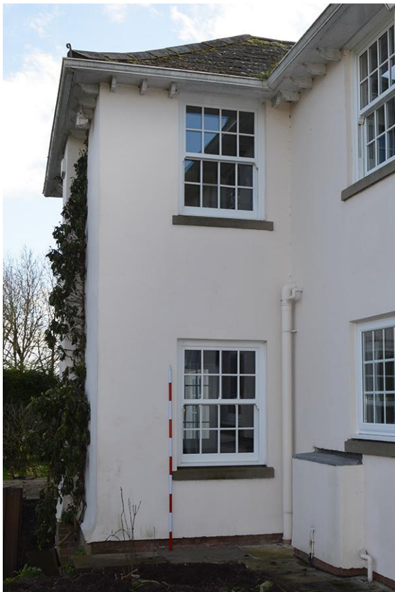
Plate 15 Bay 2 of north elevation from west
