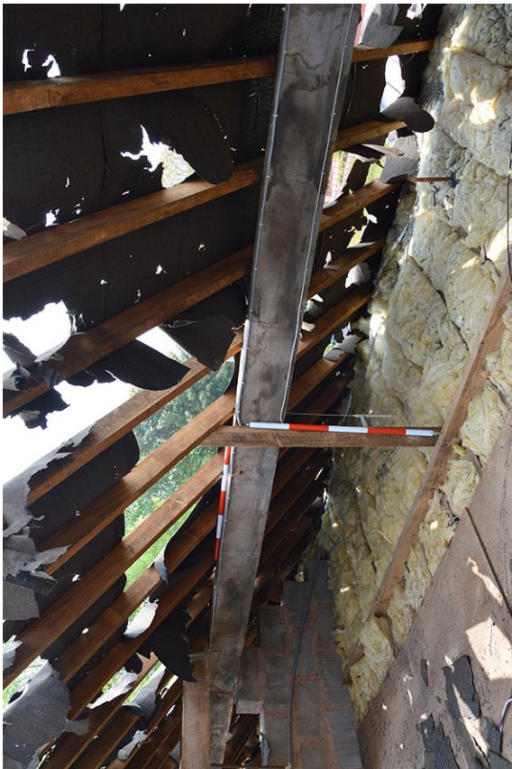
Plate 41 Old purlins in roofspace
