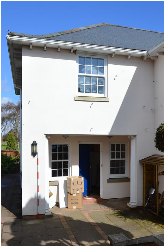
Plate 5 Bay 1 of south elevation
