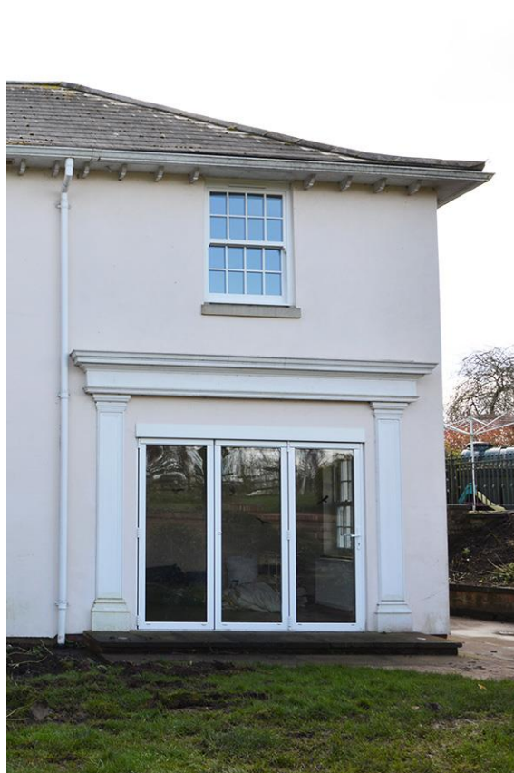
Plate 50 2010 extension from north
