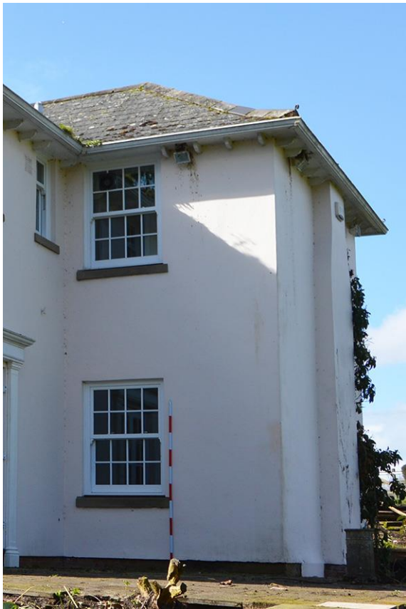
Plate 13 Bay 2 of north elevation from east
