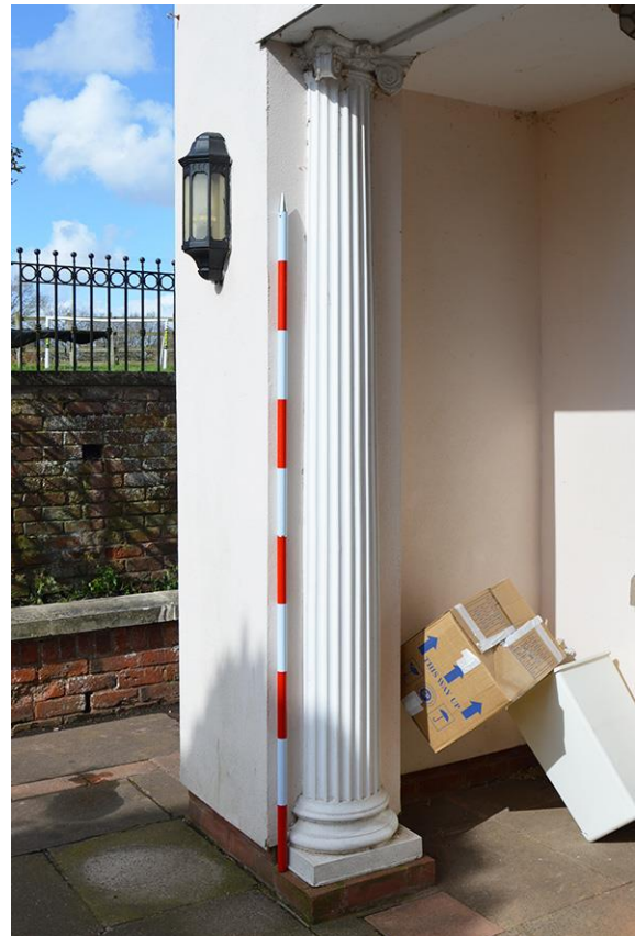
Plate 6 Bay 1 of south elevation, porch column
