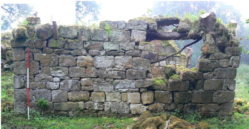
Plate 18: North face of the north wall of Building 2. The facing stones are mostly re-used from the tower
