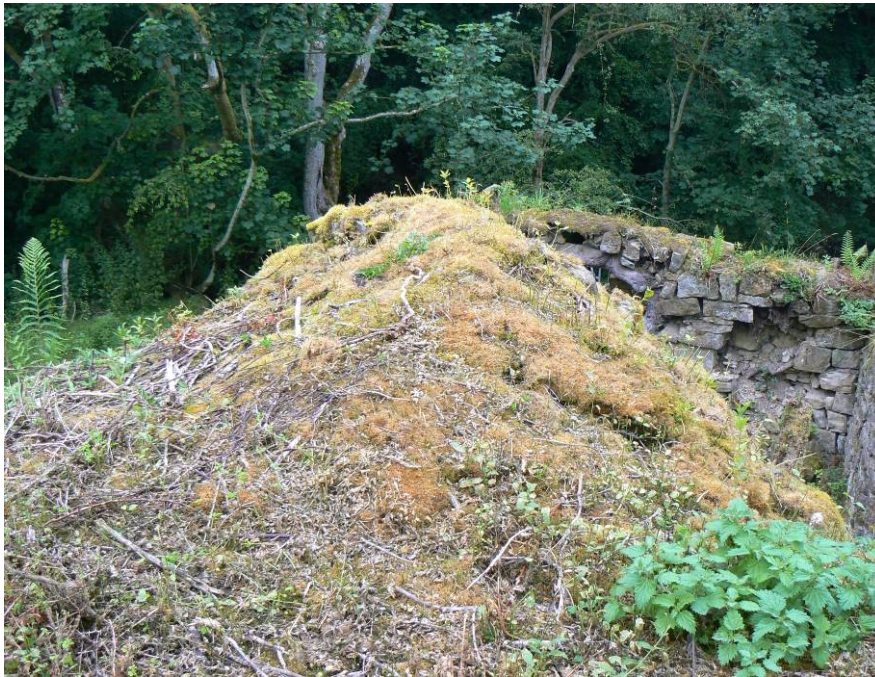
Plate 13: The northern edge of the first-floor level of Overgrass Tower
