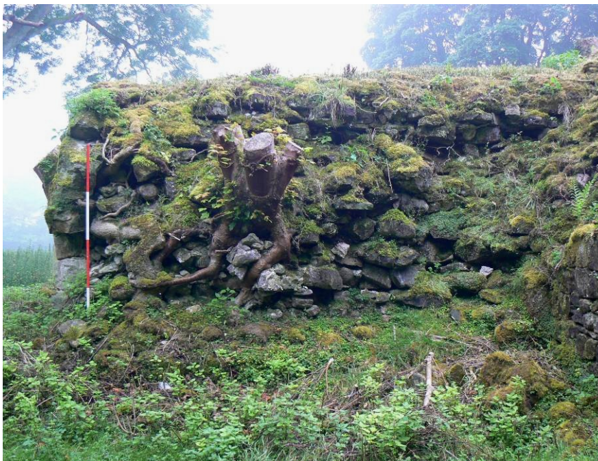
Plate 4: The eastern part of the north wall of Overgrass Tower reduced entirely to corework
