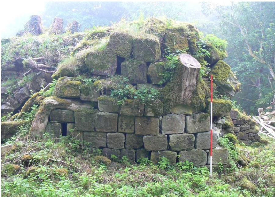
Plate 8: The surviving east face of Overgrass Tower, fallen away to both north and south. The face is leaning precariously and distorted by tree growth. The eastern loop [1.5] can be seen below the elbow in the tree root
