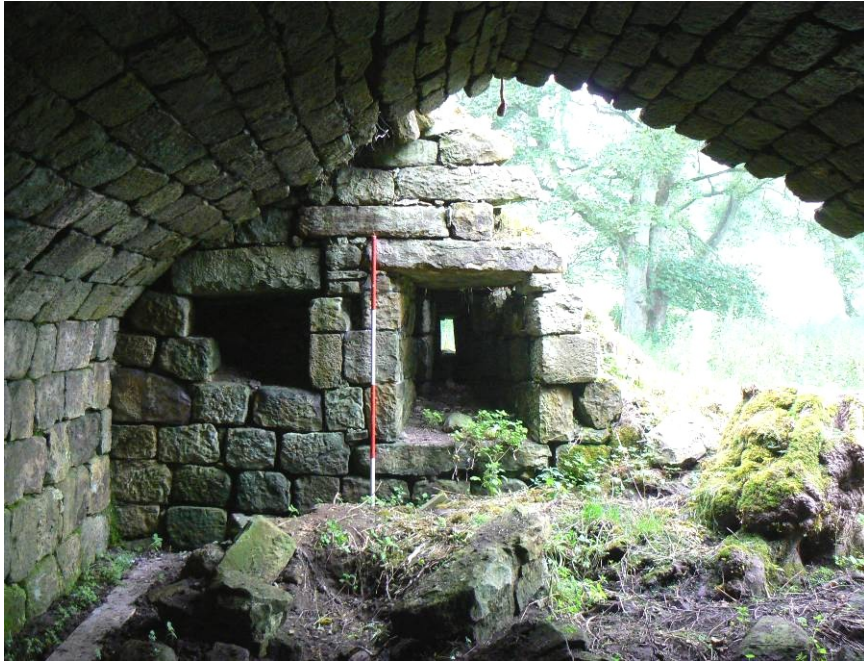
Plate 11: The basement of Overgrass Tower. Looking at the partially tumbled east wall with splayed loop [1.5] and cupboard [1.8]
