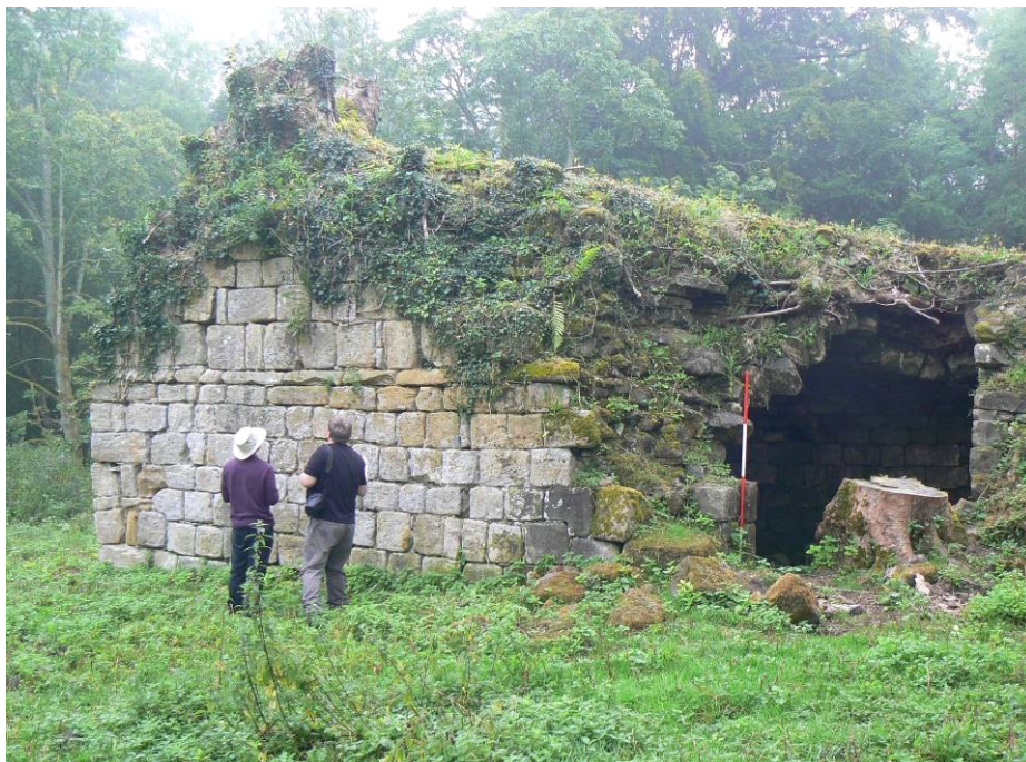
Plate 6: The tumbled south-east angle of Overgrass Tower. The scale stands against the surviving west jamb of the entrance lobby with the tumbled vault to the right
