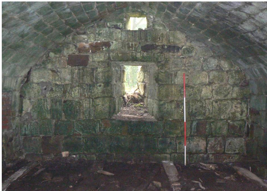
Plate12: The basement of Overgrass Tower. Looking at the west wall with splayed loop [1.4] and light [1.6] above
