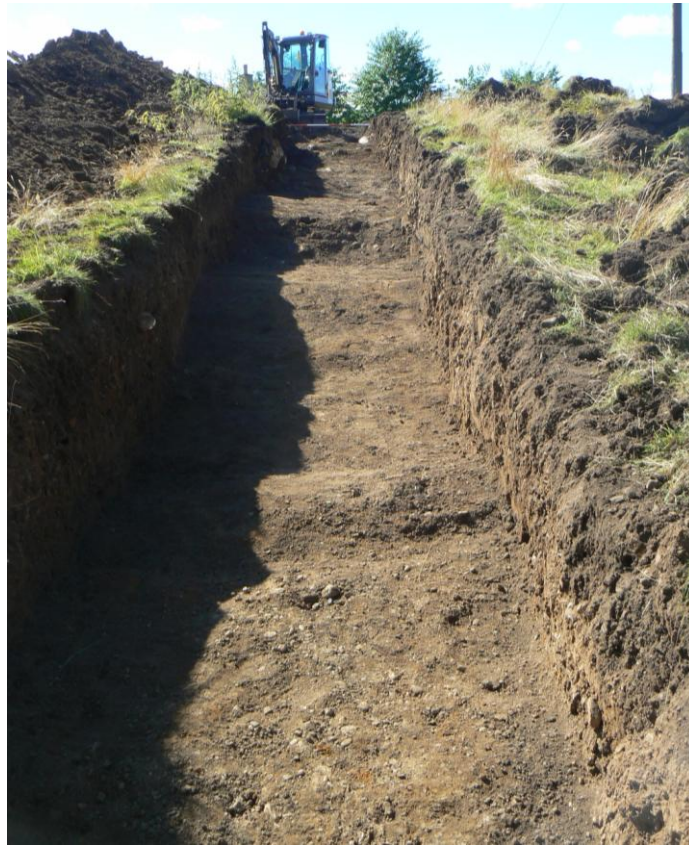
Plate 3: Trench 2, looking north-west. Gravels and sands exposed in the base
