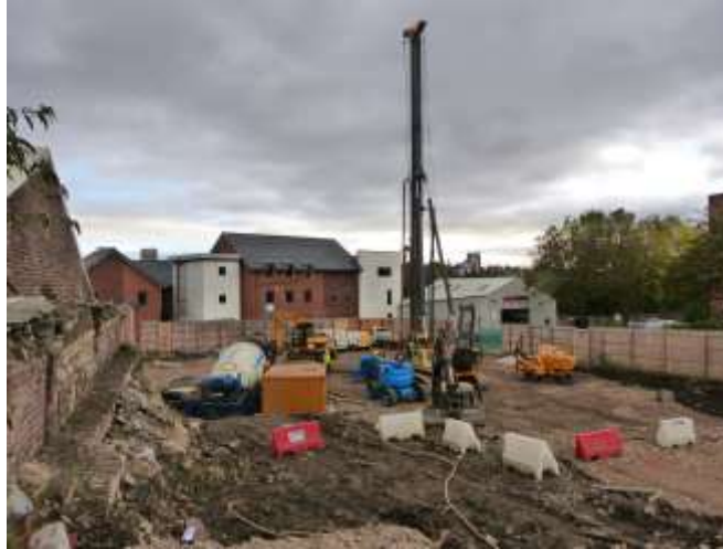
Plate 12: Looking east. Starting to pile the site.
