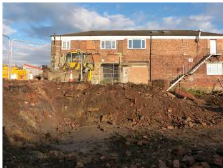
Plate 14: Looking north across the site during stripping.
