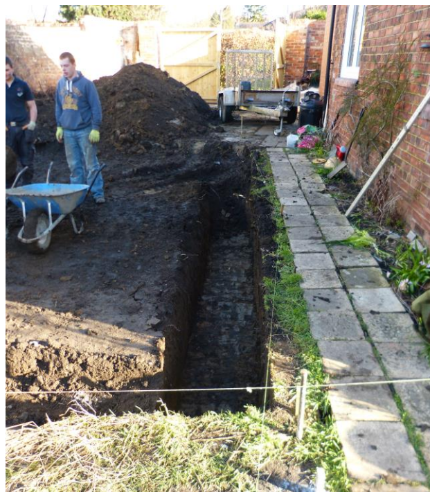
Plate 2: The east trench of the garage excavated. Looking north
