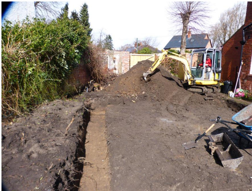
Plate 4: The west garage trench excavated. Looking north.
