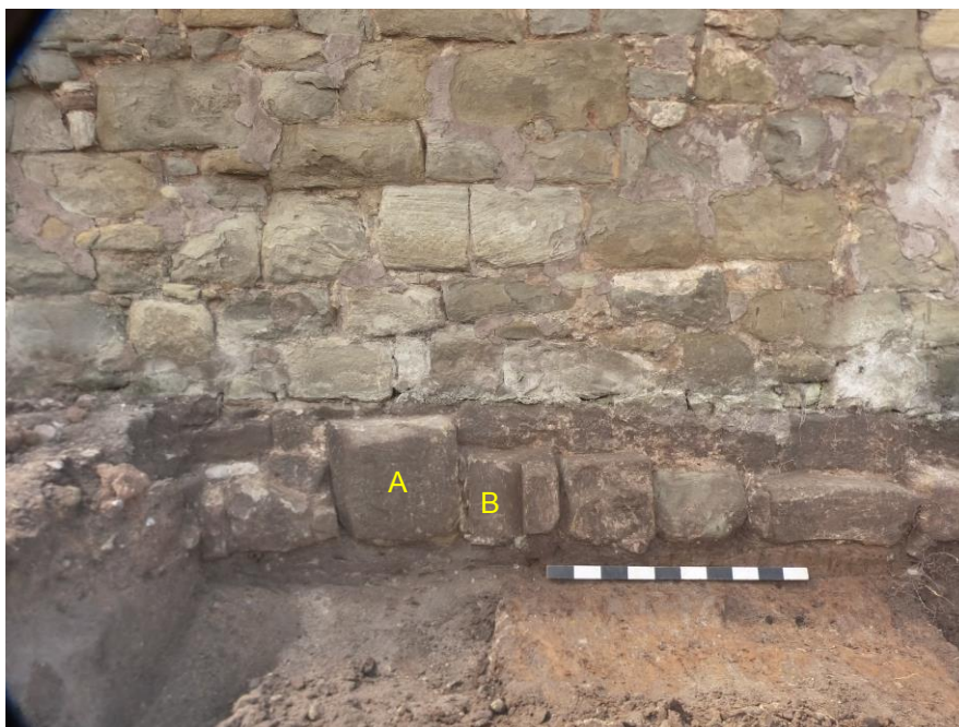
Plate 7: The offset foundation course of the vaulted building exposed in Trench A following removal of the buttress (see figure 5). A and B mark re-used stones with mouldings.
