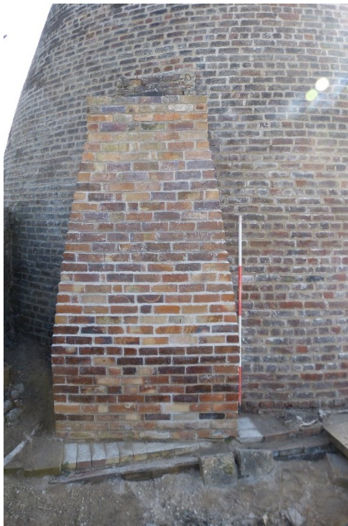
Plates 28, 29 and 30: Vents on the west face of the eastern bottle kiln. Views pre (top) and post-consolidation and rebuilding. 2m scale.
