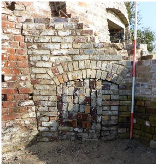
Plates 21 and 22: Post-conservation views of fireplace in north-east angle of building 8 against eastern bottle kiln (left) and from same point west across building 8. 2m scale.
