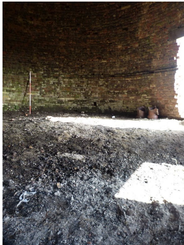
Plate 33: Post clearance view of the eastern bottle kiln. Looking north. 2m scale.
