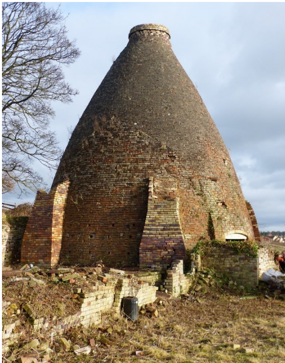
Plates 11 and 12: Eastern bottle kiln from the west. Remains of drying floor (7) and building (8) in front. Pre (left) and post conservation. 2m scale.
