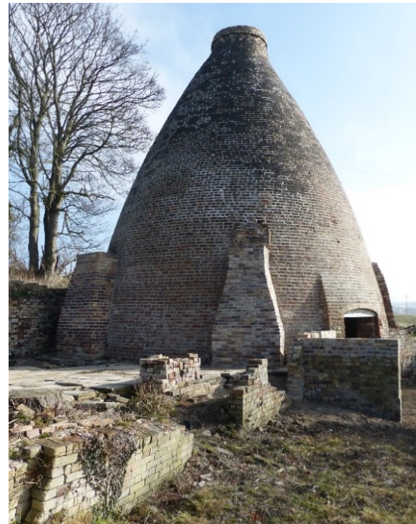
Plates 11 and 12: Eastern bottle kiln from the west. Remains of drying floor (7) and building (8) in front. Pre (left) and post conservation. 2m scale.
