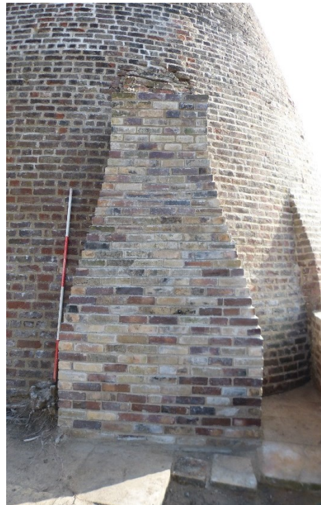
Plates 28, 29 and 30: Vents on the west face of the eastern bottle kiln. Views pre (top) and post-consolidation and rebuilding. 2m scale.
