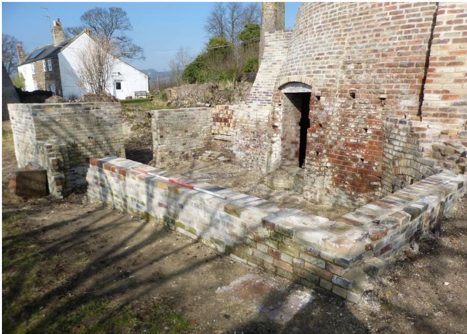
Plates 17 and 18: Looking north-west across remains of building 8 to the south of the eastern bottle kiln. Pre (top) and post conservation. 2m scale.
