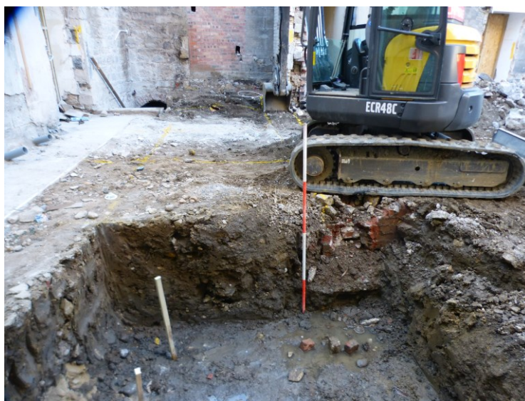
Plate 3: Foundation pit for the library room within the courtyard. Looking south.
