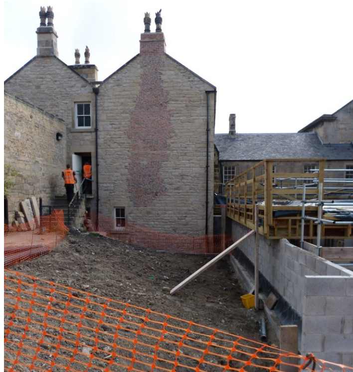
Plate 11: Retaining wall constructed. Looking east.
