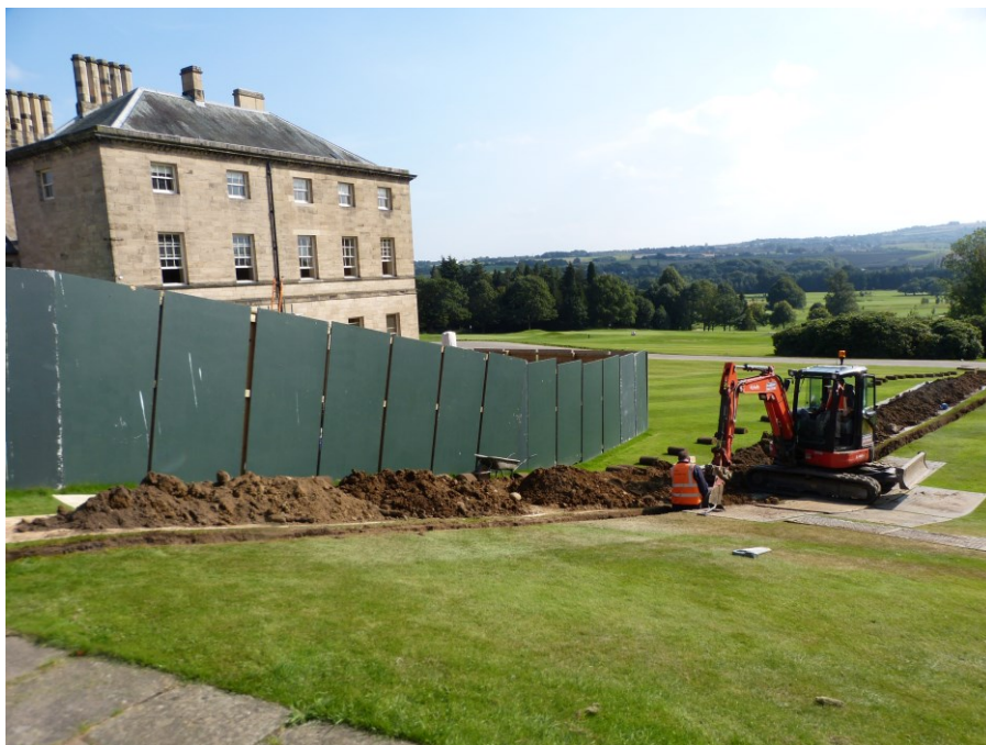
Plate 14: Excavation of service trench (5). Looking south-east across Close House
