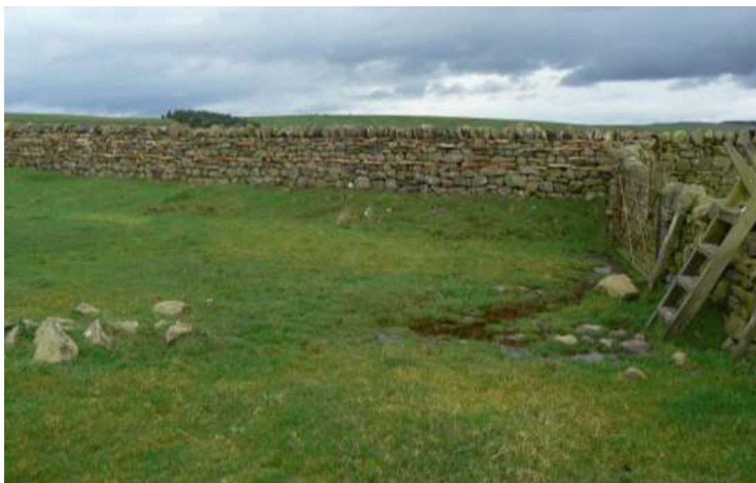
Plate 20: The same view as plate 19 following rebuilding of the dry-stone wall.
