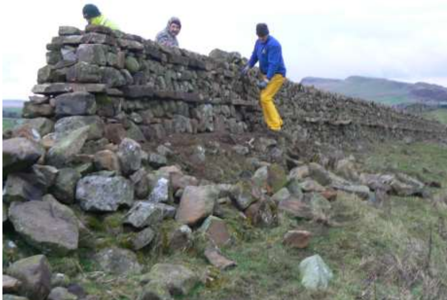
Plate 8: Rebuilding the dry-stone wall west of Great Chesters.
