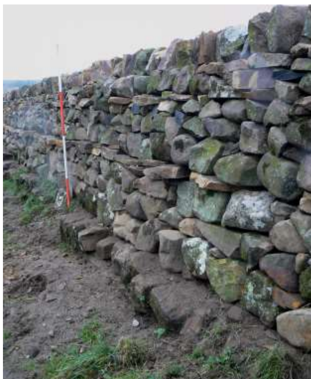
Plate 35: East of Great Chesters. Roman fabric at base of north face of rebuilt dry-stone wall. 2m scale.
