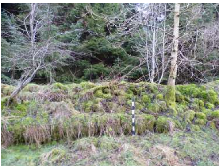
Plate 16: The Wall in Area 6 before clearance of trees and saplings. The Wall face is exposed but obscured by vegetation.
