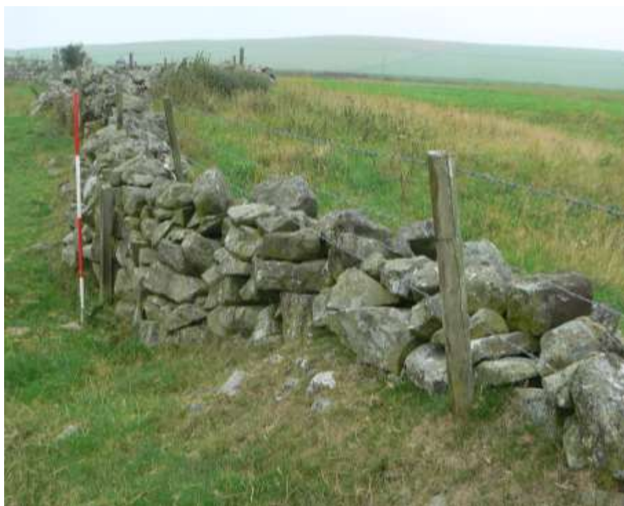
Plate 2: East of Great Chesters. Dry-stone field wall overlying the remains of the Roman Wall in 2013. Looking east in the area of Turret 42b. Scale is 2m long.
