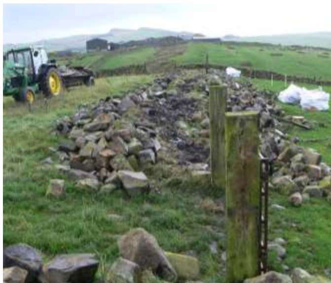
Plate 11: Dismantling the dry-stone wall over the Wall mound. West of Great Chesters, looking east.
