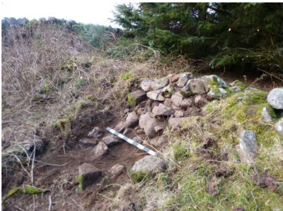
Plate 1: Slot A in Area 1, looking north-west. The tumbled dry-stone wall remains a prominent feature. There is little evidence for the Roman Wall. 1m scale.
