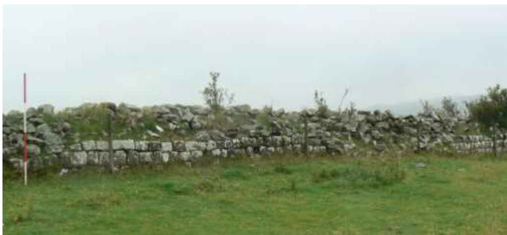
Plate 6: The same length of in-situ Roman Wall below tumbled field wall east of Great Chesters Farm in 2012. 2m scale.
