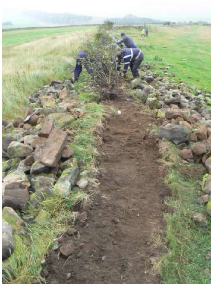
Plate 4: East of Great Chesters. Dry-stone wall over Wall mound cleared away. Removing self-seeded saplings and shrubs. Looking east.
