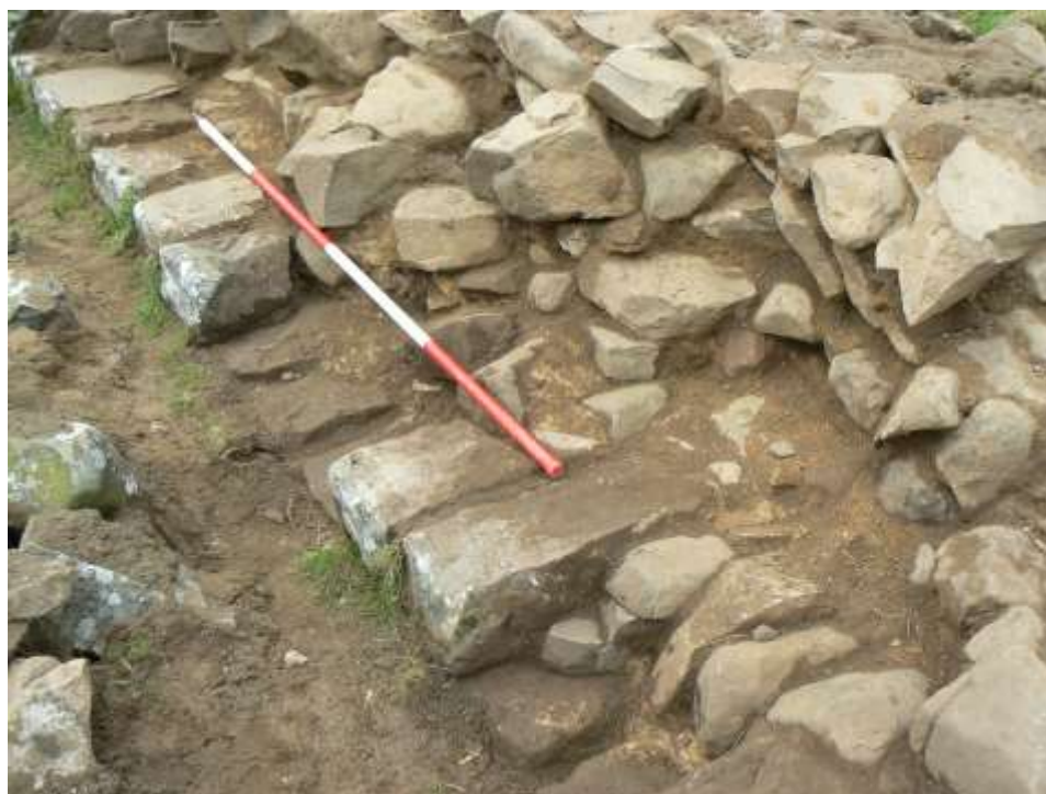
Plate 10: Roman facing stones and core east of Great Chesters. Original friable sandy-brown mortar still bonds the facing stones and core. 2m scale.
