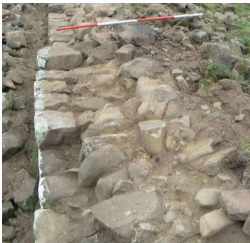
Plate 26: Same area as plate 25, looking west. Facing stones and core bonded with a sandy brown mortar. 2m scale.
