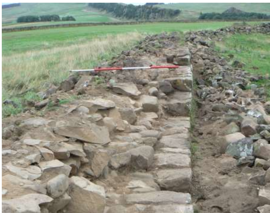
Plate 24: East of Great Chesters. South face of the Wall and core exposed following removal of dry-stone wall and cleaning. Looking east. 2m scale.
