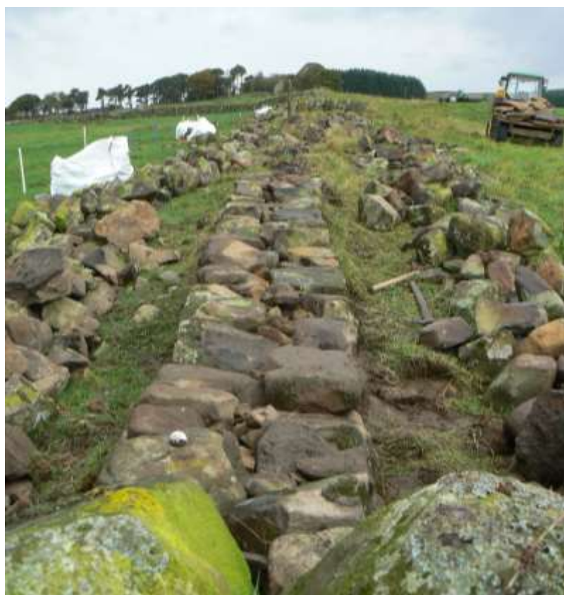
Plate 32: West of Great Chesters looking west. Base of new dry-stone wall.
