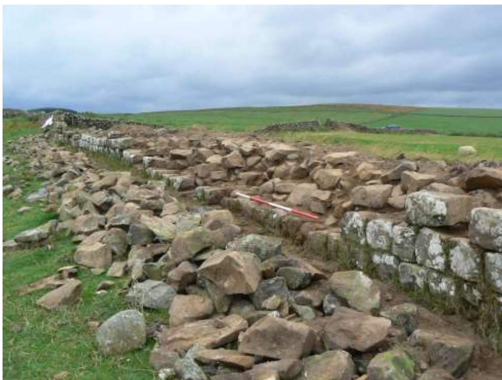
Plate 28: Similar view to plate 27 following removal of overlying dry-stone wall. The exposed fabric is all in-situ Roman. 2m scale.
