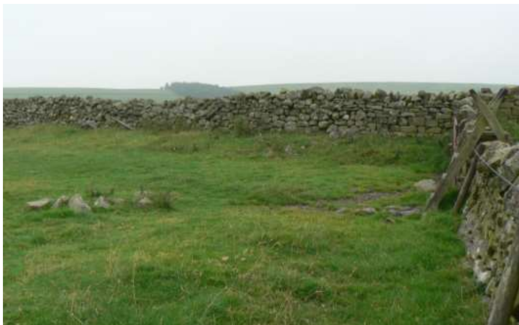
Plate 19: Slumped dry-stone wall over remains of Hadrian's Wall. East of Great Chesters in 2013. Looking north-west.
