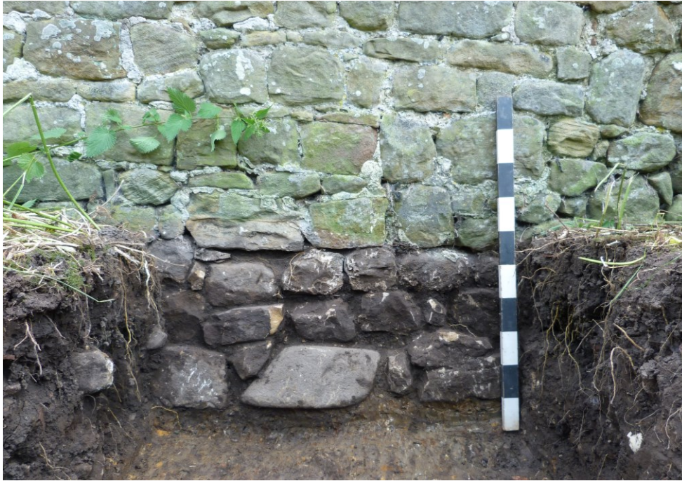
Plate 15: Trench 6. Foundations of the north wall of building C. 1m scale.
