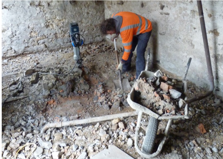
Plate 19: Reducing the level of the floor surface in Outbuilding 2.
