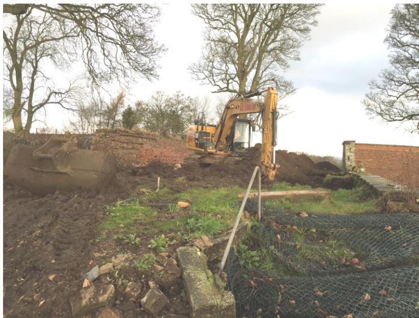
Plate 3: Beginning excavation for the swimming pool. Looking north.
