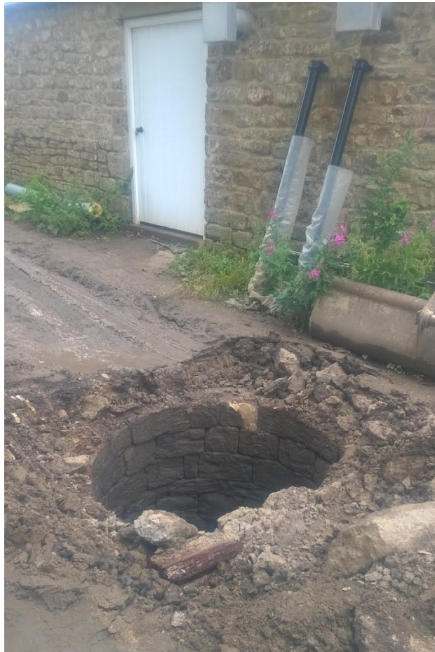
Plate 2: the capping removed. Boiler house to rear.
