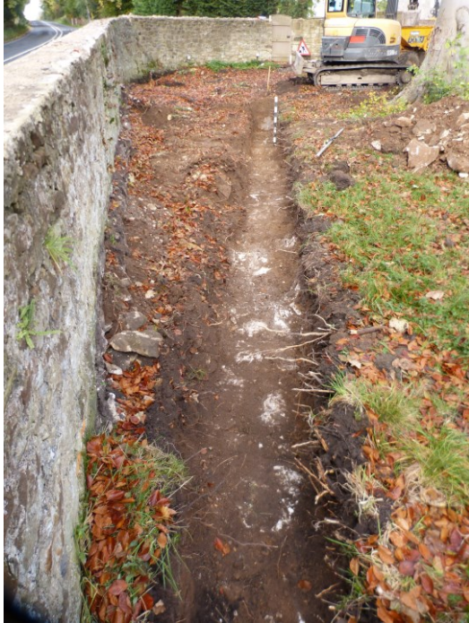
Plates 7 and 8: Excavation of the trench for the new roadside wall. Sandstone bedrock is exposed in the base along its whole length. Plate 7 looking west, plate 8, looking east.
