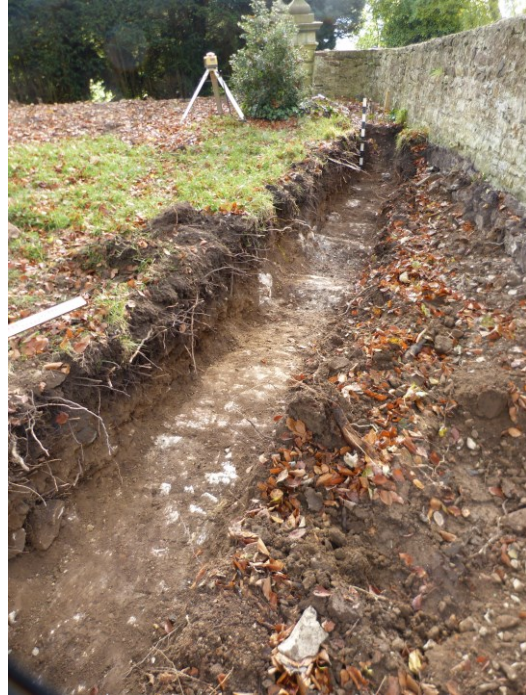
Plates 7 and 8: Excavation of the trench for the new roadside wall. Sandstone bedrock is exposed in the base along its whole length. Plate 7 looking west, plate 8, looking east.
