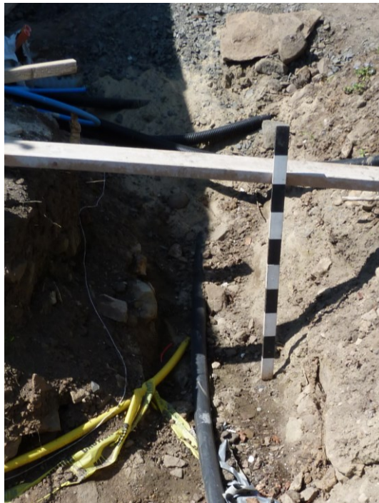
Plate 3: Trench for spur. Looking west.
