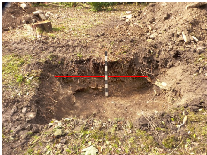
Plate 13: Test pit 3 in the footprint of the ramp. Red line indicates level of sandstone bedrock. 1m scale.
