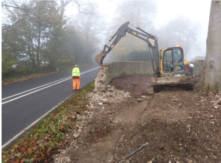
Plate 10: Subsequent demolition of the roadside wall. Looking west.
