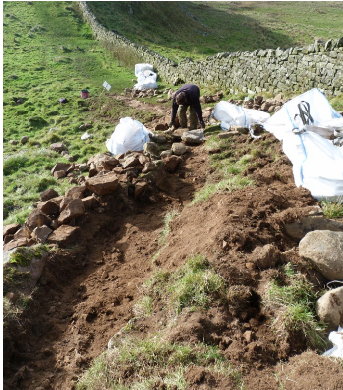
Plate 8: The slot excavated. Same area as shown in plate 7.
