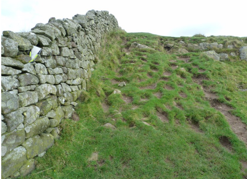
Plate 12: Area B, looking east. Prior to remedial works.
