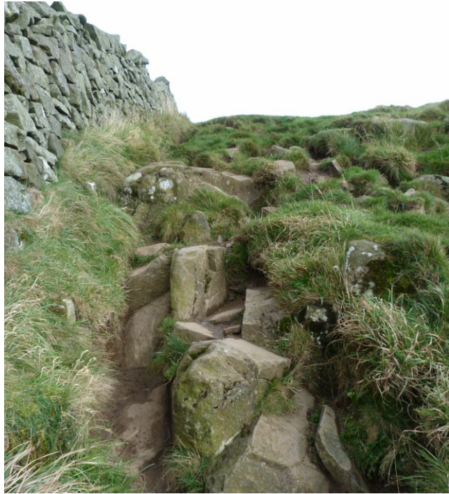
Plate 4: Area of deep erosion with exposed bedrock Area A, towards the top of the path, looking east.
