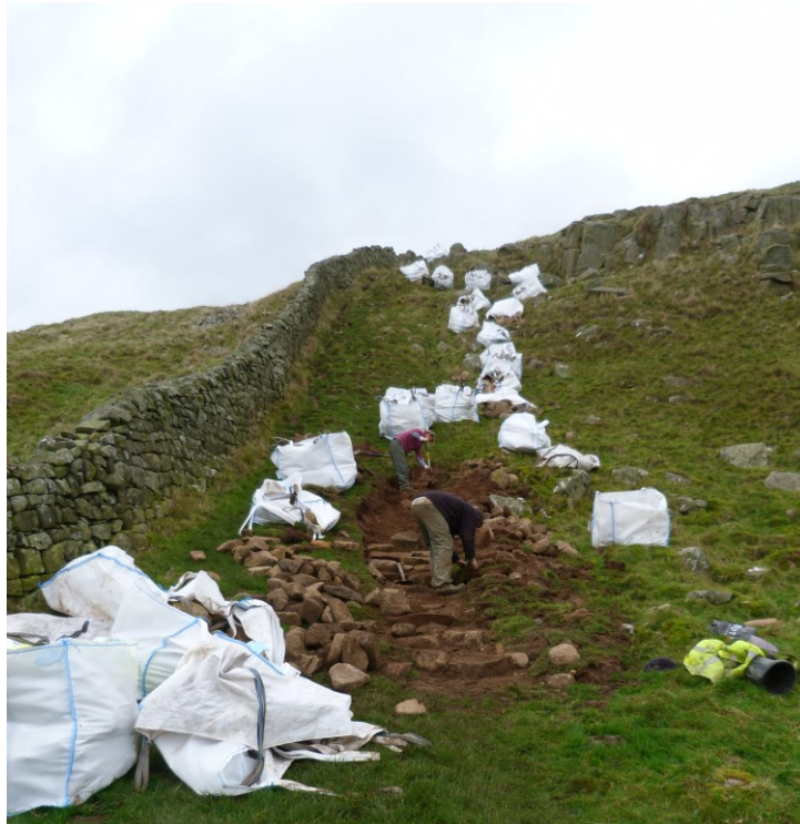
Plate 6: Looking east. Constructing steps at the western end of Area A.
