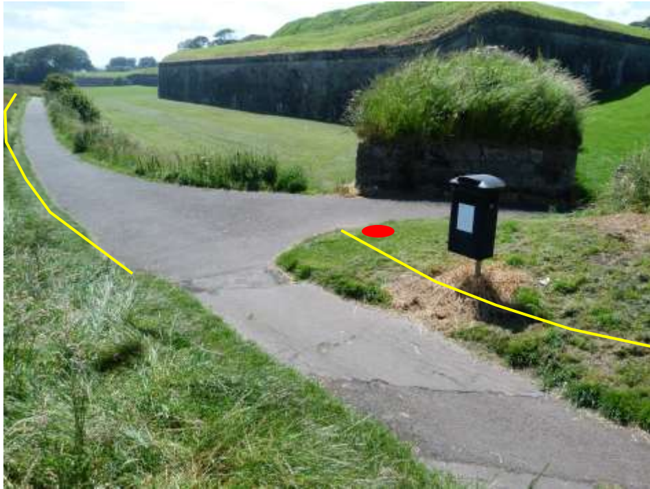
Plate G: Existing footpath. Located on figure 6. Looking south-west towards Batardeau and Brass Bastion beyond. Yellow lines show intended widening. Red disk location of finger post and pole.
