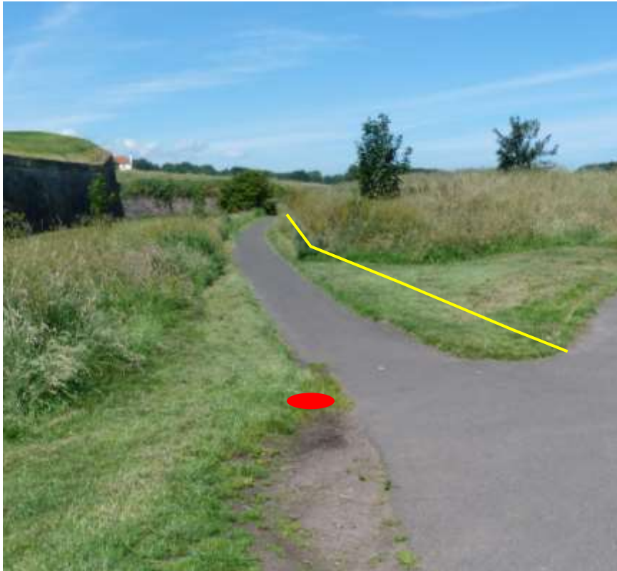
Plate 33: Existing footpath. Looking north. Brass Bastion and Batardeau to left. Yellow line shows intended widening. Red disk location of way marker.
