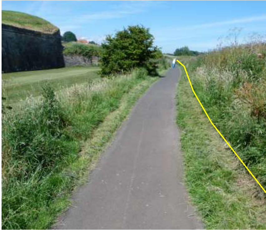
Plate 31: Before works. Looking north. Brass Bastion to left. Yellow line shows intended widening.
