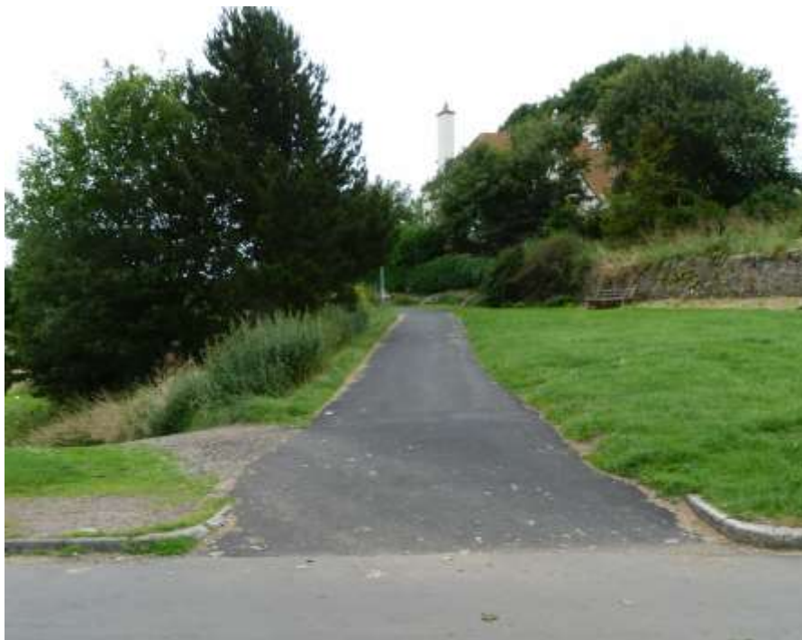
Plate 16. After works. Same view as Plate 15.
