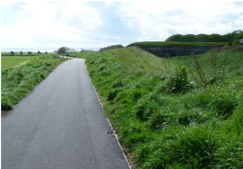
Plate 24: After works. Same view as plate 23.
