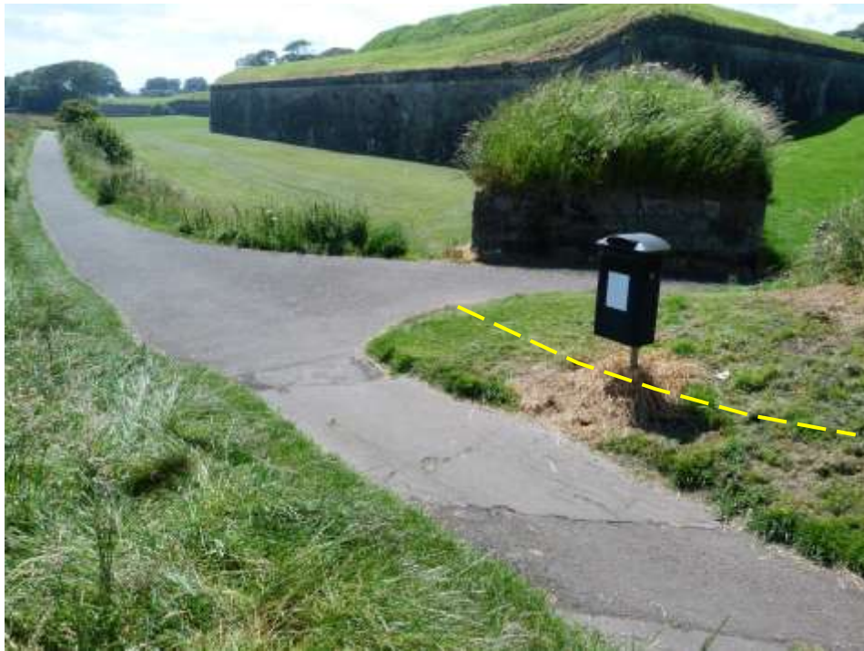
Plate 27: Before works. Looking south-west towards Batardeau and Brass Bastion beyond. Hatched yellow line shows intended widening.
