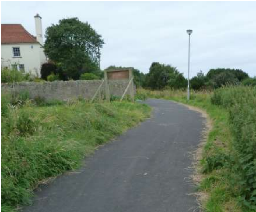
Plate 20: After works. Same view as plate 19.
