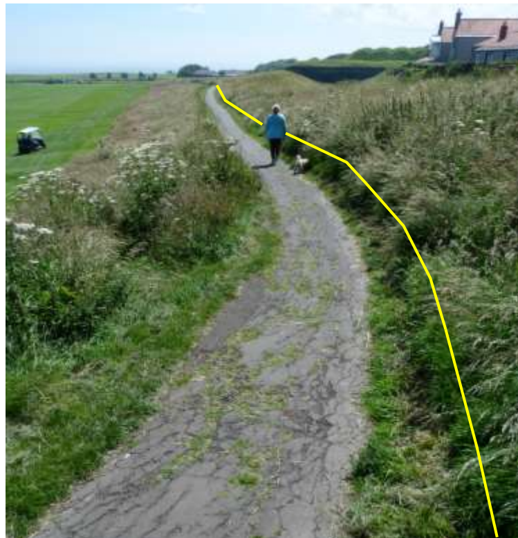
Plate D: Existing footpath. Located on figure 5. Looking south alongside Edwardian ditch (to right). Extent of counterscarp can be seen in distance. Yellow line shows intended widening.
