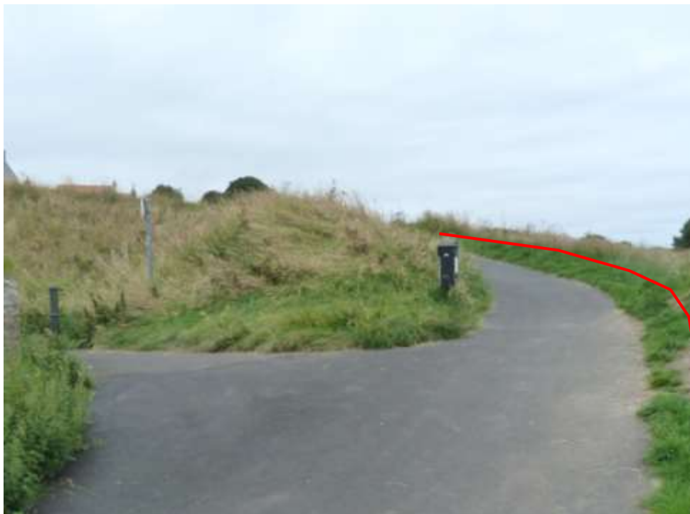
Plate 30: After works. Same as plate 29. Red line shows actual line of widening to avoid counterscarp bank of Brass Bastion.
