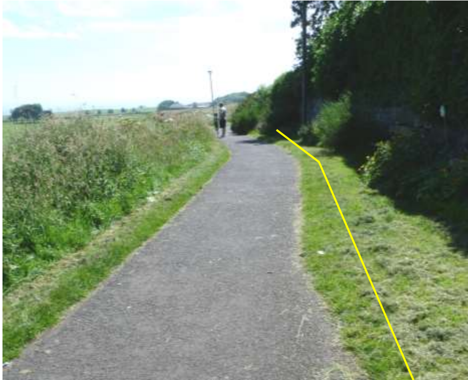
Plate 17: Before works. Looking south alongside Fields House. Yellow line shows intended widening.
