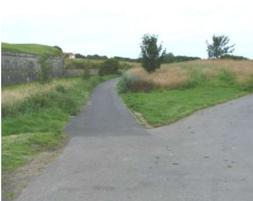
Plate 34: After works. Same as plate 33.
