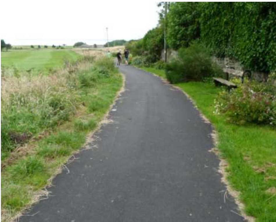
Plate 18: After works. Same view as plate 17.
