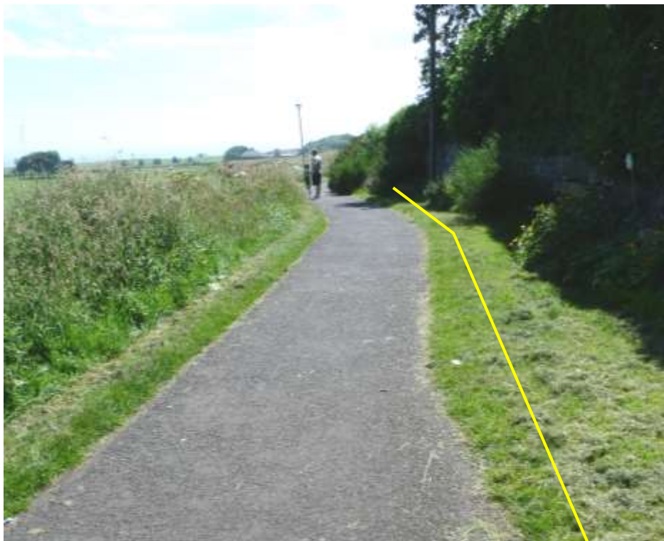
Plate B: Existing footpath. Located on figure 5. Looking south alongside Fields House. Yellow line shows intended widening.
