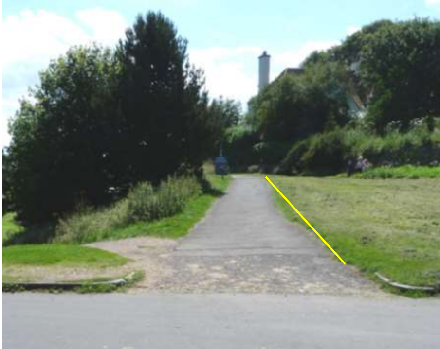
Plate 15: Before works. Looking south across the eastward extension of Northumberland Avenue. Fields House behind trees. Yellow line shows intended widening.
