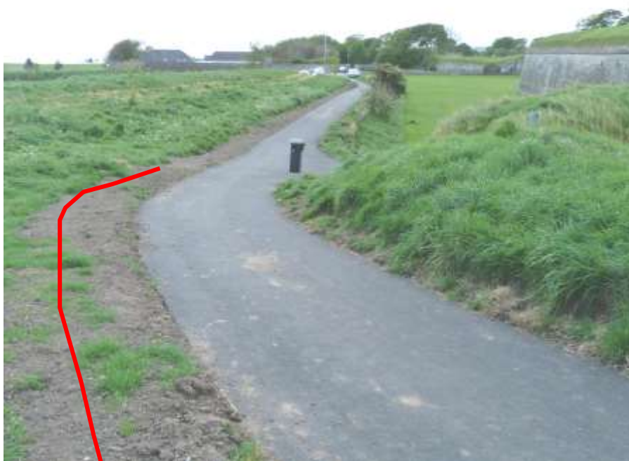
Plate 26: After works. Same as figure 25. Red line shows actual widening of footpath to avoid impact on counterscarp bank of Brass Bastion to right.
