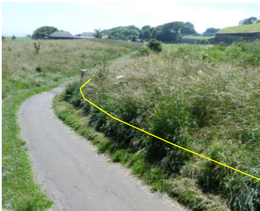
Plate F: Existing footpath. Located on figure 6. Looking south. Earthworks of north-east angle of Brass Bastion Counterscarp to right. Yellow line shows intended widening.
