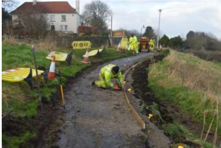
Plate 2: Fixing the wooden kerbing. Looking north towards Fields House.
