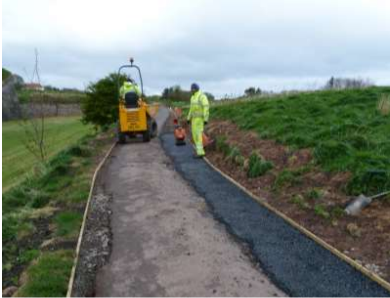
Plate 9: The same stretch of path as seen on plate 8 but looking north. Laying the first strip of tarmac.
