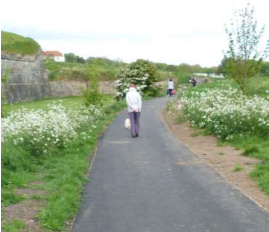
Plate 32: After works. Same as figure 31.
