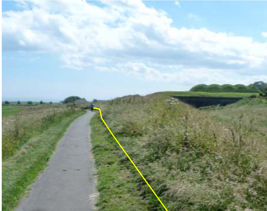
Plate E: Existing footpath. Located on figure 6. Looking south alongside Edwardian ditch (to right). Brass Bastion beyond. Yellow line shows intended widening.
