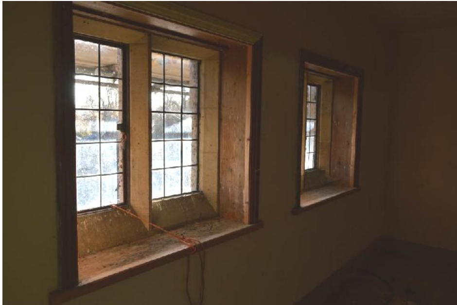
Plate 101: Gatehouse first floor. Windows looking south-west.
