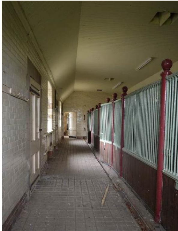
Plate 53: Eastern block of horse boxes in the north range. Looking west.
