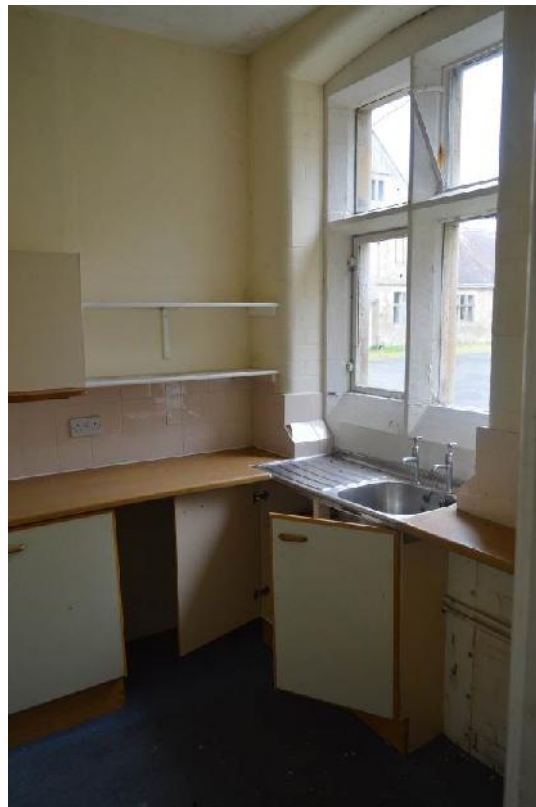
Plate 94: West domestic block. South kitchen. Looking north-east.
