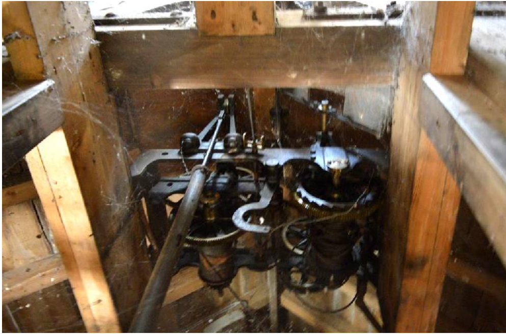
Plate 103: Mechanism of clock (looking up from first floor.
