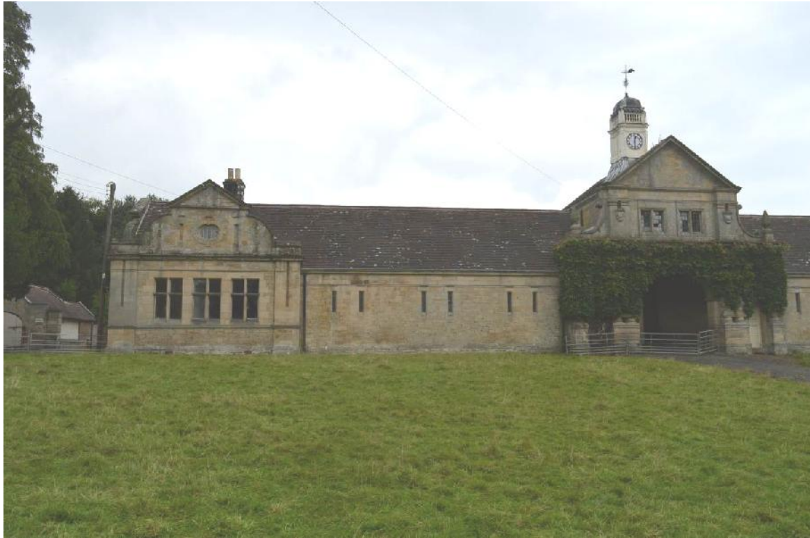
Plate 9: The western half of the south range of the building. Looking north.
