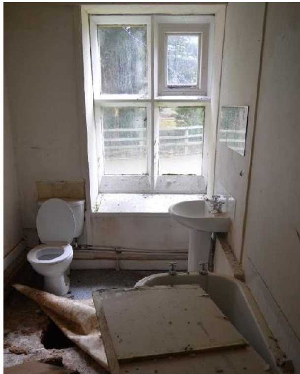
Plate 92: West domestic block. Bathroom. Looking west.
