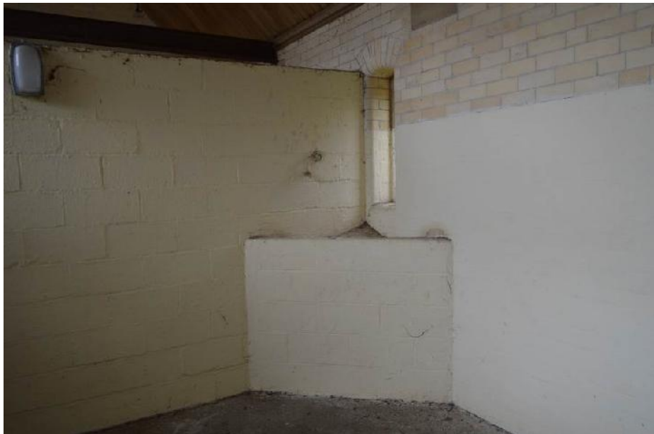
Plate 90: Interior of coach house 1 with trough in corner. Looking south-east.
