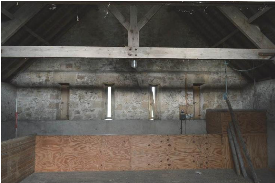
Plate 60: The fodder store. Looking north.
