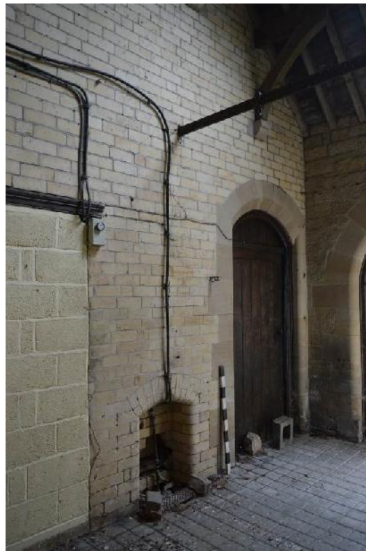
Plate 78: Horse wash. Looking west to arched door in south wall.
