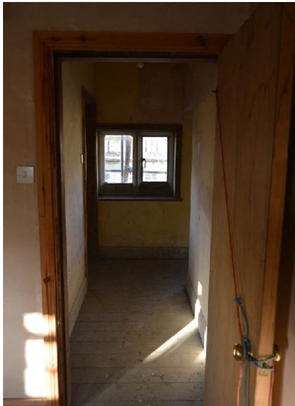
Plate 100: Gatehouse. First-floor corridor. Looking south.
