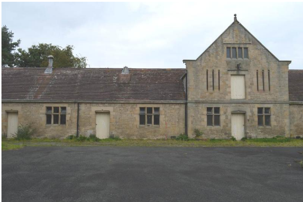
Plate 16: The courtyard. Looking north at the western part of the north range.
