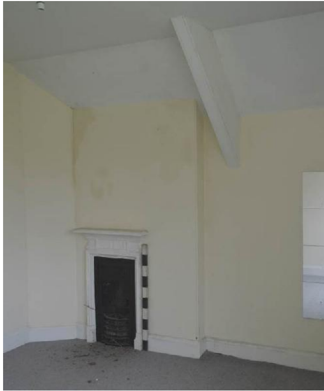
Plate 73: Fireplace in bedroom in east domestic block.
