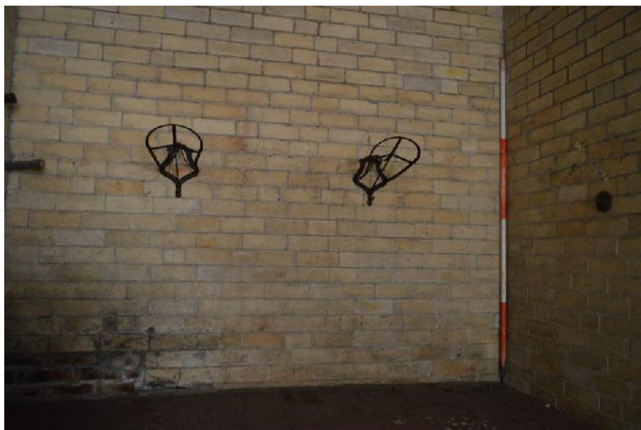
Plate 64: Tack room. Saddle supports in north wall. Looking north-east.
