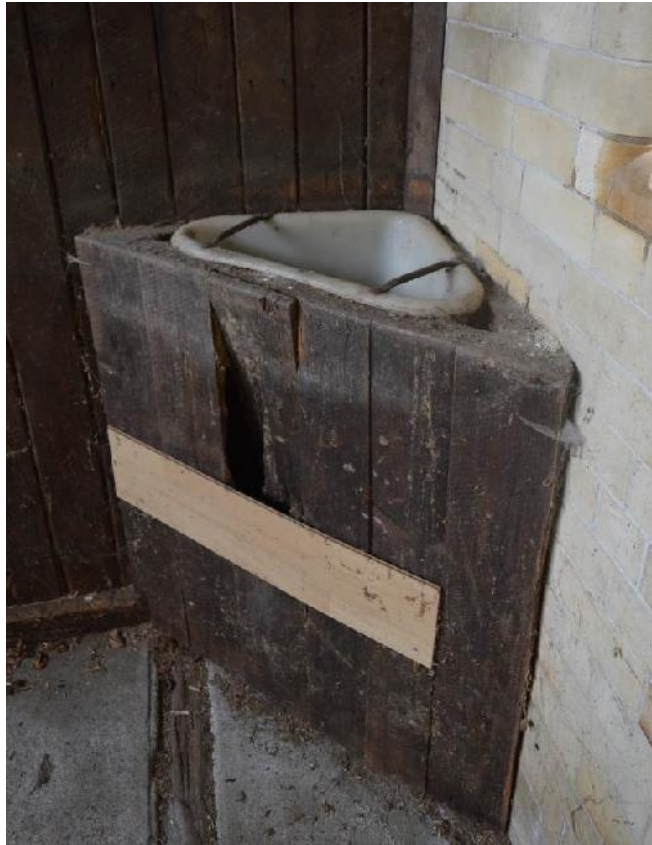
Plate 85: Trough in coach house 2. Looking south-east.
