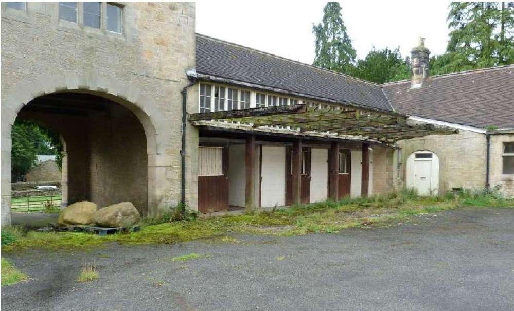
Plate 86: Coach house 1. External view from courtyard. Looking south-west
