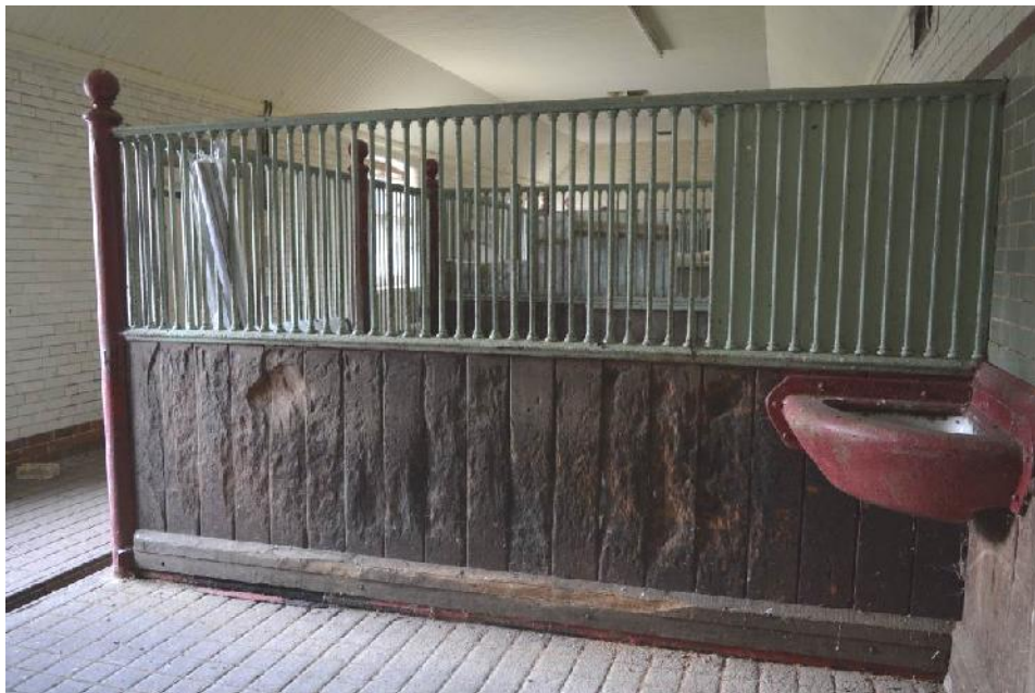
Plate 48: Partition screen in one of the horse boxes.
