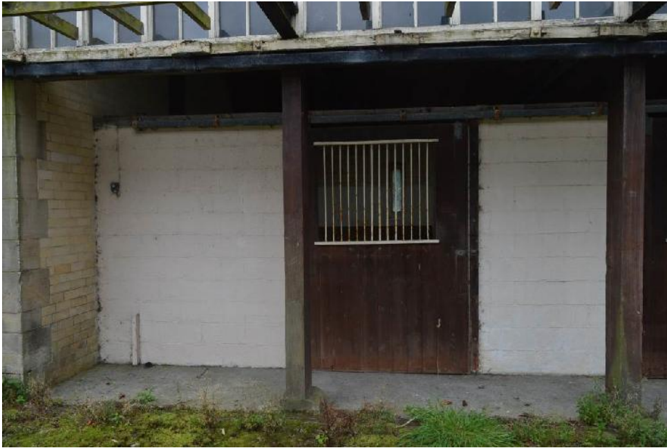
Plate 87: Entrance door with grille to coach house 1. Looking south.
