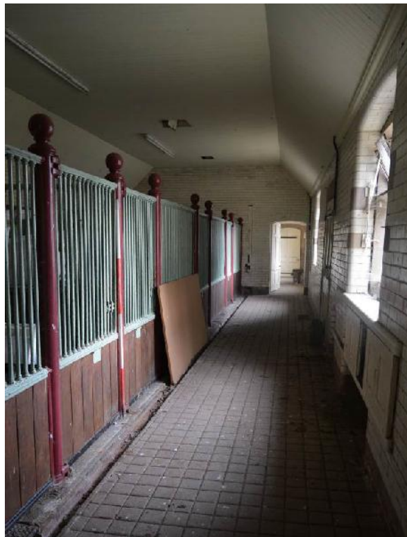
Plate 44: Horse boxes in the north range. West block looking east.
