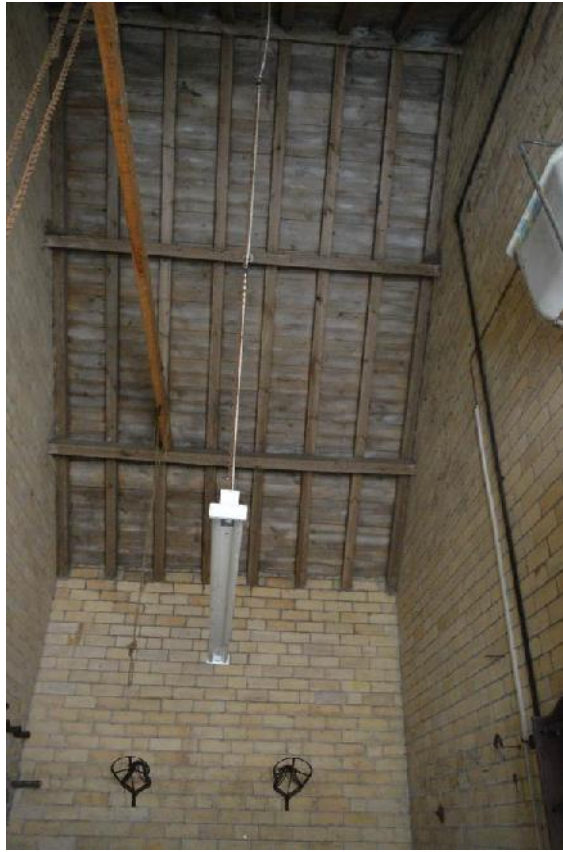
Plate 63: Tack room with supports for saddles. Looking north.
