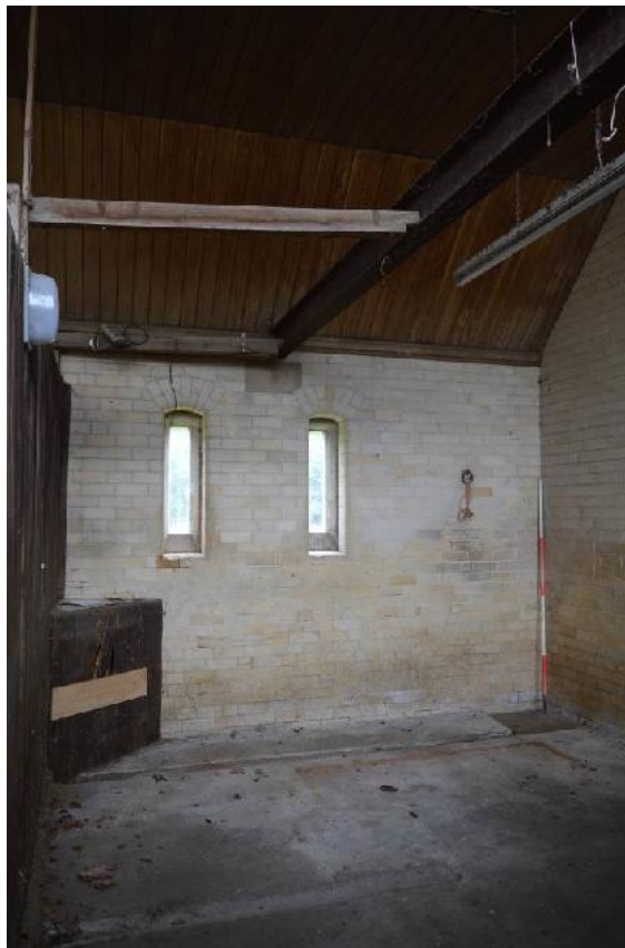
Plate 84: Interior of coach house 2. Looking south.
