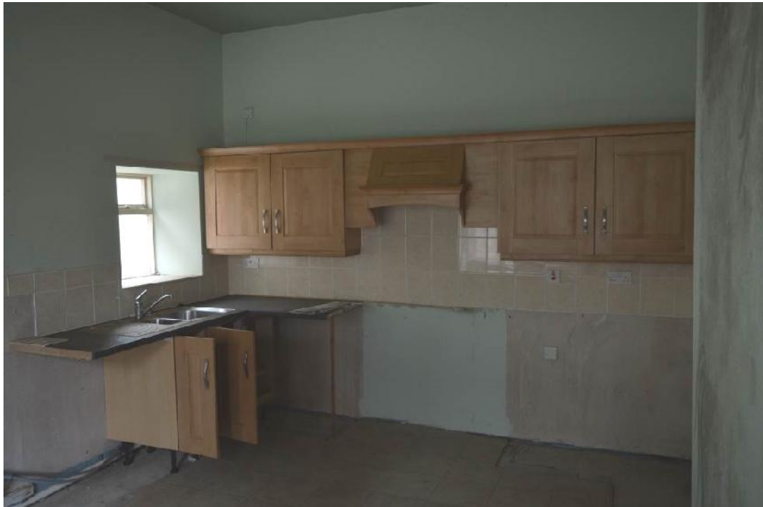
Plate 96: West domestic block. North kitchen. Looking east.
