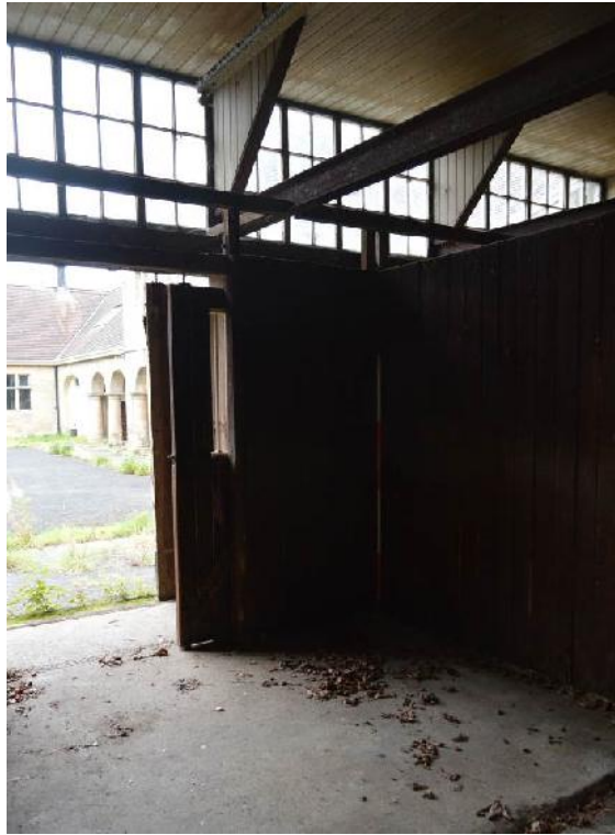
Plate 83: Interior of coach house 2. Looking north-east.
