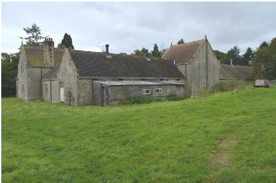
Plate 6: The north-east corner of the building. Looking south-west.
