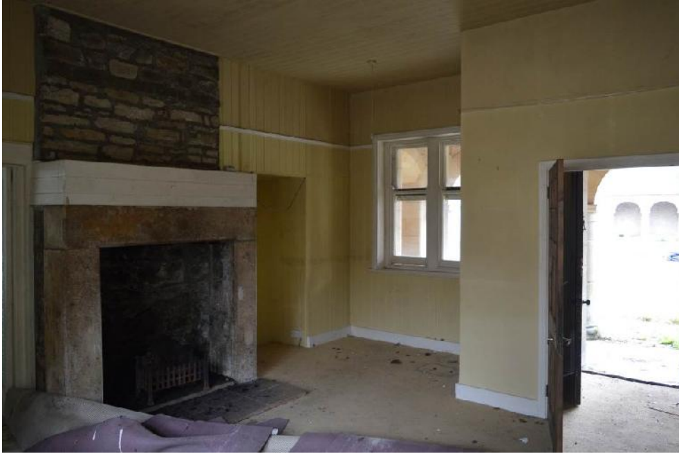
Plate 95: West domestic block. Living room in centre block. Looking east.
