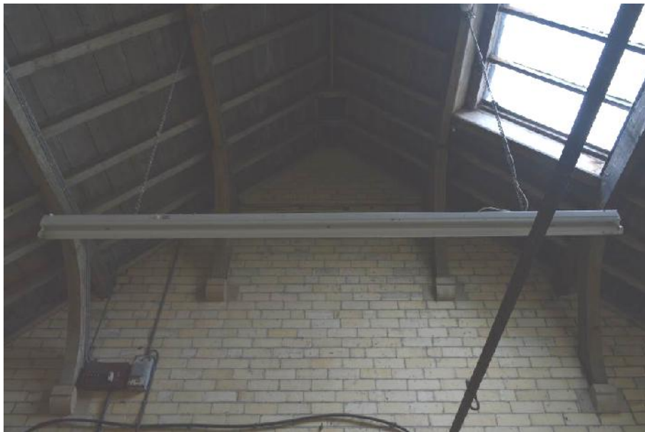
Plate 80: Horse wash. The roof structure. Looking south.
