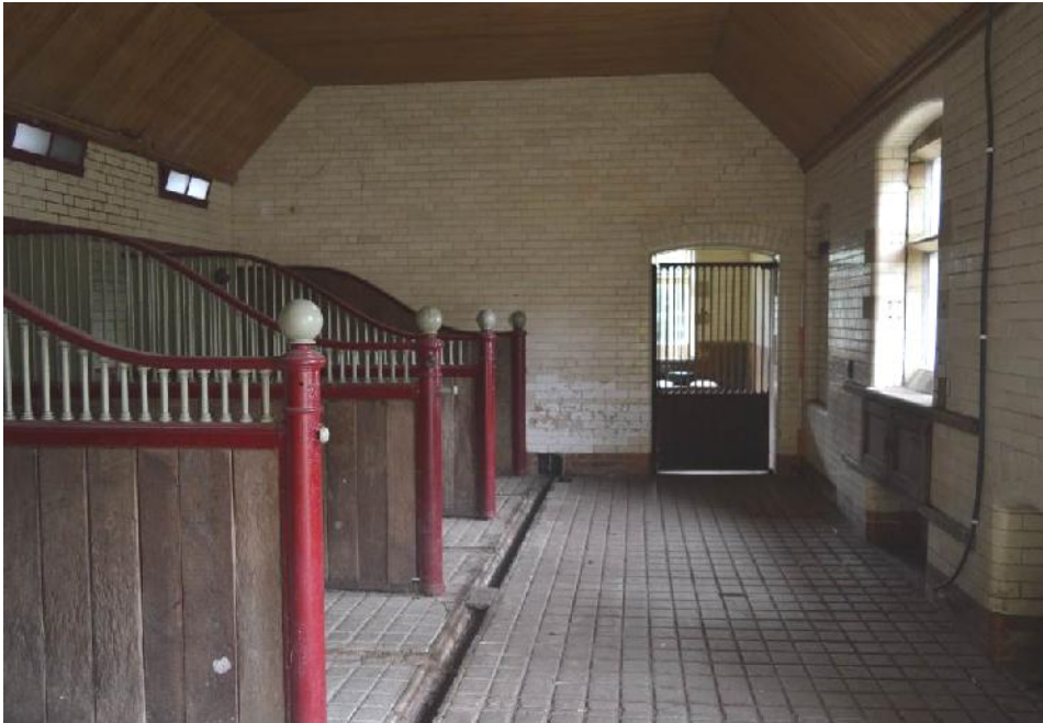
Plate 26: Looking south along the front of stalls in the mares' stables.
