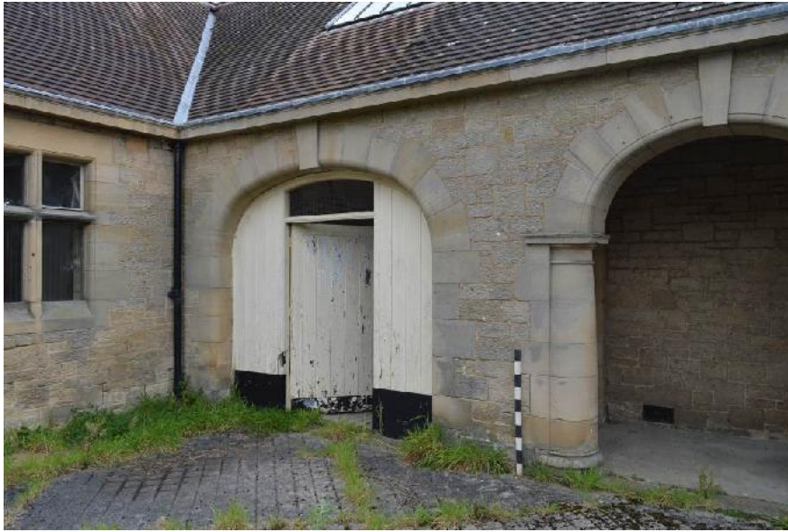
Plate 75: Entrance to horse wash from courtyard. Looking north-east.
