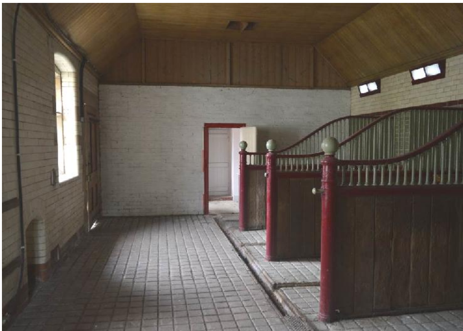
Plate 27: Looking north along the front of stalls in the mares' stables.
