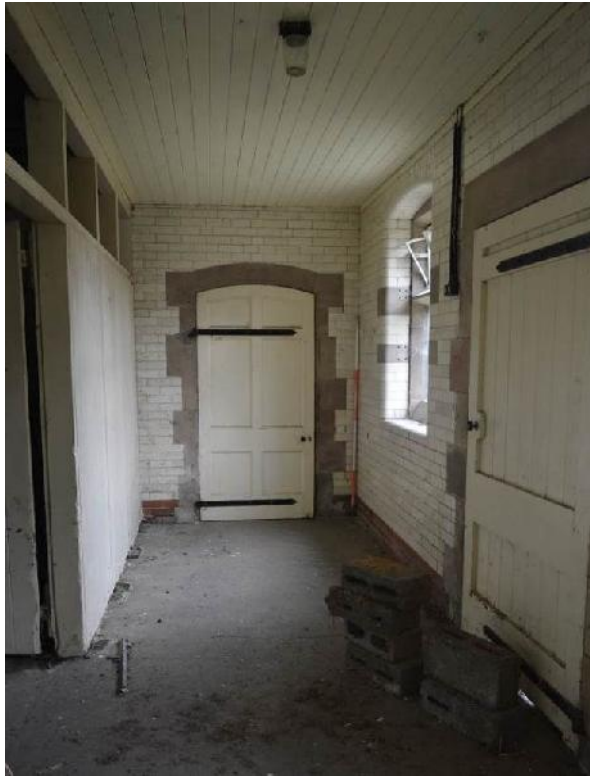
Plate 51: Passage south of the hay store. Looking east.
