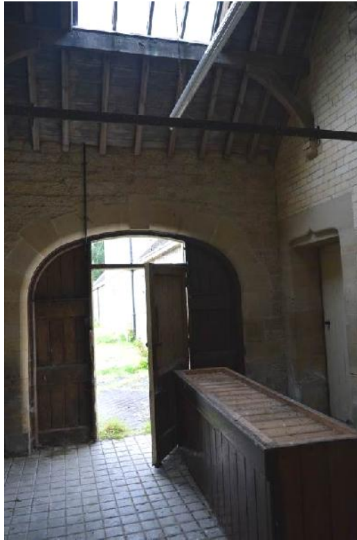
Plate 77: Horse wash. Looking west towards entrance.
