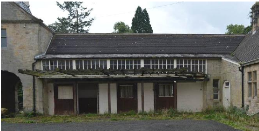
Plate 18: The courtyard. Looking south at the western part of the south range.
