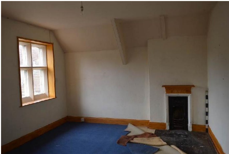
Plate 74: Fireplace in bedroom in east domestic block.
