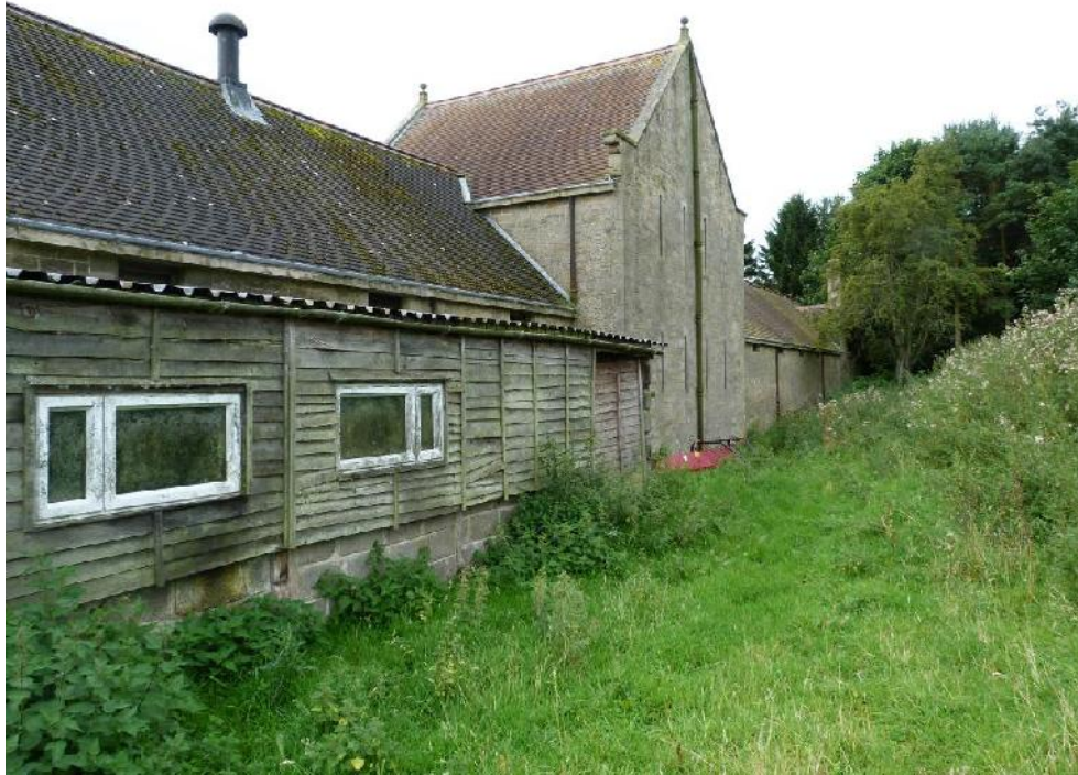
Plate 7: The north face of the building and timber offshot. Looking west.
