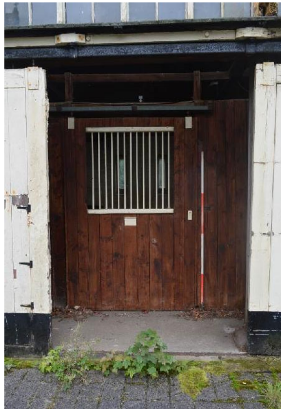
Plate 82: Entrance door with grille to coach house 2. Looking south.
