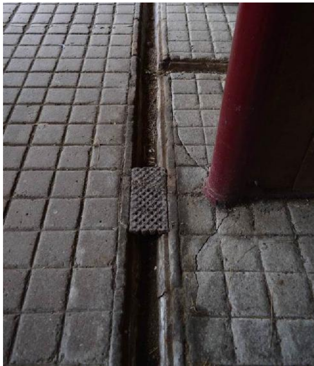
Plate 35: Drainage channel and non-slip concrete floor in the Mares' stables.
