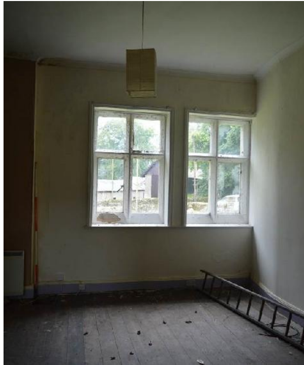
Plate 91: West domestic block. Looking south.
