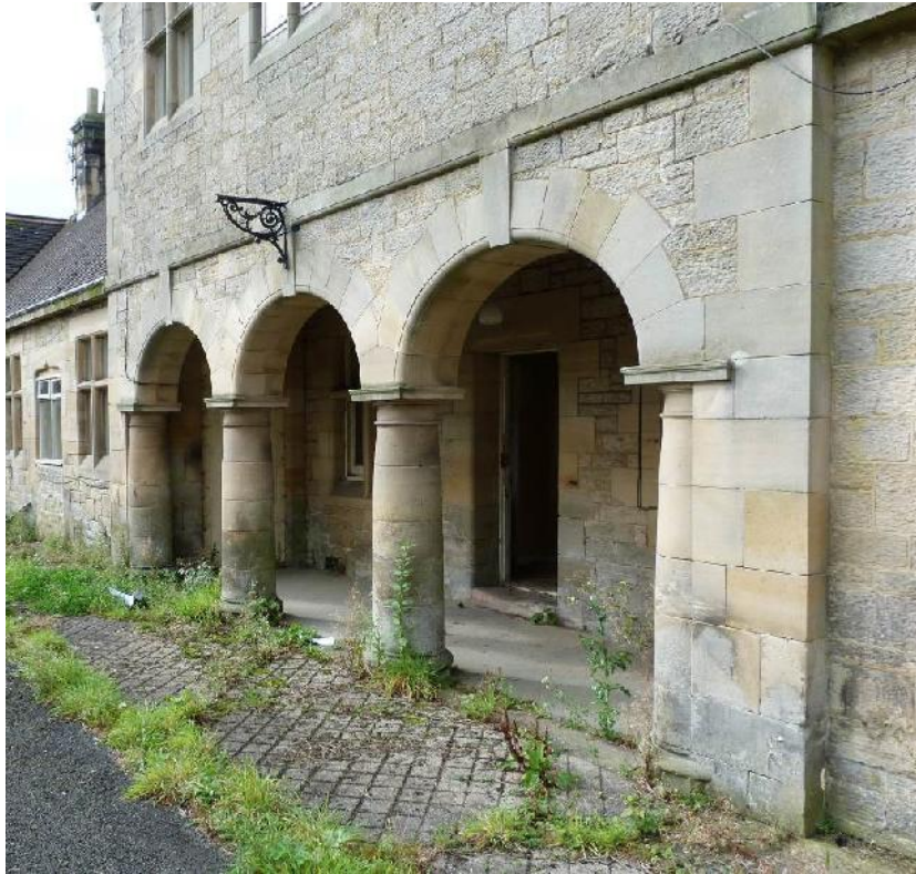
Plate 2: The east-facing frontage of the western accommodation block
