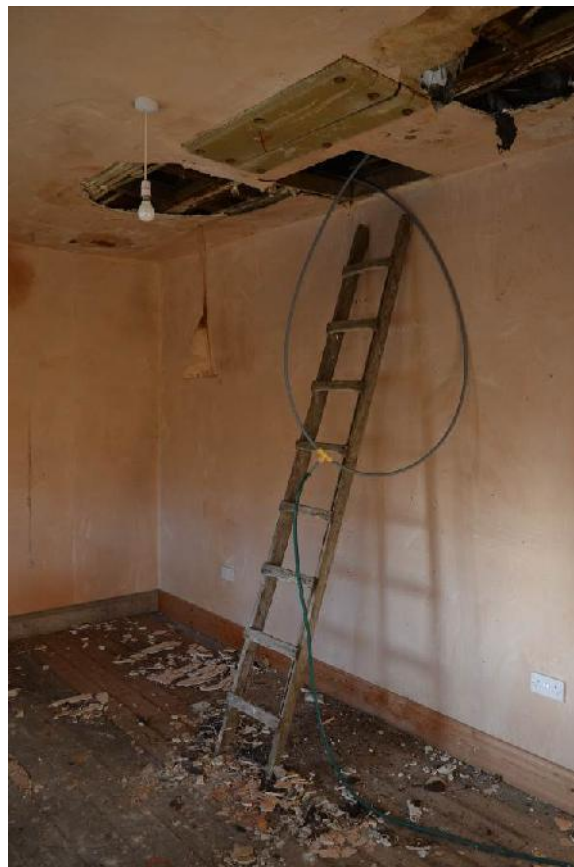
Plate 102: Gatehouse first floor. Entrance hatch to clock cupola.
