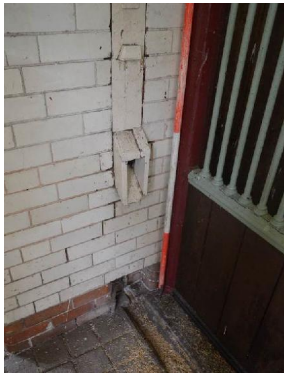
Plate 54: Feed chute in the west wall of the east block of stalls. There was an identical chute for the west block.
