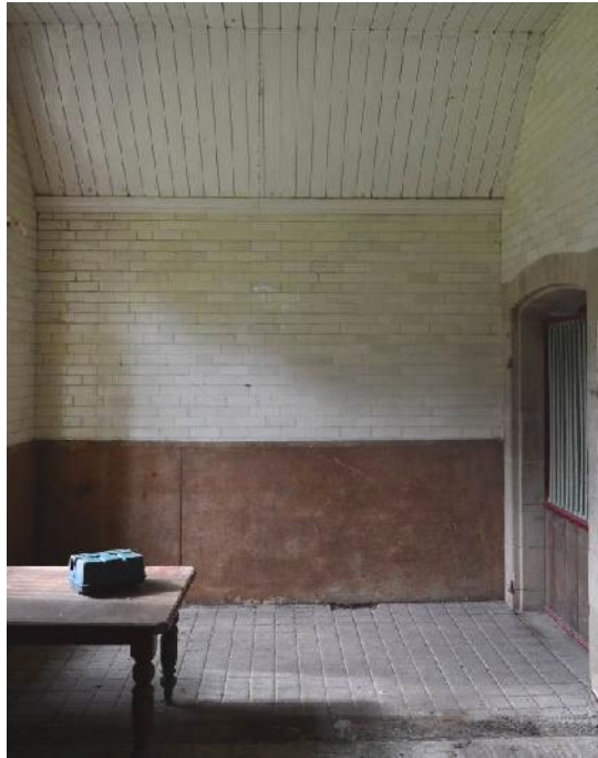
Plate 39: Looking north-west in the loose box.
