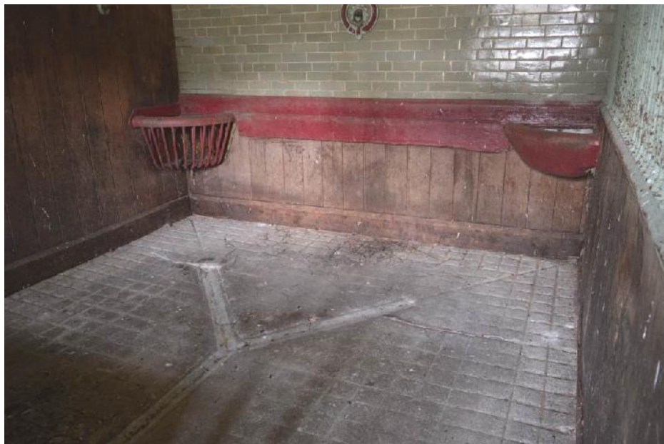
Plate 46: Inside one of the horse boxes. Non-slip concrete floor 'Y' drainage and manger and trough.
