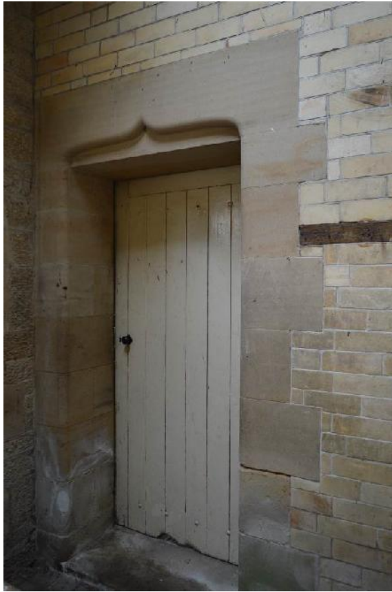
Plate 79: Horse wash. Door in north wall.
