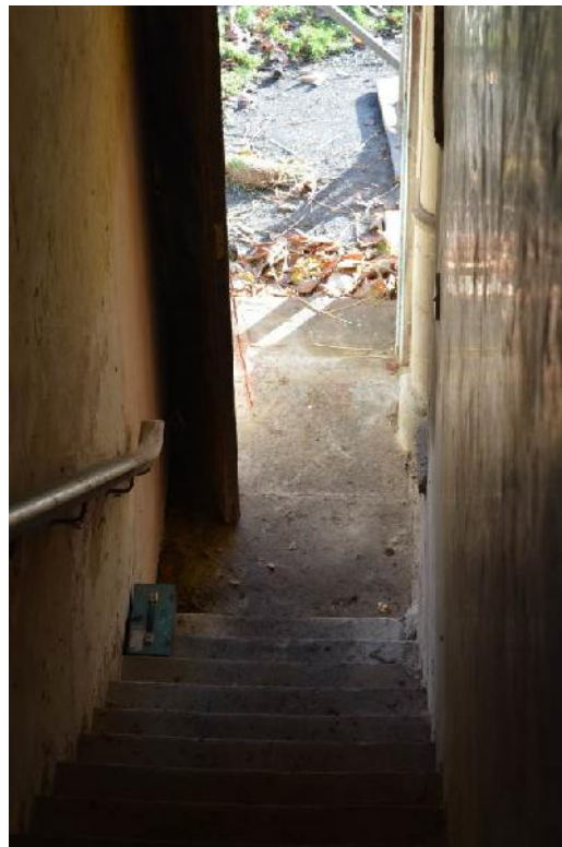
Plate 98: Gatehouse. Staircase down to ground.
