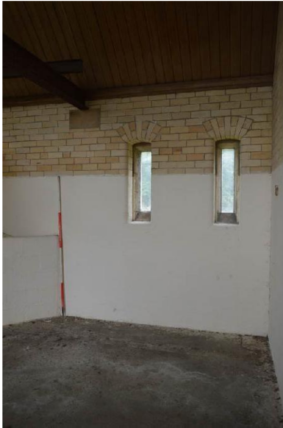
Plate 89: Interior of coach house 1. Looking south.
