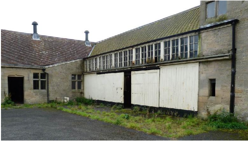
Plate 81: Coach house 2 from the courtyard. Looking south-east.
