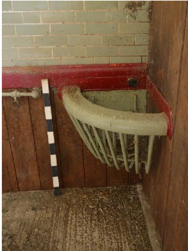
Plate 41: Manger in the loose box.
